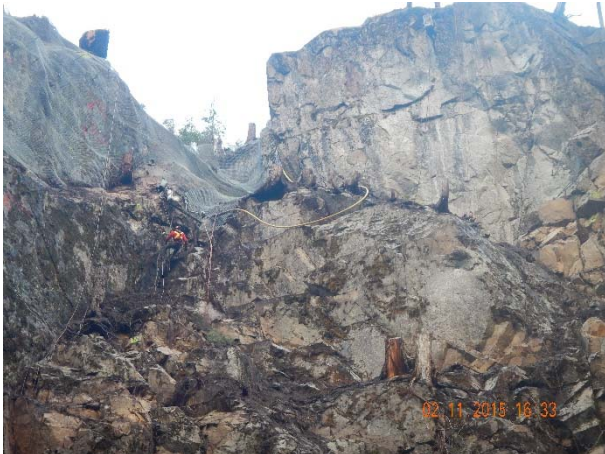
Photo 19 – Rock consolidation above intake access road (November 2, 2015).
