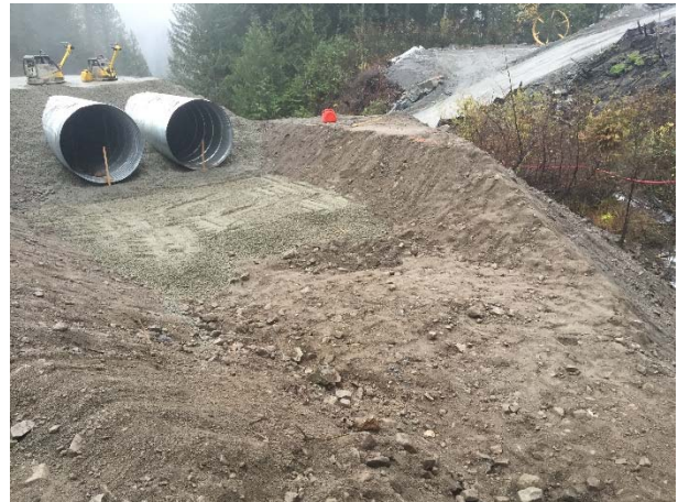
Photo 15 – ASTR03 over-drain construction (November 6, 2015).
