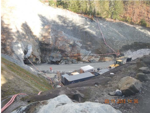
Photo 10 – Current conditions at the ULRHEF downstream tunnel portal (November 3, 2015).
