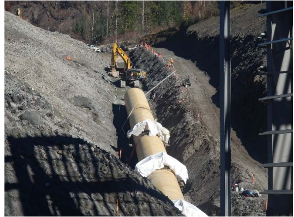
Photo 13 – Penstock installation, welding, and coating (November 5, 2015).
