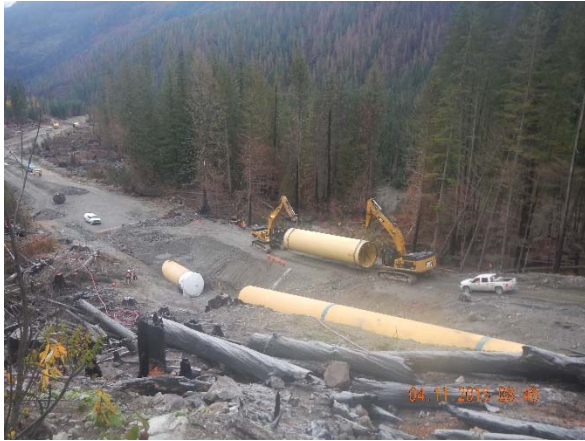
Photo 12 – Transporting and placing penstock (November 4, 2015).
