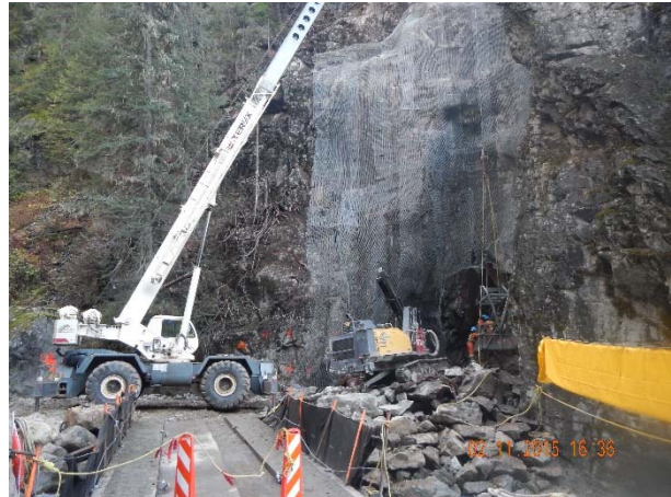
Photo 20 – Rock consolidation above diversion tunnel (November 2, 2015).
