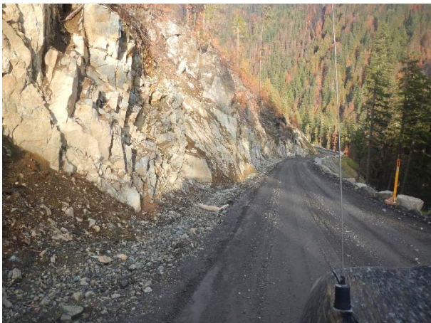
Photo 23 – Ditch maintenance and installation of Curlex within the ditch line (November 5, 2015).
