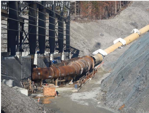
Photo 17 – Current conditions at the ULRHEF powerhouse (November 5, 2015).
