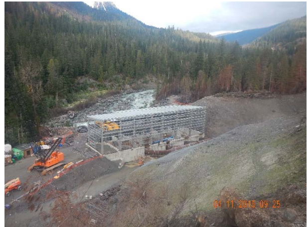
Photo 18 – ULRHEF powerhouse superstructure construction (November 4, 2015).
