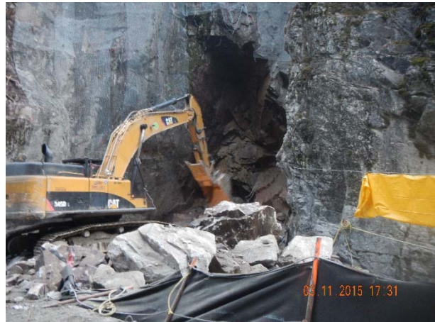
Photo 22 – Mucking after diversion tunnel blast (November 3, 2015).
