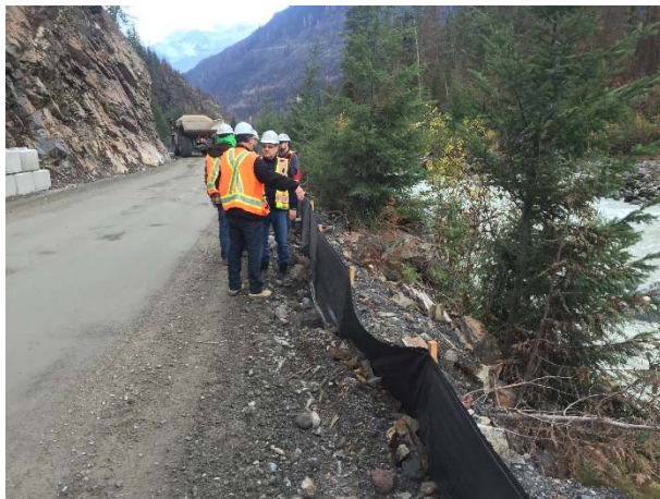
Photo 1 – Kick-off meeting held at KM 41.1 prior to road repairs (October 26, 2015).
