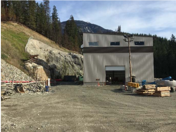
Photo 29 – BDRHEF tunnel portal and powerhouse structure (October 27, 2015).
