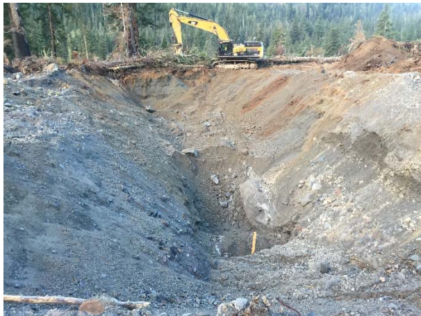
Photo 18 – Excavation for Drain #5 (October 28, 2015).
