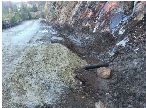
Photo 2 – Culvert installed at KM 41.1 on the Lillooet River FSR (October 27, 2015).
