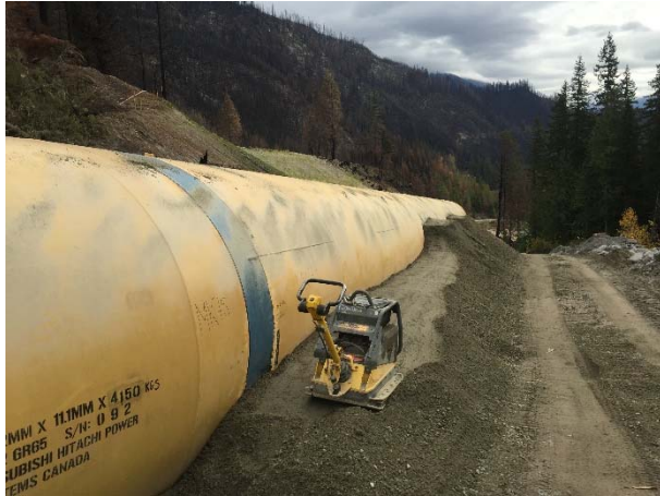
Photo 16 – Penstock backfill works near 2+850 (October 26, 2015).
