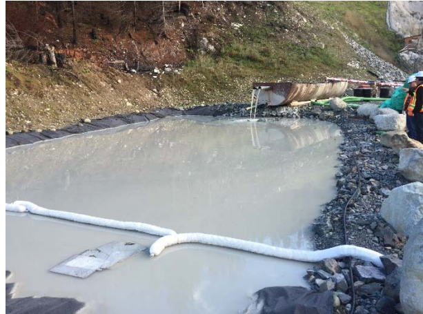
Photo 30 – BDRHEF tunnel portal settling ponds (October 27, 2015).
