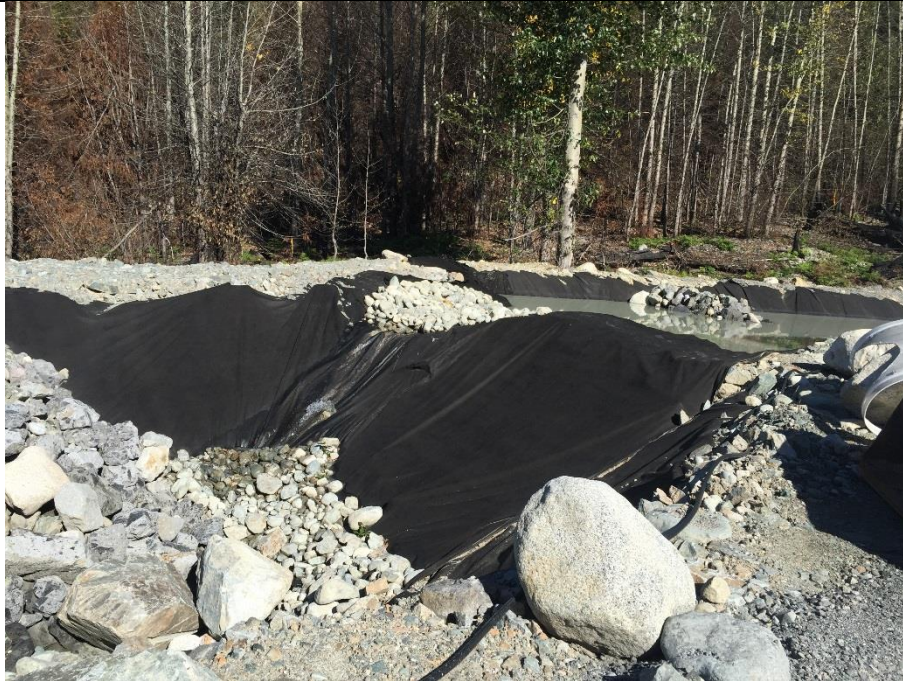
BDR#25. Water from the fourth cell of the water treatment ponds is seeping out of the edge of the pond, flows over an active haul path, and along the edge of the powerhouse access road before infiltrating to ground
