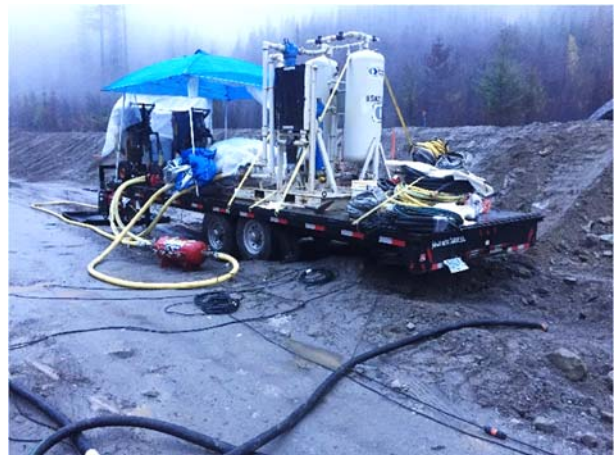
Photo 19 – Penstock lining equipment at 3+500 on the penstock alignment (October 29, 2015).
