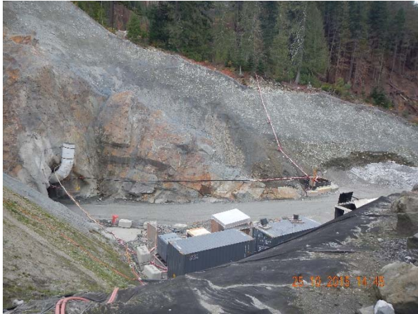
Photo 13 – Current conditions at the ULRHEF downstream tunnel portal (October 25, 2015).
