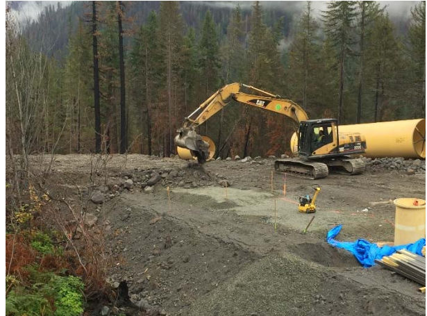
Photo 17 – Penstock backfill near 3+200 (October 28, 2015).
