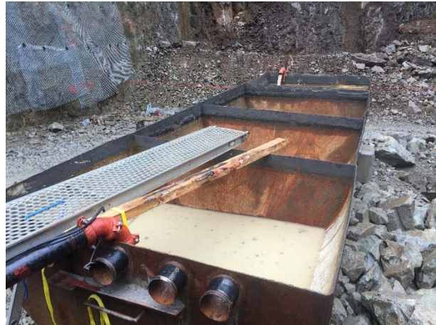
Photo 28 – Tunneling wastewater pumped to active water treatment system (October 29, 2015).
