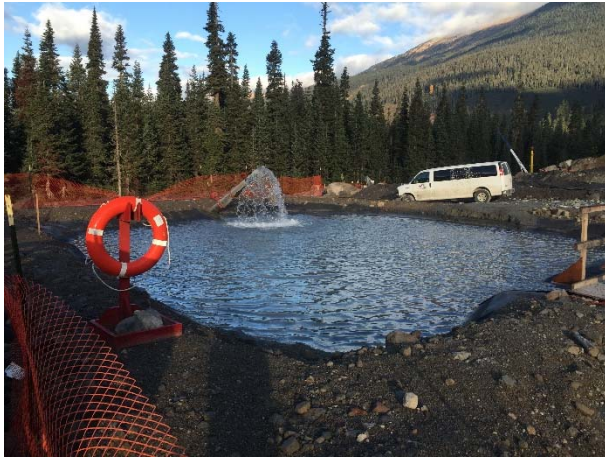
Photo 9 – First cell of ULRHEF intake sediment basins (October 26, 2015).
