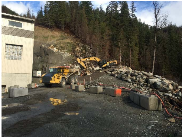
Photo 31 – Modification works on BDRHEF powerhouse debris flood protection berm (October 30, 2015).
