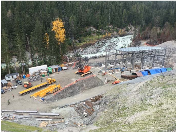
Photo 20 – Current conditions at the ULRHEF powerhouse (October 26, 2015).
