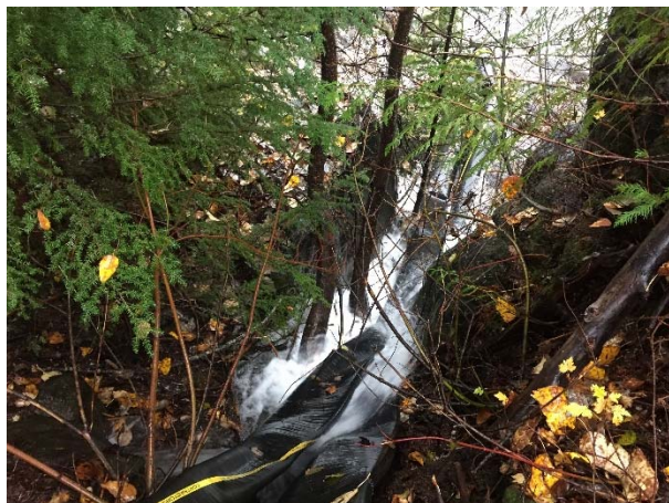
Photo 22 – Dewatering seepage water from the ULRHEF powerhouse sump to the Lillooet River (October 31, 2015).
