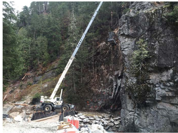
Photo 24 – Rock consolidation above diversion tunnel (October 26, 2015).
