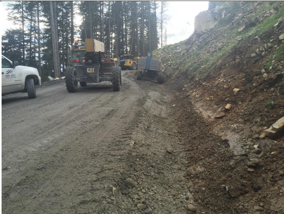
BDR#25. Water from the fourth cell of the water treatment ponds is seeping out of the edge of the pond, flows over an active haul path, and along the edge of the powerhouse access road before infiltrating to ground
