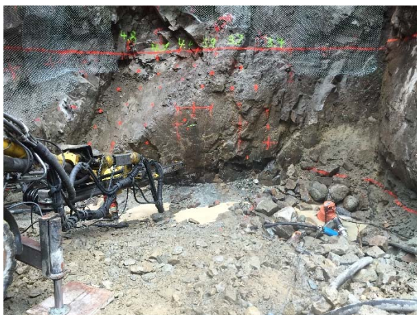
Photo 25 – Drilling for diversion tunnel blast (October 29, 2015).
