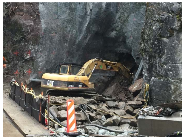
Photo 26 – Mucking after diversion tunnel blast (October 29, 2015).
