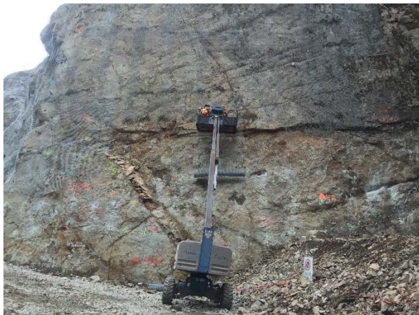
Photo 23 – Rock consolidation above intake access road (October 26, 2015).
