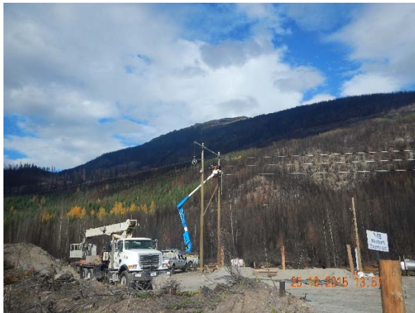
Photo 32 – Post-wildfire rebuild works in Segment 1 (October 25, 2015).
