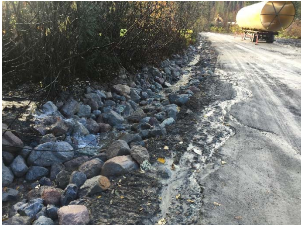
Photo 5 – Armoured ditch installed at KM 42.5 on the Lillooet River FSR (October 30, 2015).
