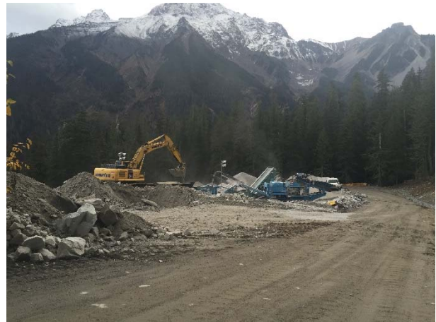
Photo 2 – Conditions at the KM 45 crusher pad that has been installed on top of the rock spoil pile (October 22, 2015).
