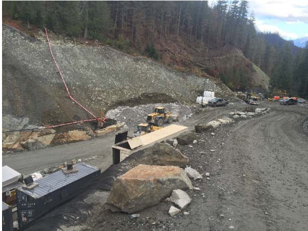
Photo 7 – Current conditions at the ULRHEF downstream tunnel portal laydown (October 22, 2015).
