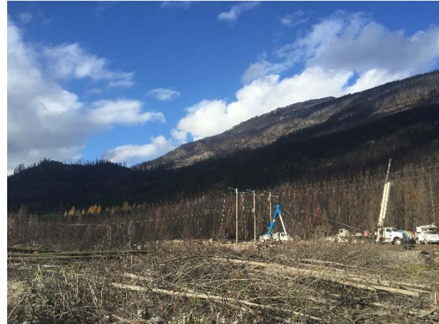
Photo 23 – Post wildfire repair works in Segment 1 (October 22, 2015).
