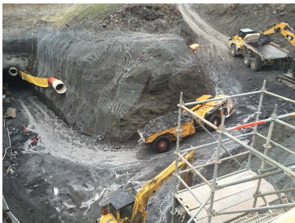
Photo 5 – Blast rock mucking at the ULRHEF upstream tunnel portal (October 21, 2015).
