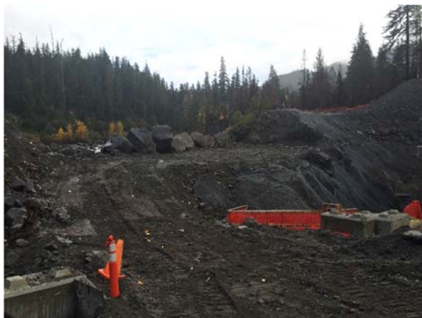
Photo 11 – Excavation of the top of the flood protection berm (October 21, 2015).
