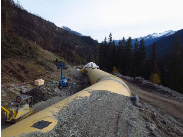
Photo 9 – Penstock backfill works near 2+900 (October 24, 2015).
