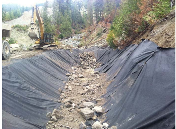
Photo 8 – Maintenance of the ULRHEF downstream tunnel portal infiltration ponds (October 19, 2015).
