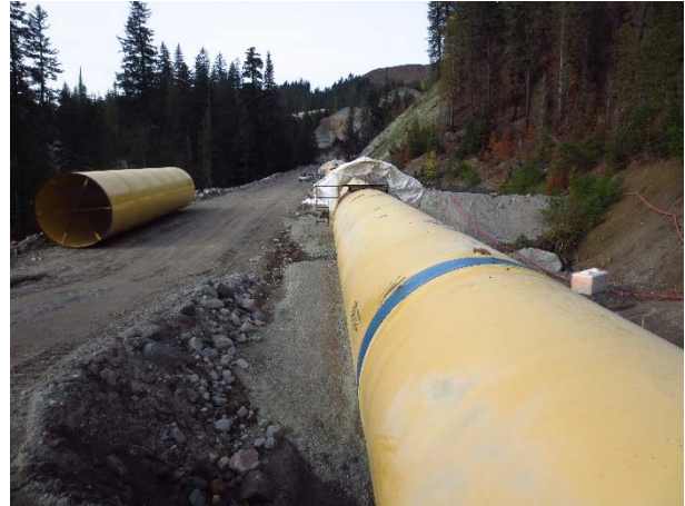
Photo 10 – Penstock welding near 2+900 (October 24, 2015).
