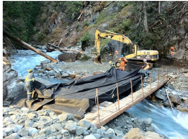
Photo 16 – Upstream diversion tunnel portal access bridge installation at BDRHEF intake (October 23, 2015).
