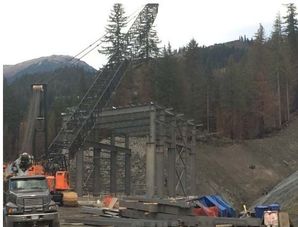
Photo 12 – ULRHEF powerhouse superstructure installation (October 22, 2015).
