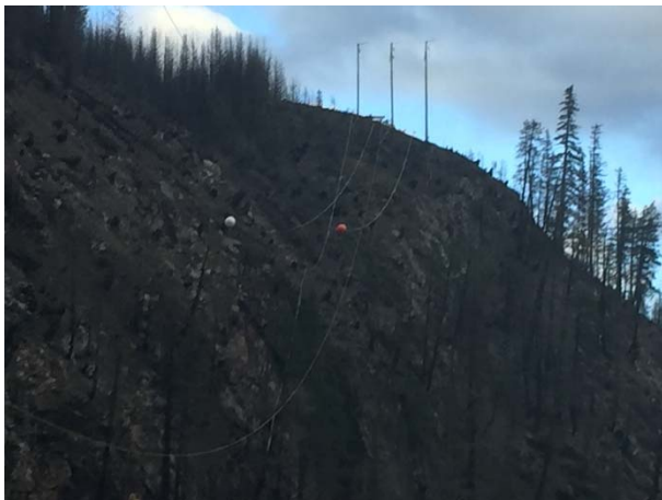
Photo 24 – Aeronautical markers being installed in Segment 1 between structures 4 – 5. (October 22, 2015)
