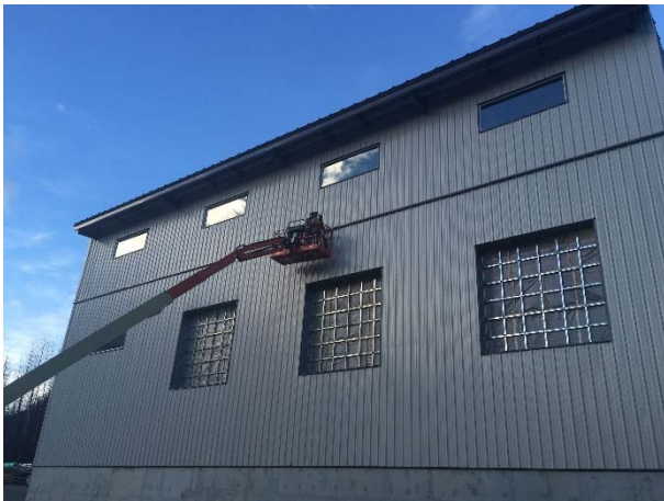
Photo 19 – BDRHEF powerhouse structure works (October 20, 2015).
