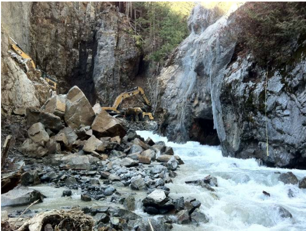
Photo 15 – Instream excavation at the BDRHEF intake (October 20, 2015).
