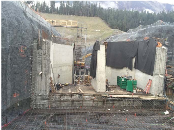
Photo 3 – Rebar and form work at the ULRHEF intake (October 21, 2015).
