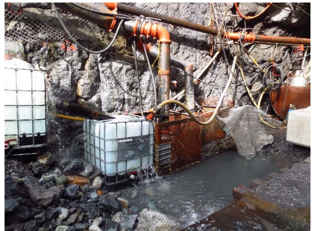
Photo 8 – ULRHEF upstream tunnel portal sump (October 5, 2015).
