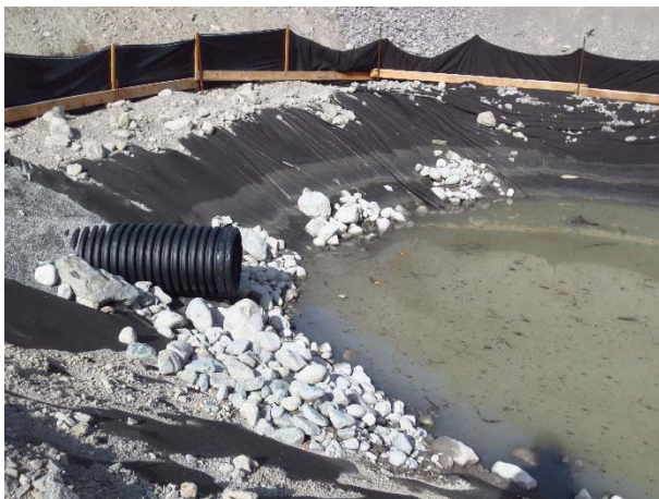
Photo 9 – ULRHEF intake sediment basin outlet pipe (October 5, 2015).
