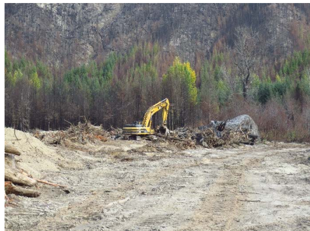
Photo 2 – Stripping and grubbing of the PAG rock storage area (October 6, 2015).
