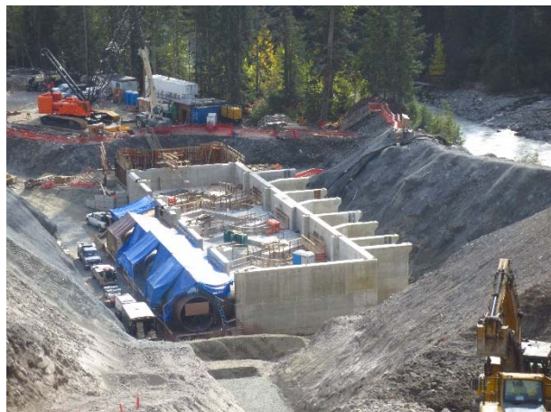
Photo 15 – Current conditions at the ULRHEF powerhouse (October 6, 2015).
