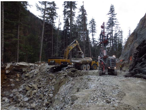
Photo 17 – Excavation for access ramp at BDRHEF intake (October 6, 2015).
