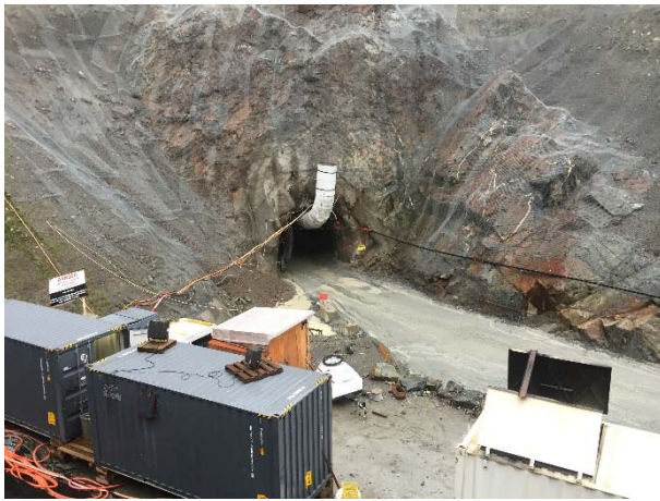
Photo 10 – Current conditions at the ULRHEF downstream tunnel portal (October 8, 2015).
