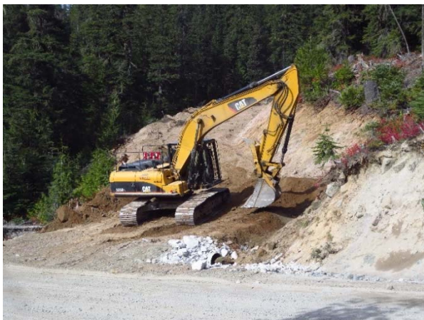
Photo 1 – Ditching access road to KM 45 spoil pile (October 5, 2015).
