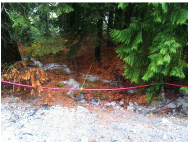
Photo 12 – ULRHEF downstream tunnel portal infiltration pond seepage (October 10, 2015).
