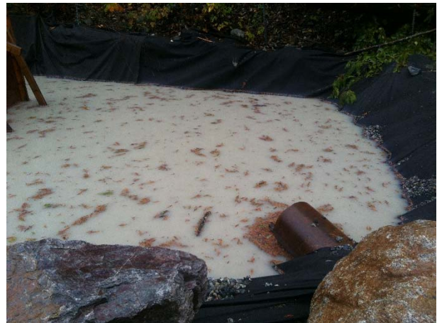
Photo 11 – ULRHEF downstream tunnel portal infiltration ponds (October 10, 2015).
