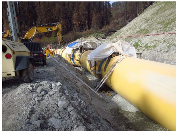
Photo 14 – Penstock welding near 3+500 (October 5, 2015).
