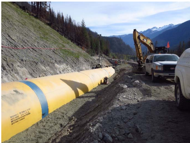
Photo 13 – Penstock backfill works (October 5, 2015).
