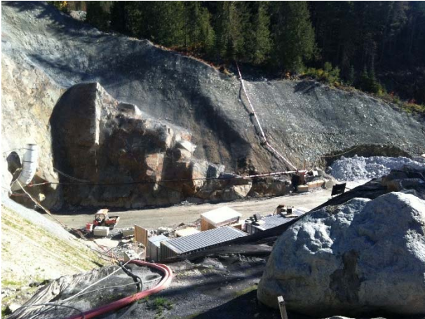
Photo 3 – Current conditions at the ULRHEF downstream tunnel portal (October 3, 2015).
