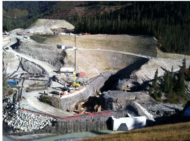
Photo 2 – Overview of the ULRHEF intake works area (October 3, 2015).
