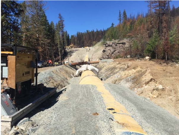
Photo 6 – Penstock backfill works near ASTR-04 (September 29, 2015).
