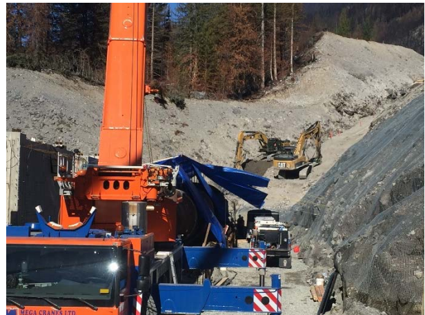
Photo 9 – Installation of the manifold continued during this reporting period (September 29, 2015).
