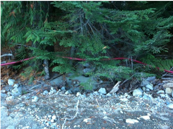
Photo 5 – ULRHEF downstream tunnel portal infiltration pond seepage (October 3, 2015).
