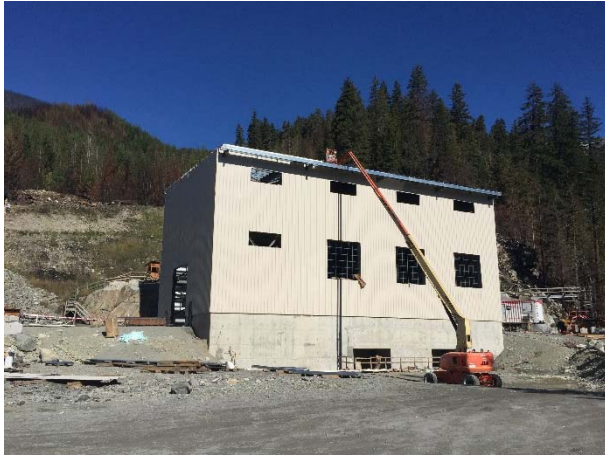
Photo 12 – BDRHEF powerhouse structure (September 29, 2015).
