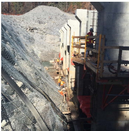
Photo 8 – Current conditions at the tailrace of the ULRHEF powerhouse (September 29, 2015).
