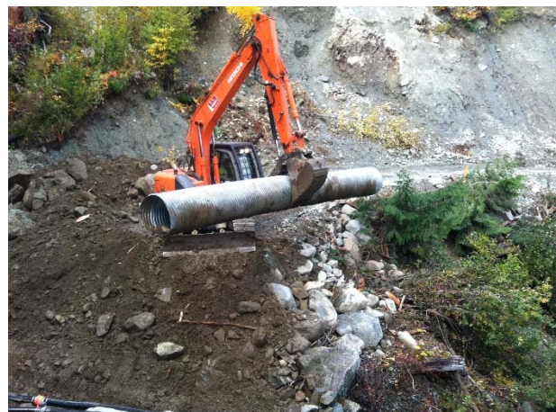
Photo 17 – Removal of stream 272a culvert completed in the dry. (October 2, 2015).
