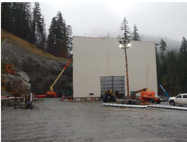
Photo 22 – BDRHEF downstream portal entrance and powerhouse structure (September 24, 2015).
