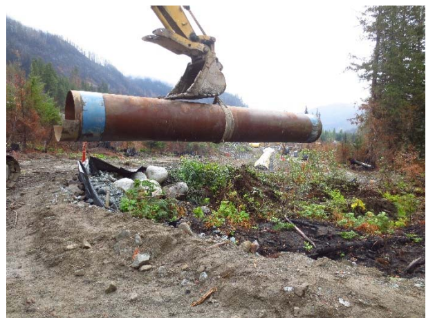
Photo 14 – Culvert extension installation at ASTR04 penstock crossing (September 16, 2015).
