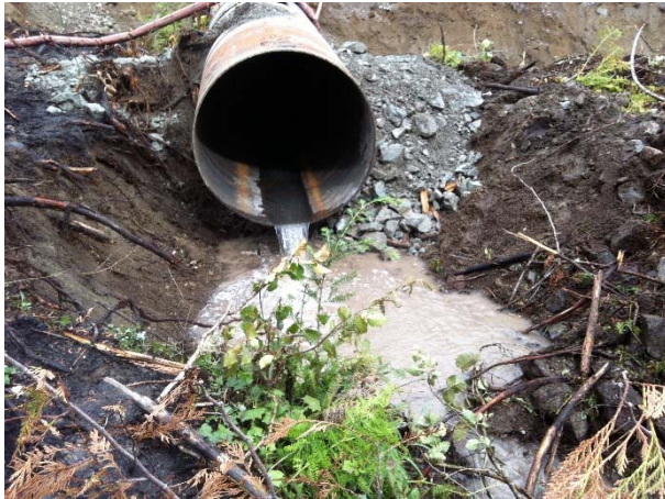
Photo 15 – Culvert extension installation at ASTR04 penstock crossing (September 17, 2015).
