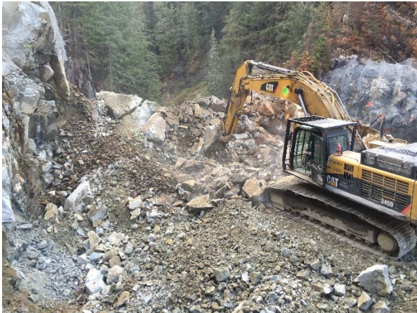
Photo 20 – Excavation for access ramp at BDRHEF intake (September 26, 2015).
