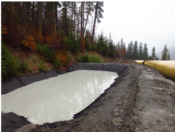
Photo 10 – New settling ponds at 2+750 on the penstock alignment (September 19, 2015).
