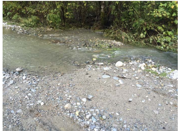
Photo 25 – Water flowing across South Lillooet FSR in Segment 6 (September 25, 2015).
