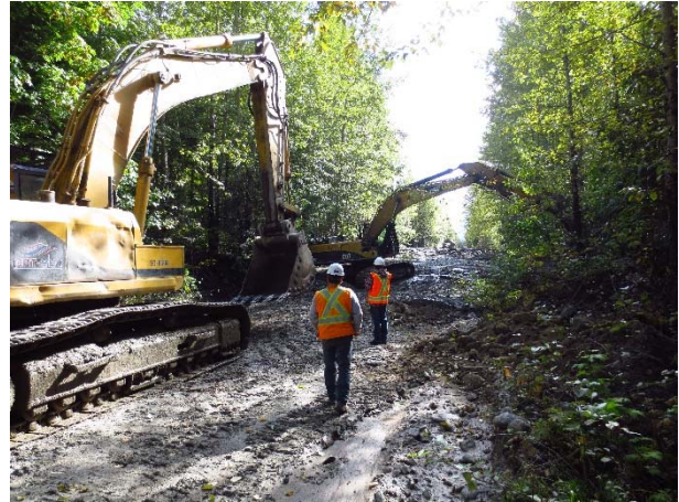
Photo 2 – Road maintenance works at 32 KM to repair debris slide damage (September 21, 2015).
