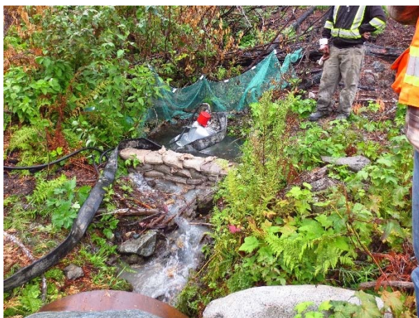
Photo 13 – Sandbag berm and pump used to isolate work area from flowing water at ASTR04 (September 16, 2015).
