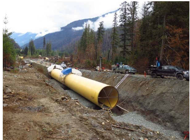
Photo 12 – Penstock welding near 3+500 (September 23, 2015).
