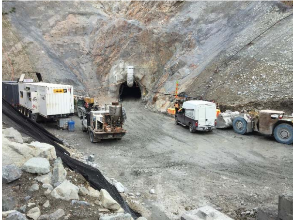
Photo 8 – Current conditions at the ULRHEF downstream tunnel portal (September 20, 2015).
