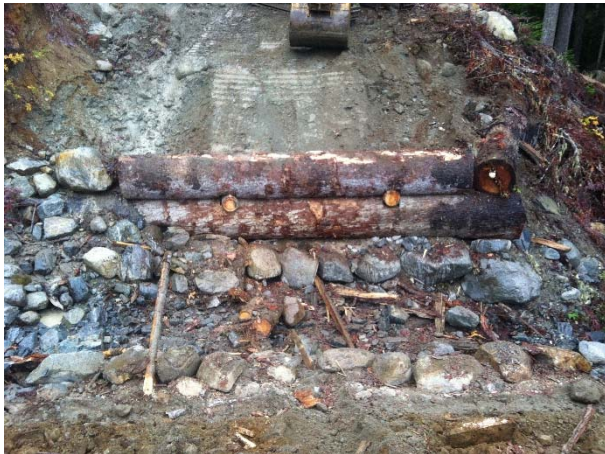
Photo 24 – Bridge removal at Stream 347A in Segment 14 (September 18, 2015).
