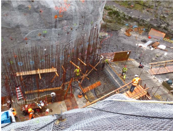
Photo 4 – Rebar and formwork installation at the ULRHEF intake (September 19, 2015).
