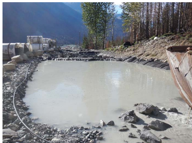
Photo 23 – BDRHEF downstream portal settling ponds (September 21, 2015).
