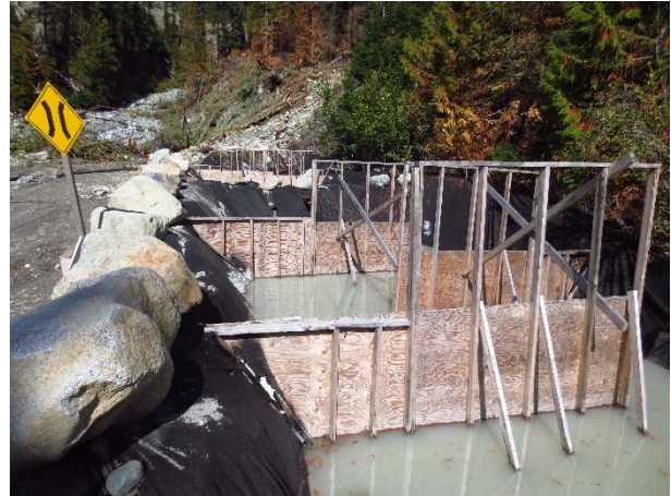
Photo 9 – ULRHEF downstream tunnel portal infiltration ponds (September 21, 2015).
