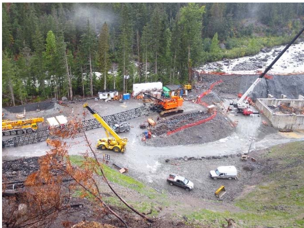
Photo 16 – Current conditions at the ULRHEF powerhouse (September 23, 2015).
