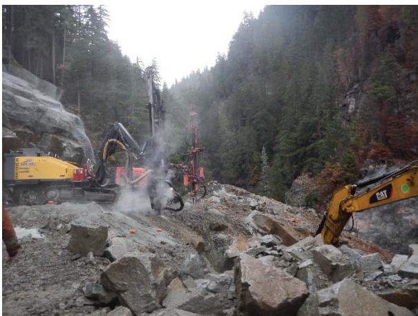
Photo 18 – Drilling and excavation for access ramp at BDRHEF intake (September 24, 2015).
