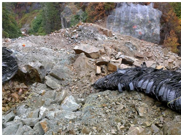
Photo 19 – Conditions following blast for access ramp at BDRHEF intake (September 24, 2015).
