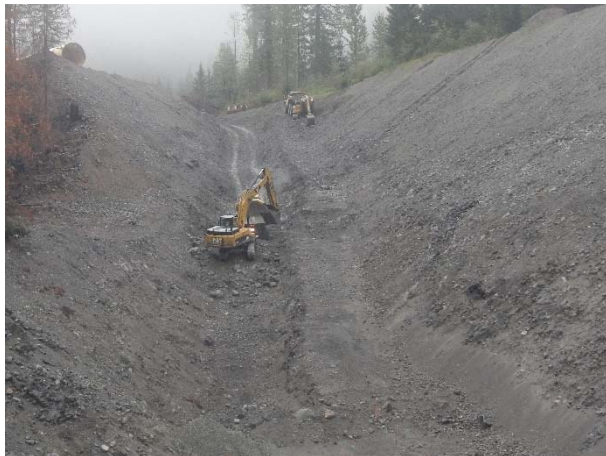
Photo 11 – Penstock excavation near 4+000 (September 24, 2015).
