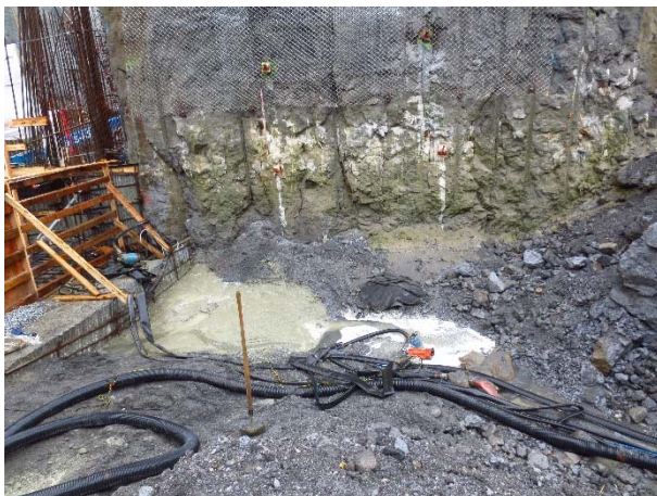
Photo 6 – Intake sump collecting seepage and runoff from worksite (September 23, 2015).
