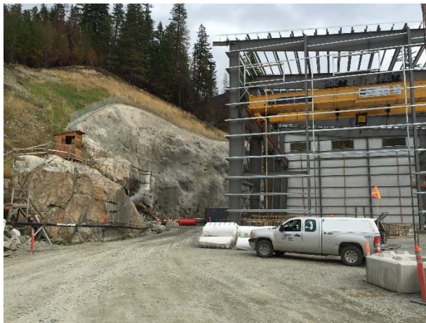
Photo 22 – BDRHEF downstream portal entrance and powerhouse structure (September 7, 2015).
