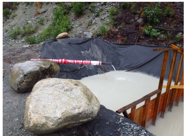
Photo 12 – ULRHEF downstream tunnel portal infiltration ponds (September 7, 2015).
