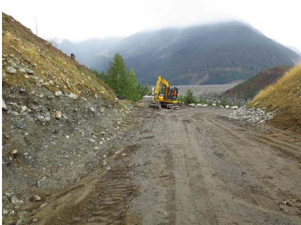
Photo 1 – Maintenance work on camp access road (September 2, 2015).
