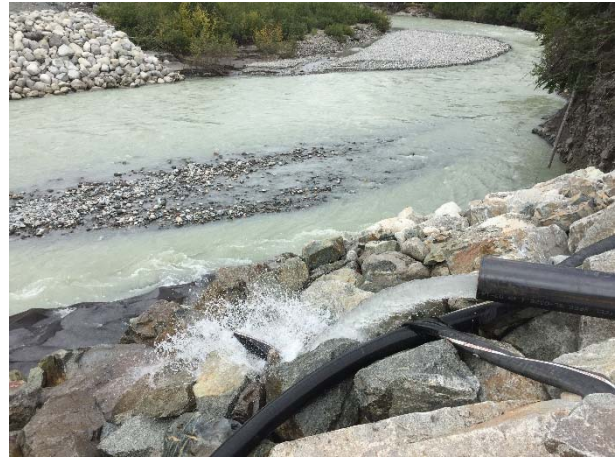
Photo 10 – Dewatering intake work area to Lillooet River (September 12, 2015).
