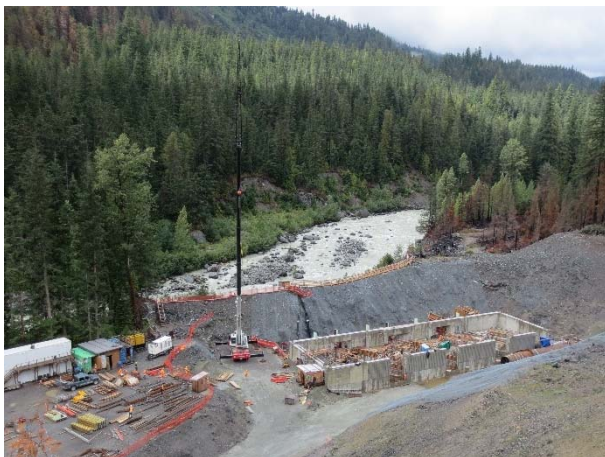
Photo 16 – Current conditions at the ULRHEF powerhouse (September 2, 2015).
