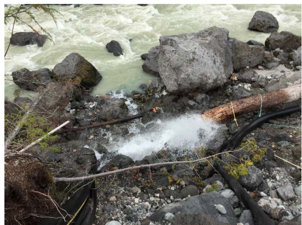
Photo 19 – Dewatering powerhouse sump to Lillooet River (September 7, 2015).
