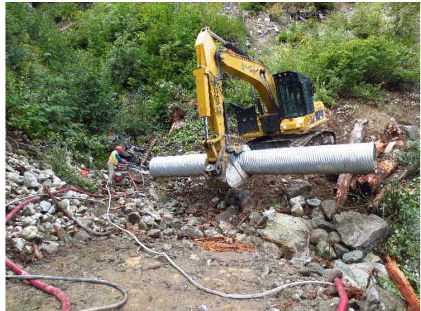
Photo 25 – Culvert installation with isolation in place at Stream 272A (September 4, 2015).
