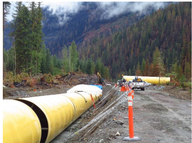
Photo 14 – Penstock welding at 3+750 (September 2, 2015).
