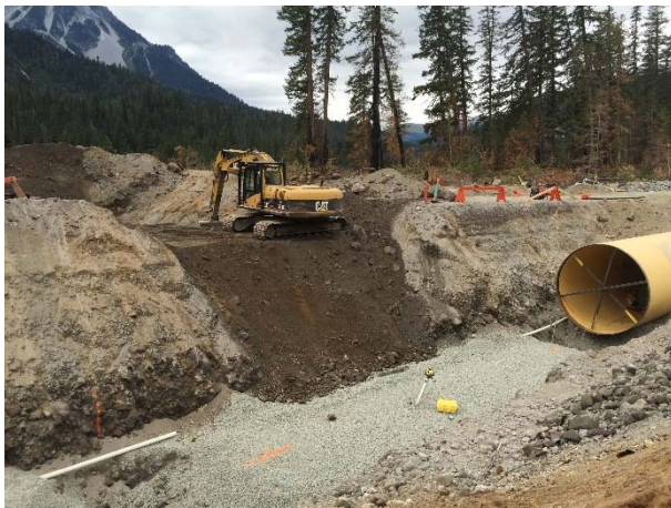
Photo 13 – Penstock backfill works (September 7, 2015).
