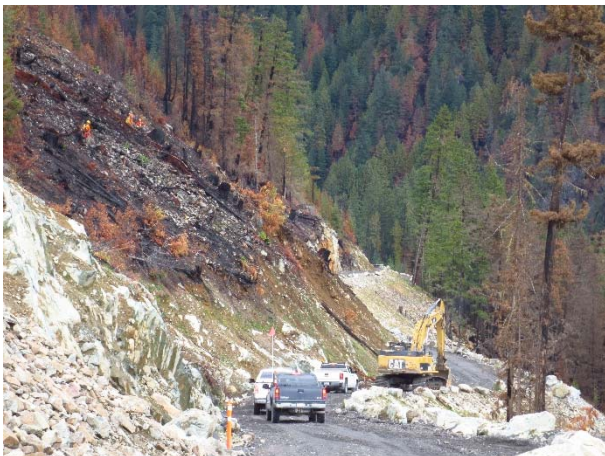
Photo 20 – Slope consolidation works on BDRHEF intake access road (September 2, 2015).
