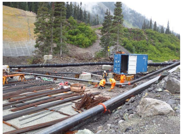
Photo 8 – ULRHEF intake dewatering system repair works (September 2, 2015).
