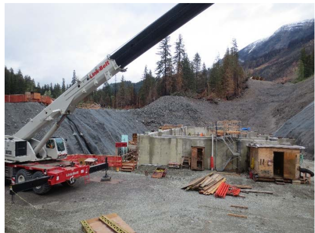
Photo 17 – Clean-up and site preparation at the ULRHEF powerhouse (September 2, 2015).
