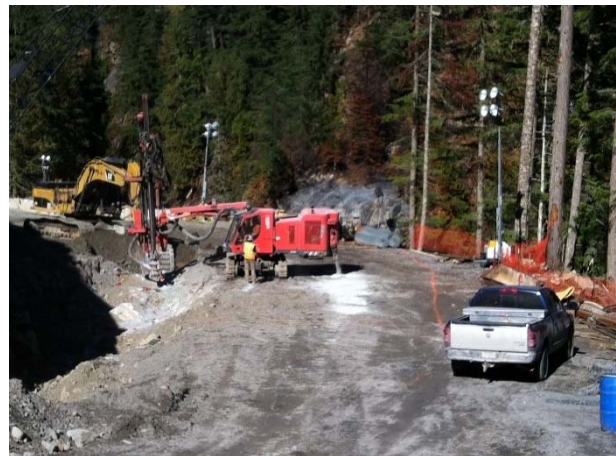
Photo 21 – Preparation for blasting and excavation of ramp at BDRHEF intake (September 10, 2015).
