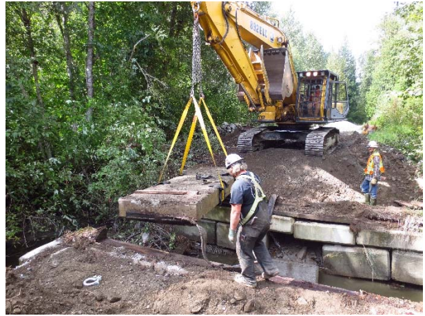
Photo 27 – Bridge installation works at MB59 (September 4, 2015).
