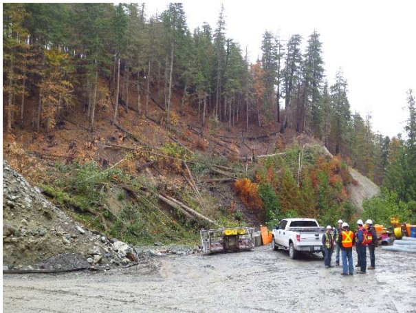
Photo 15 – Kick-off meeting for Truckwash Creek penstock crossing clearing works (September 2, 2015).
