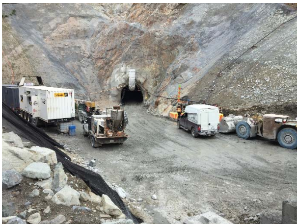
Photo 11 – Current conditions at the ULRHEF downstream tunnel portal (September 7, 2015).
