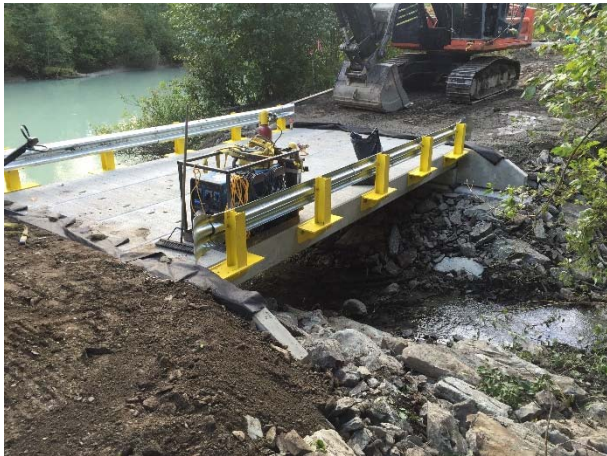
Photo 28 – Bridge installed at MB59 (September 7, 2015).
