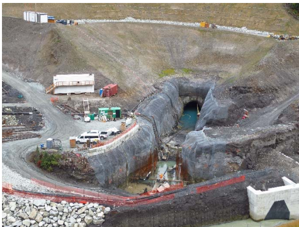
Photo 7 – Current conditions at the ULRHEF intake (September 2, 2015).
