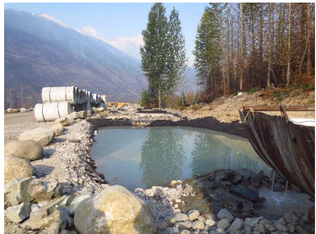
Photo 17 – Conditions within the BDRHEF powerhouse setting ponds. (August 27, 2015).
