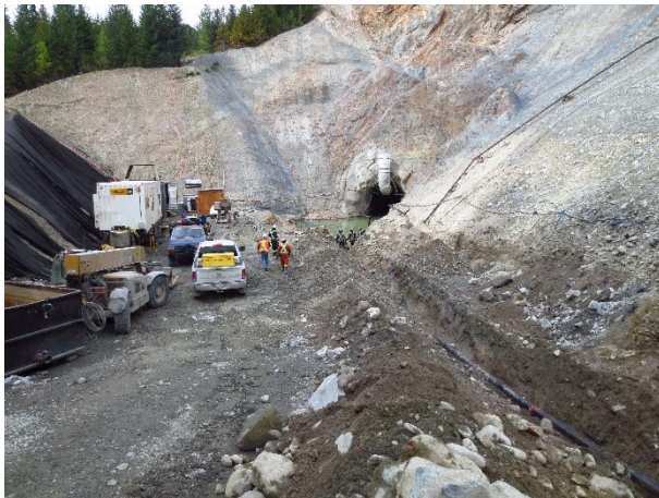
Photo 9 – Burying the dewatering pipes at the ULRHEF downstream tunnel portal (August 28, 2015).
