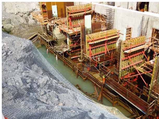
Photo 13 – Dewatering of the ULRHEF powerhouse (August 26, 2015).
