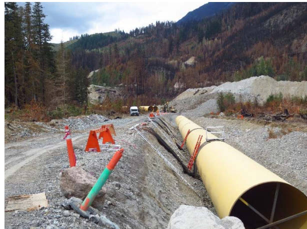
Photo 12 – Penstock installation currently on hold. (August 28, 2015).
