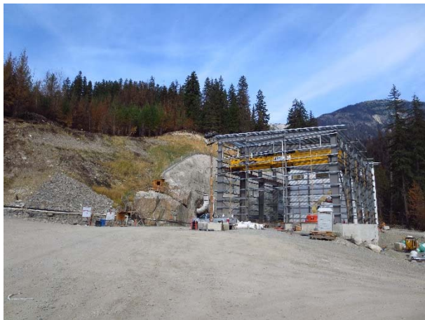
Photo 16 – Works remain on hold at the BDRHEF powerhouse (August 26, 2015).
