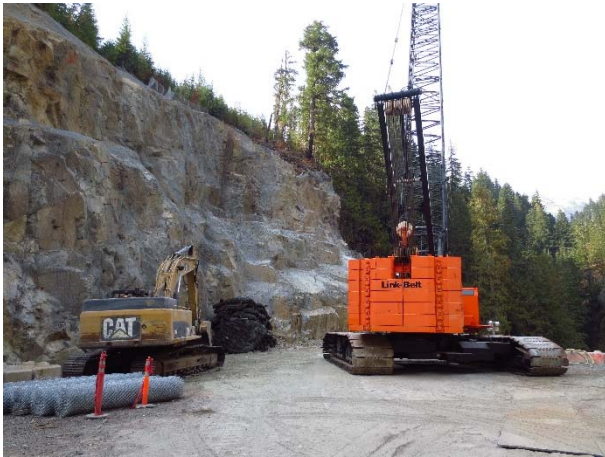
Photo 15 – Works on hold at the BDRHEF intake (August 26, 2015).
