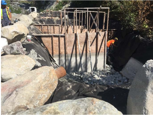
Photo 7 – Repairs underway in the downstream infiltration ponds (August 12, 2015).
