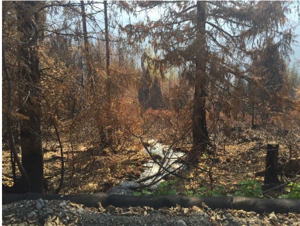
Photo 1 – Stream 9A RVMA downstream of the magazine access road crossing following the removal of danger trees. (August 12, 2015).
