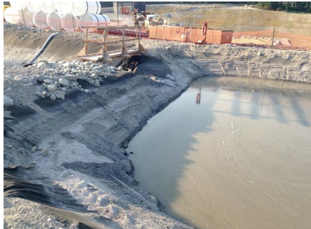
Photo 6 – Discharge of the initial pulse of sediment laden water was directed to water treatment ponds (August 27, 2015).
