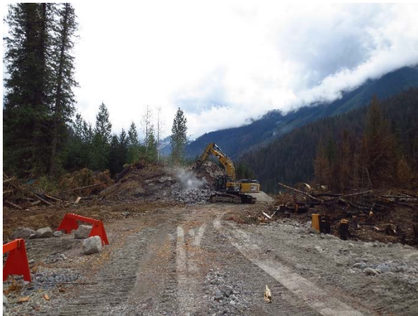
Photo 11 – Breaking up the large rock at 3+900 of the penstock alignment (August 28, 2015).
