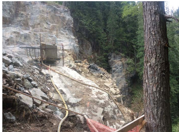
Photo 10 – BDRHEF crane pad area following blast (June 30, 2015).
