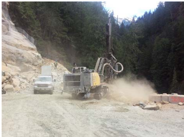
Photo 9 – Drilling at BDRHEF crane pad (June 30, 2015).
