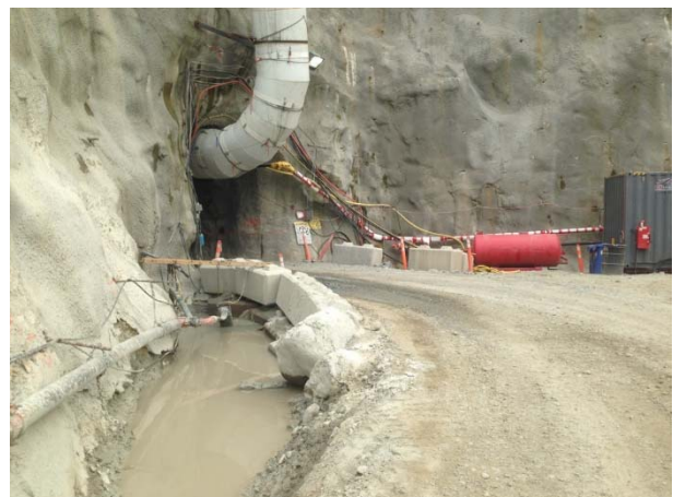
Photo 14 – BDRHEF downstream tunnel portal (June 30, 2015).
