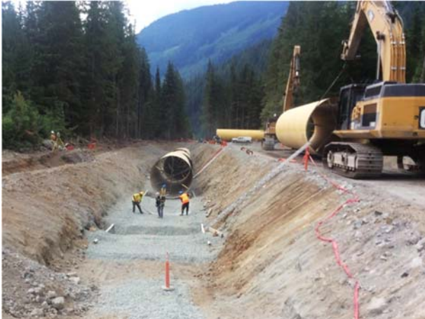
Photo 6 – Penstock installation at 3+850 (June 30, 2015).
