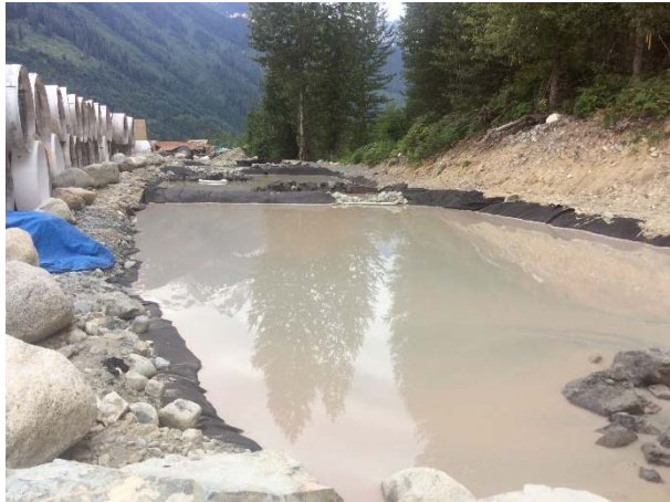
Photo 15 – BDRHEF powerhouse and downstream tunnel portal settling ponds (June 30, 2015).
