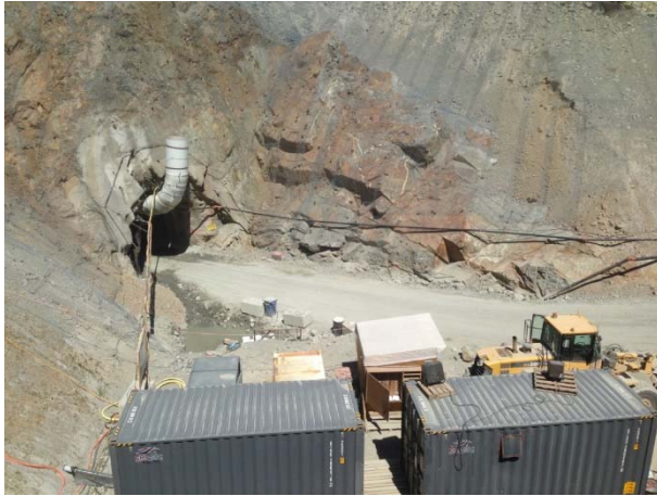
Photo 3 – Current conditions at the ULRHEF downstream tunnel portal (July 1, 2015).
