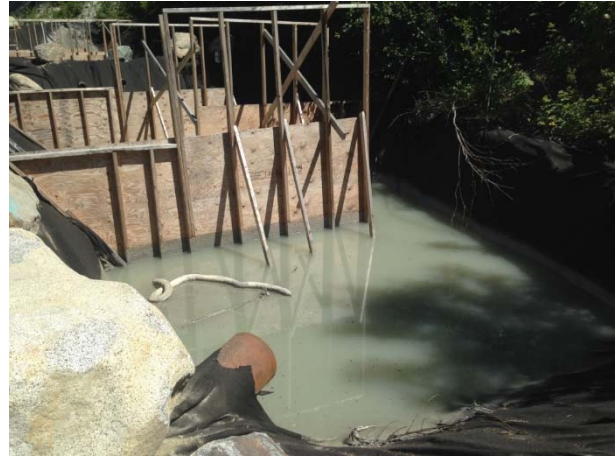
Photo 4 – ULRHEF downstream tunnel portal settling ponds (July 1, 2015).
