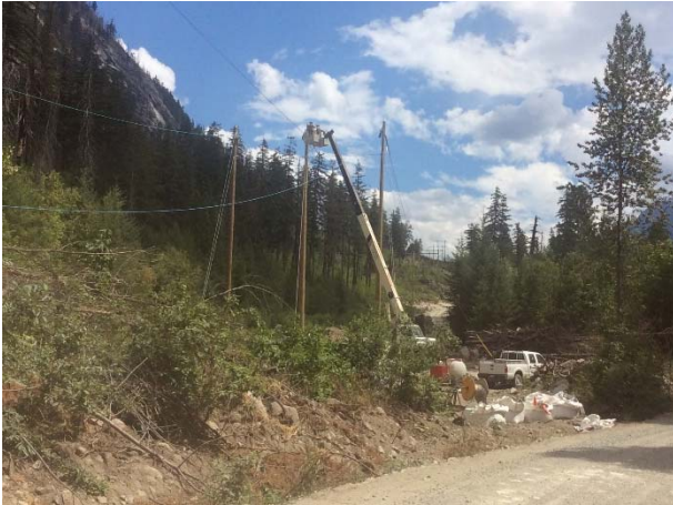
Photo 16 – Clipping conductors in Segment 3 (June 30, 2015).
