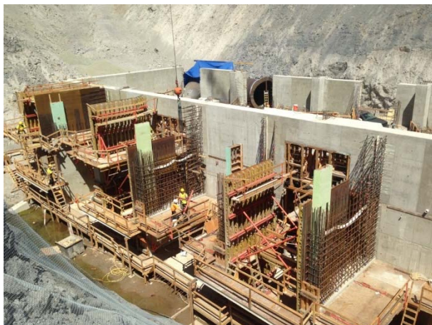
Photo 7 – Rebar installation and formwork at the ULRHEF powerhouse (July 1, 2015).
