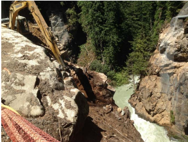
Photo 11 – Excavation of blast material near crane pad (July 1, 2015).
