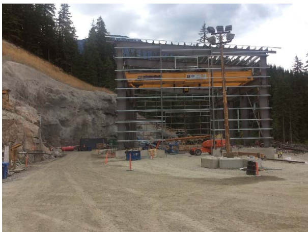
Photo 13 – Construction of BDRHEF powerhouse superstructure (June 30, 2015).
