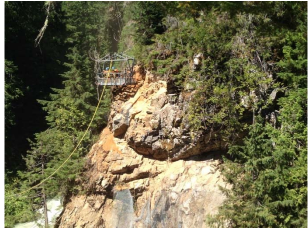
Photo 12 – Scaling works above BDRHEF diversion tunnel (July 1, 2015).
