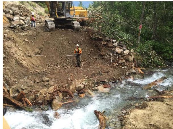
Photo 20 – Preparing footing for the new bridge following completion of the old bridge removal (June 24, 2015).
