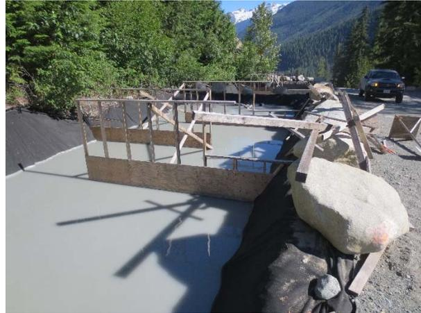
Photo 8 – ULRHEF downstream portal infiltration ponds. Water has not yet discharged from the second pond (June 26, 2015).
