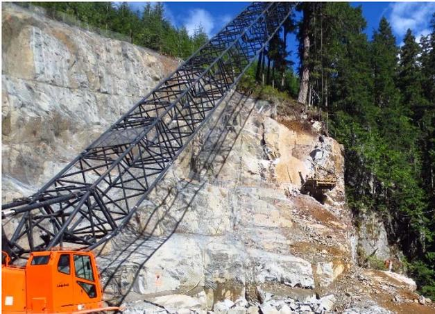
Photo 14 – Crane and man basket used for slope stabilization works (June 21, 2015).
