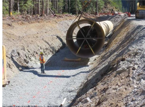
Photo 10 – Penstock installation on prepared bedding (June 26, 2015).
