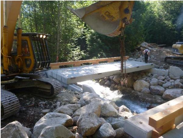
Photo 21 – Placement of the Vans Creek bridge deck (June 27, 2015).
