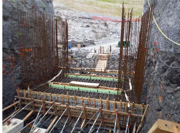
**Photo 4 – Completed form work and rebar immediately prior to the first concrete pour for the intake structure (June 24, 2015).**
