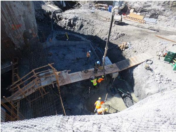
**Photo 5 – Concrete pour for the intake structure (June 26, 2015).**
