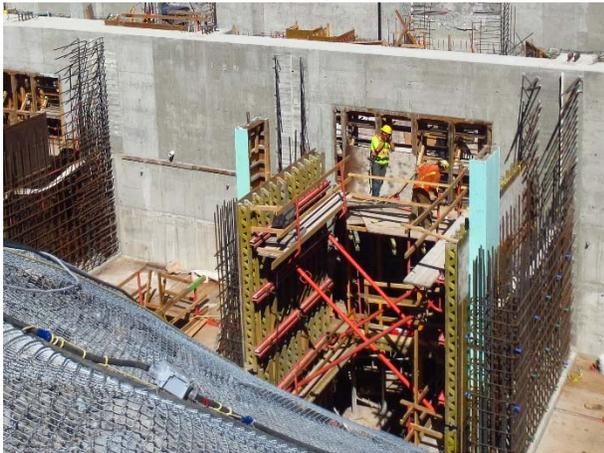
**Photo 11 – Rebar installation and formwork at the ULRHEF powerhouse (June 26, 2015).**
