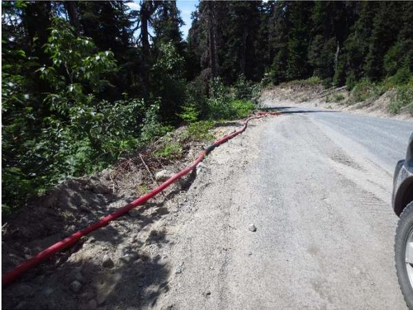
Photo 1 – Installation of temporary power cable along the Lillooet River FSR near KM 47 (June 22, 2015).
