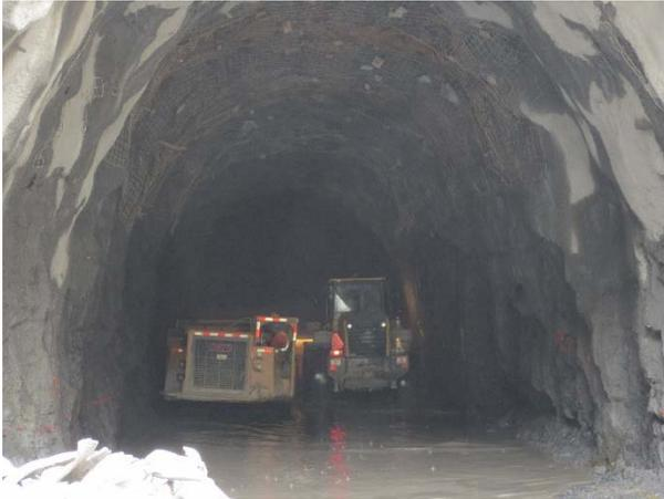
**Photo 3 – Conditions within the ULRHEF upstream tunnel during excavation of blast rock (June 24, 2015).**
