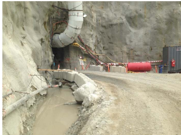
Photo 18 – BDRHEF downstream tunnel portal (June 17, 2015).
