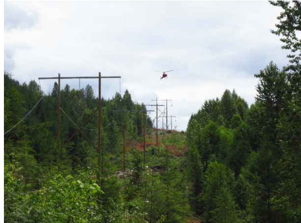
Photo 21 – Pole stringing in Segment 7 (June 20, 2015).
