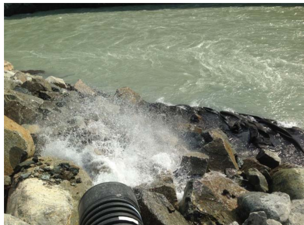
Photo 6 – Discharging clean seepage water directly to Lillooet River (June 17, 2015).
