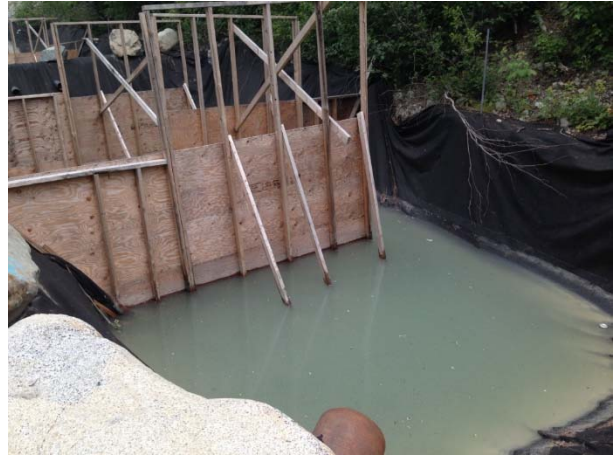
Photo 10 – ULRHEF downstream tunnel portal settling ponds (June 16, 2015).
