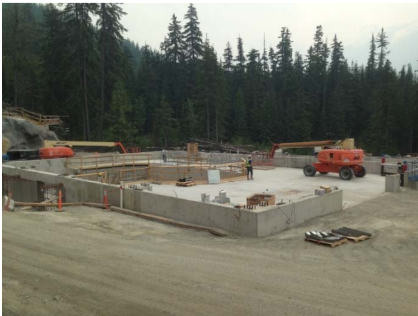
Photo 17 – Current conditions at the BDRHEF powerhouse (June 17, 2015).
