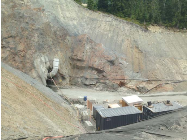
Photo 9 – Current conditions at the ULRHEF downstream tunnel portal (June 16, 2015).
