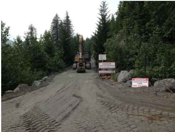
Photo 1 – Capping and re-grading at penstock access road (June 17, 2015).
