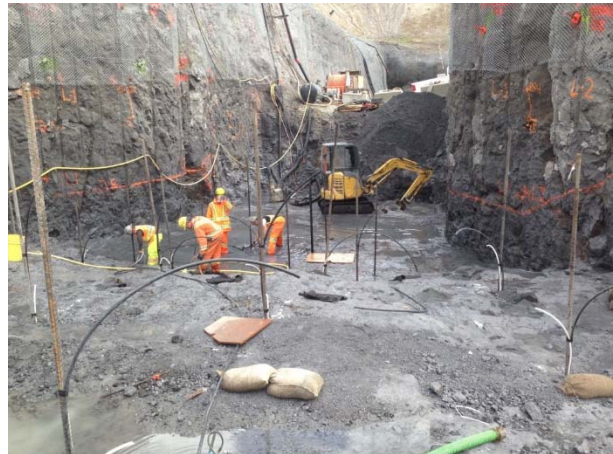
Photo 4 – Applying resin to anchor bolts at ULRHEF intake (June 19, 2015).
