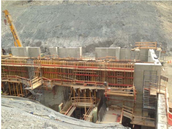
Photo 13 – Rebar installation and formwork at the ULRHEF powerhouse (June 17, 2015).
