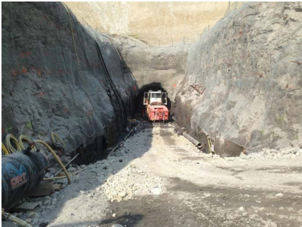
Photo 3 – ULRHEF upstream tunnel portal (June 16, 2015).
