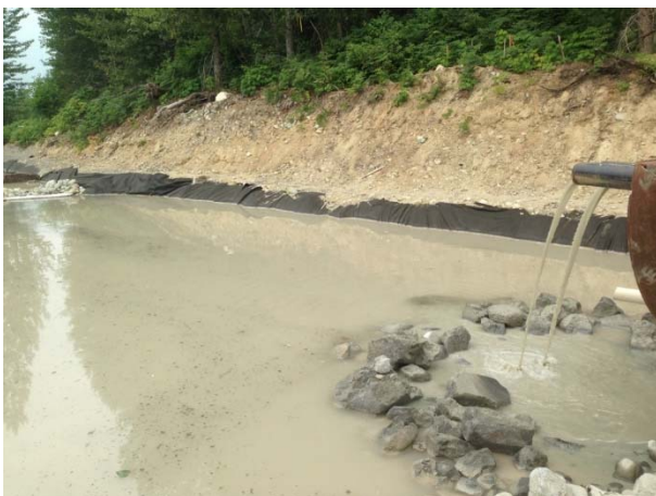
Photo 19 – BDRHEF downstream tunnel portal and powerhouse settling ponds (June 17, 2015).
