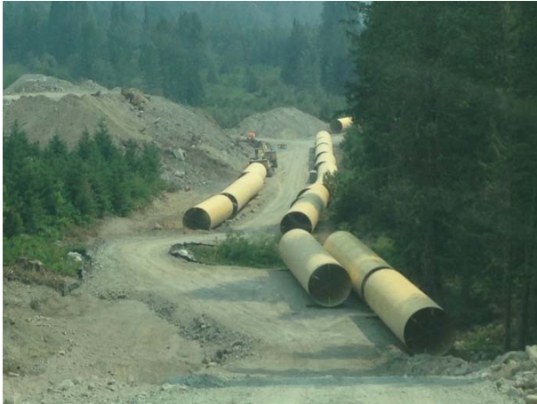
Photo 12 – Penstock staged near ASTR04 (June 16, 2015).
