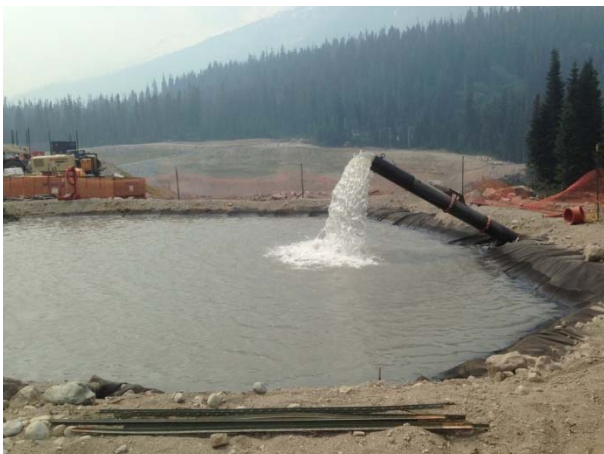
Photo 5 – ULRHEF intake and upstream tunnel portal sediment basins (June 17, 2015).
