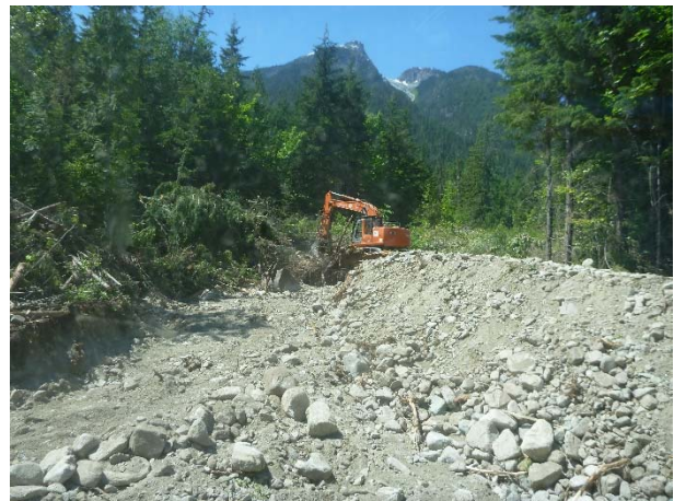
Photo 21 – Stream 261a berm construction (June 9, 2015).
