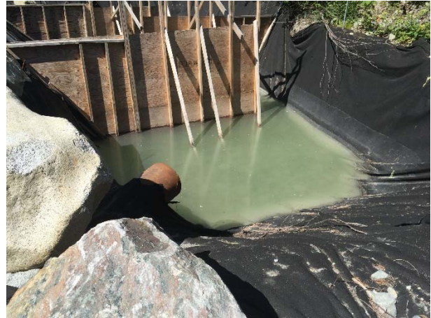
Photo 7 – ULRHEF downstream portal settling ponds (June 8, 2015).
