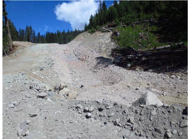
Photo 10 – Bulk excavation for penstock trench near 3+325 (June 12, 2015).
