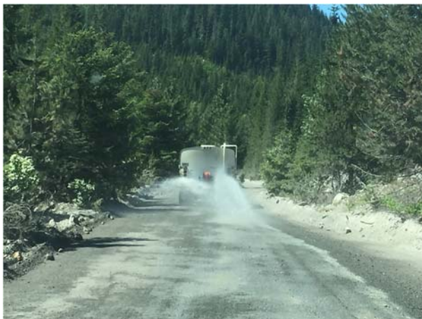
Photo 1 – Water applied to the Lillooet River FSR for dust suppression (June 8, 2015).
