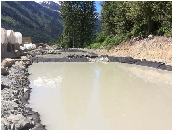
Photo 18 – BDRHEF powerhouse settling ponds (June 8, 2015).
