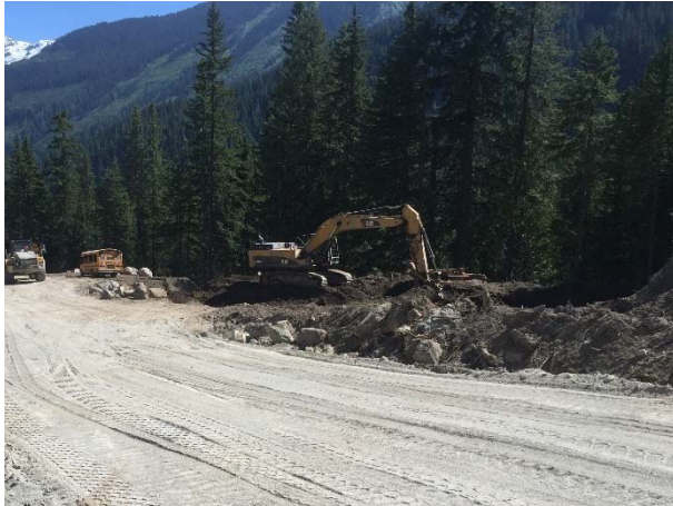
Photo 9 – Re-contouring of organic material stockpile to allow for penstock staging (June 8, 2015).
