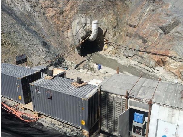
Photo 6 – Current conditions at the ULRHEF downstream tunnel portal (June 8, 2015).
