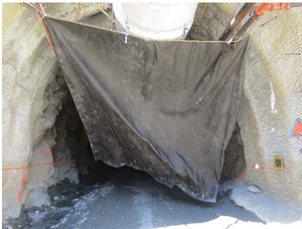
Photo 8 – Geotextile membrane installed over entrance to downstream tunnel portal (June 9, 2015).
