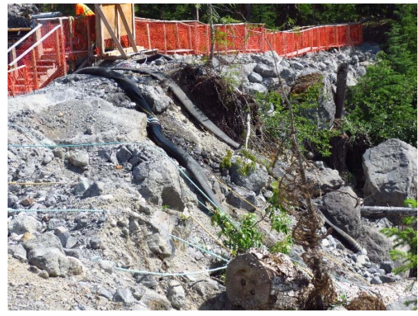
Photo 14 – ULRHEF powerhouse dewatering hoses relocated upstream of previous discharge location (June 10, 2015)
