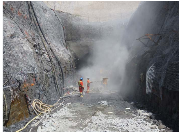
Photo 3 – Cleaning shotcrete machine at ULRHEF upstream tunnel portal (June 13, 2015).
