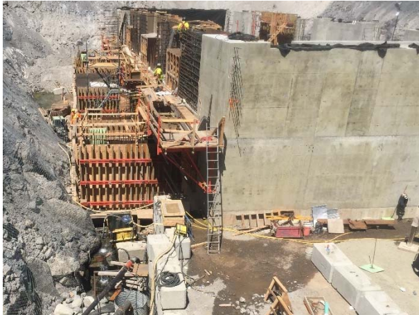
Photo 11 – Rebar installation and formwork at the ULRHEF powerhouse (June 8, 2015).
