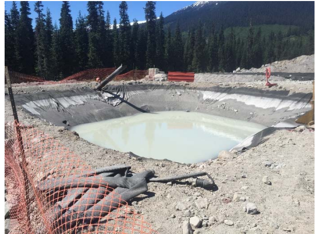
Photo 5 – ULRHEF Intake and upstream tunnel portal sediment basins (June 8, 2015).
