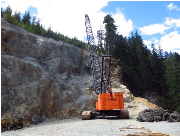
Photo 15 – Crane and man basket used for slope stabilization works (June 12, 2015).
