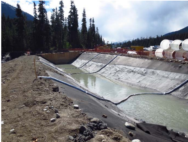
Photo 4 – ULRHEF Intake and upstream tunnel portal sediment basins (June 8 , 2015).
