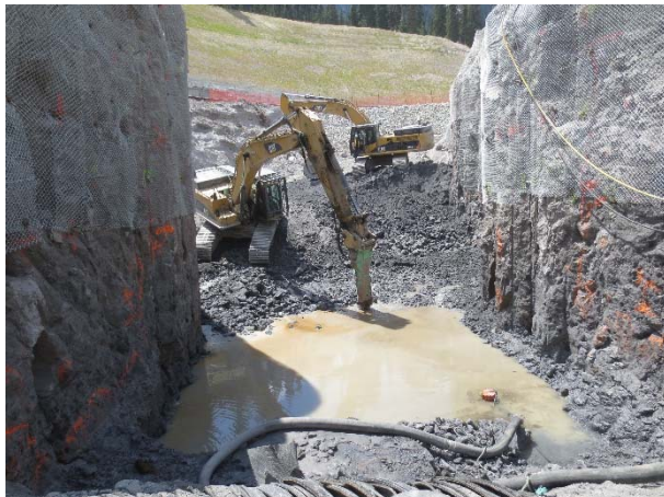
Photo 2 – Rock hammering at ULRHEF intake excavation (June 13, 2015).
