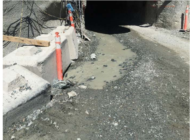
Photo 17 – BDRHEF downstream tunnel portal (June 8, 2015).
