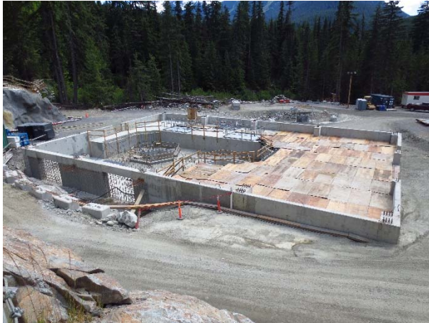
Photo 16 – Current conditions at the BDRHEF powerhouse (June 12, 2015).
