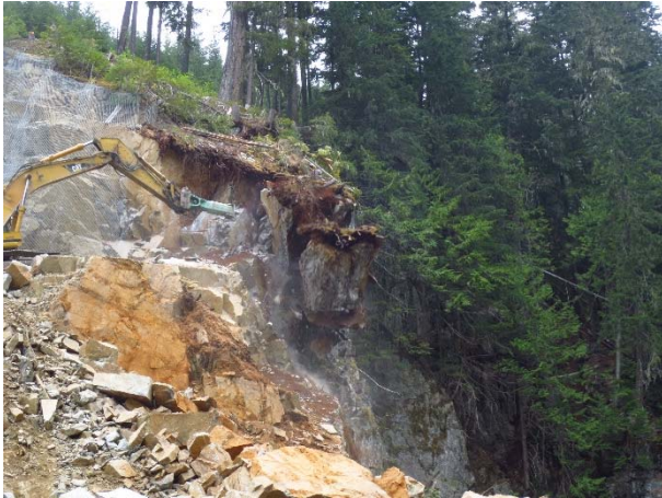
Photo 20 – Rock hammering and excavation at the intake (May 24, 2015).
