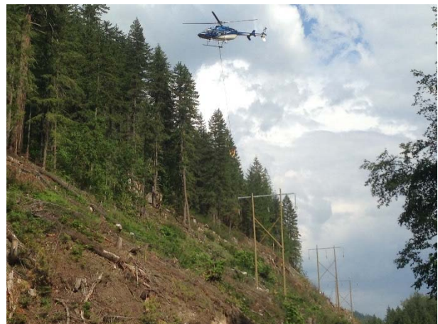
Photo 27 – Stringing conductor in Segment 5 (May 26, 2015)
