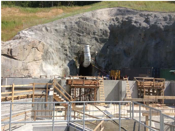
Photo 22 – Current conditions at the BDRHEF powerhouse (May 27, 2015).
