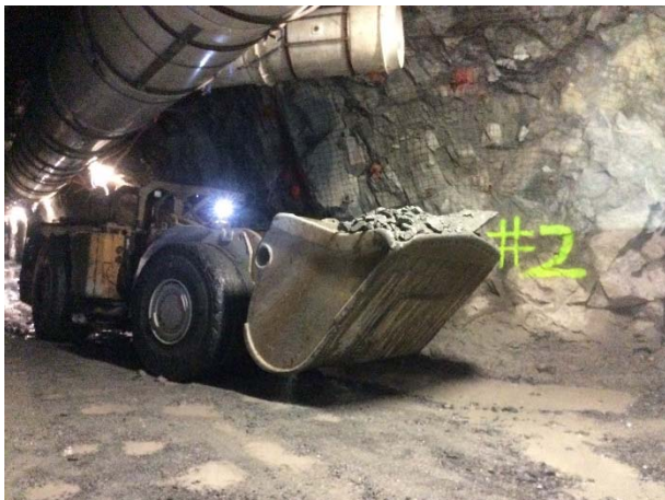
Photo 24 – Mucking blast rock within the BDRHEF tunnel (May 27, 2015).
