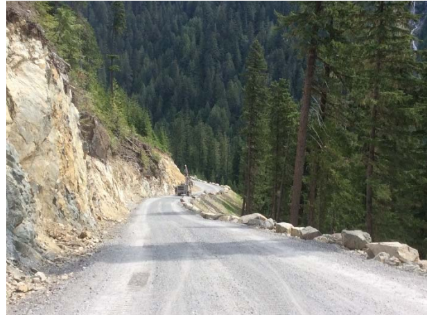
Photo 21 – Conditions along the BDRHEF intake access road (May 28, 2015).
