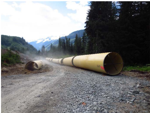
Photo 14 – Penstock delivered and stored along the penstock alignment (May 30, 2015).
