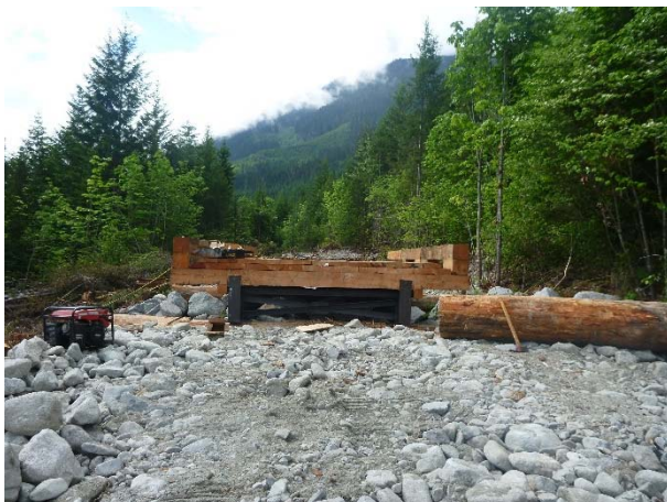
Photo 26 – Bridge installation at crossing 261a (May 26, 2015).
