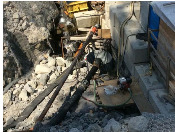
Photo 19 – ULRHEF powerhouse sump (May 27, 2015)
