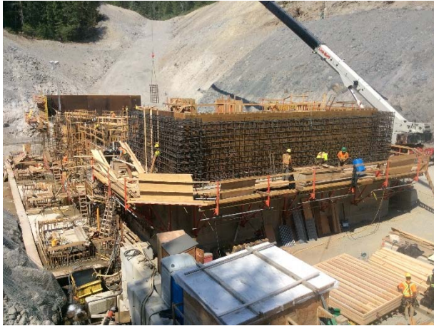
Photo 16 – Rebar installation and formwork at the ULRHEF powerhouse (May 27, 2015).
