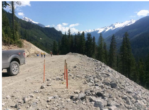
Photo 15 – Penstock fill completed near Truckwash Creek (May 27, 2015).
