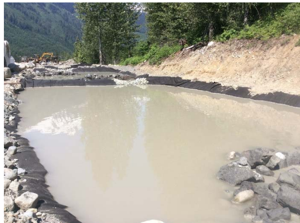
Photo 25 – BDRHEF powerhouse settling ponds (May 27, 2015).
