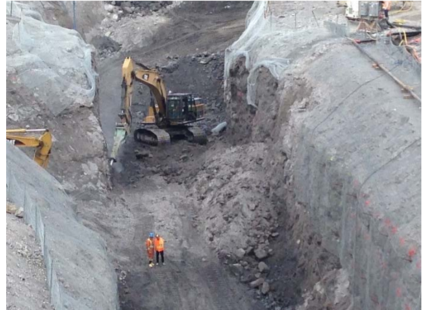
Photo 7 – Rock hammering within the ULRHEF intake/ upstream tunnel portal excavation (May 25, 2015).
