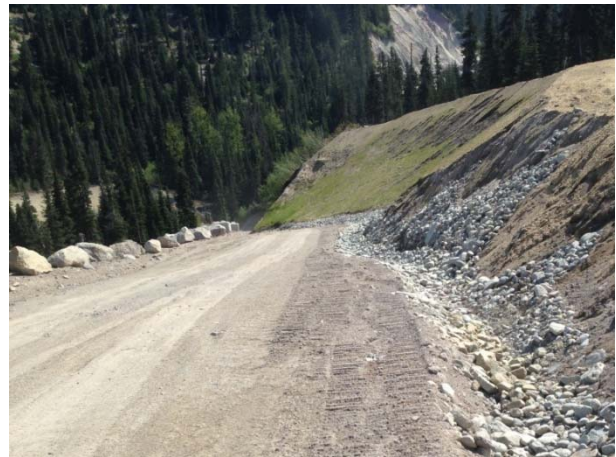
Photo 2 – Ditch maintenance completed at KM 49.25 on the Lillooet River FSR (May 19, 2015).
