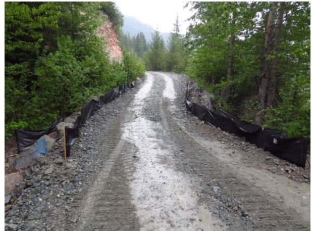
Photo 15 – Silt fencing repaired at ASTR04 crossing on Truckwash 2 access road (May 17, 2015).
