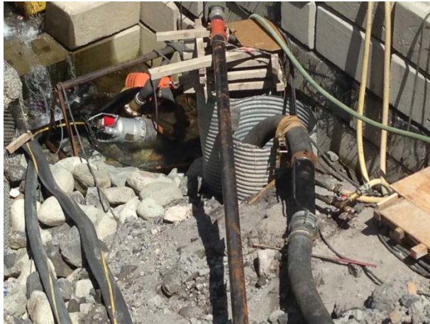
Photo 20 – ULRHEF powerhouse sump (May 19, 2015).
