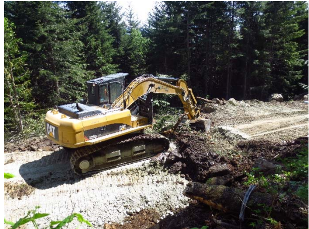
Photo 30 – Culvert installation on road 322.1 in Segment 13 (May 20, 2015).
