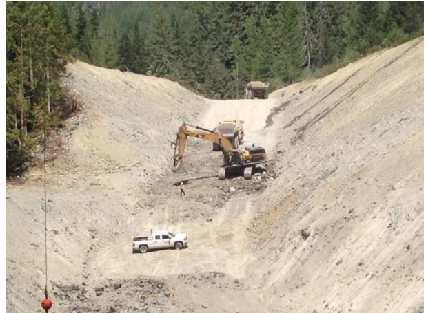
Photo 13 – Penstock bulk excavation at 4+060 (May 19, 2015).
