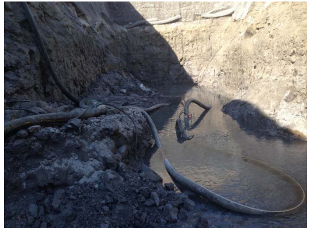
Photo 6 – Dewatering ULRHEF upstream portal excavation to sediment basins (May 18, 2015).
