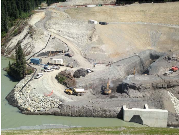
Photo 3 – Current conditions at the ULRHEF intake (May 18, 2015).
