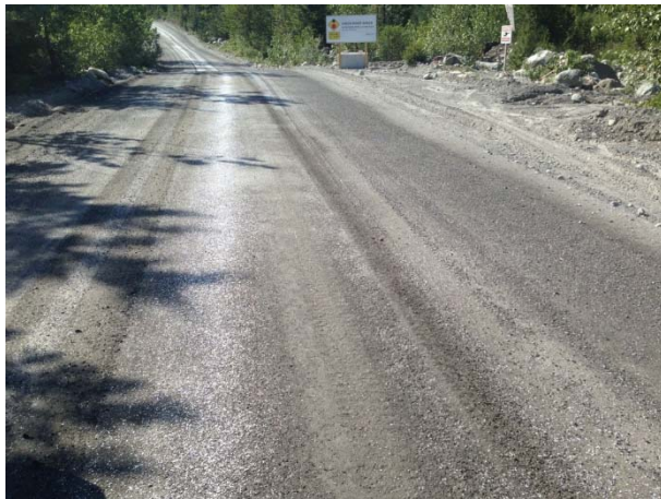
Photo 1 – Calcium chloride applied to Lillooet River FSR at KM 38 for dust suppression (May 19, 2015).
