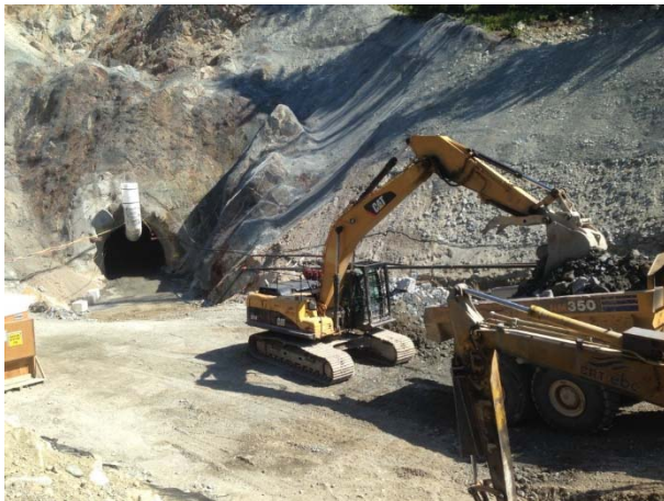
Photo 9 – Tunnel mucking at ULRHEF downstream tunnel portal (May 18, 2015).
