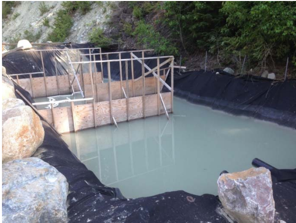
Photo 11 – ULRHEF downstream tunnel portal settling ponds (May 18, 2015).
