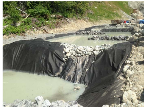
Photo 28 – BDRHEF powerhouse settling ponds (May 19, 2015).
