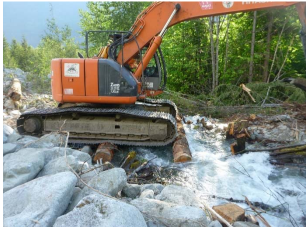
Photo 32 – Excavator crossing stream 261a (May 21, 2015).
