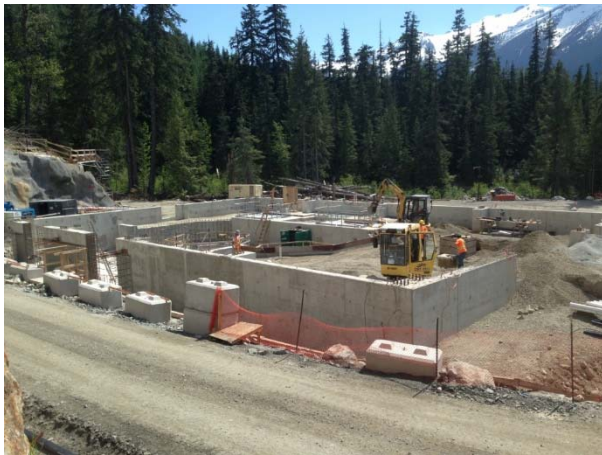
Photo 25 – Current conditions at the BDRHEF powerhouse (May 19, 2015).
