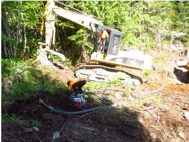
Photo 29 – Pump prepared for culvert installation on road 322.1 in Segment 13 (May 20, 2015).
