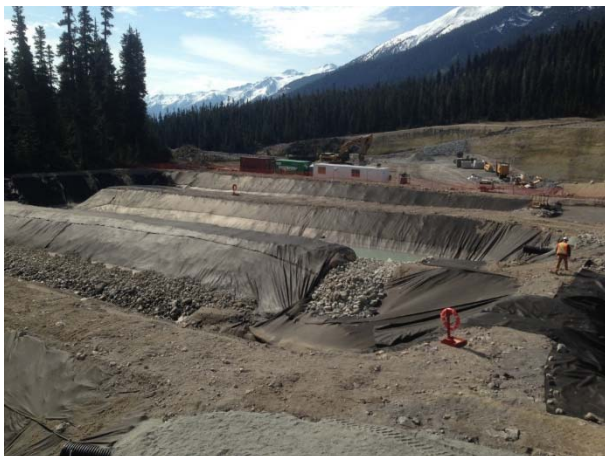
Photo 7 – ULRHEF intake sediment basins (May 18, 2015).
