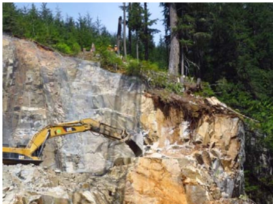
Photo 24 – Rock hammering and excavation at the intake (May 24, 2015).
