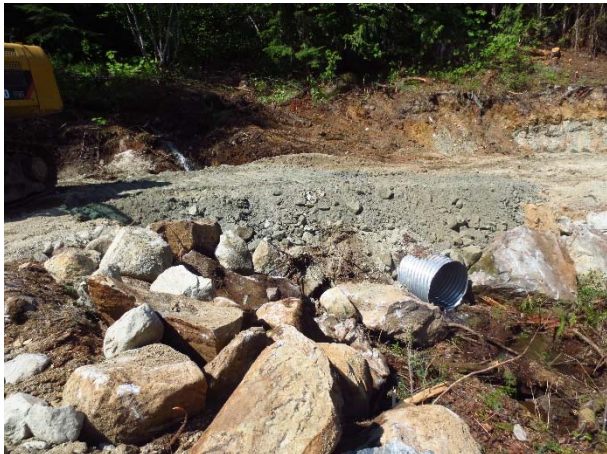
Photo 31 – Culvert installation on road 322.1 in Segment 13 (May 20, 2015).
