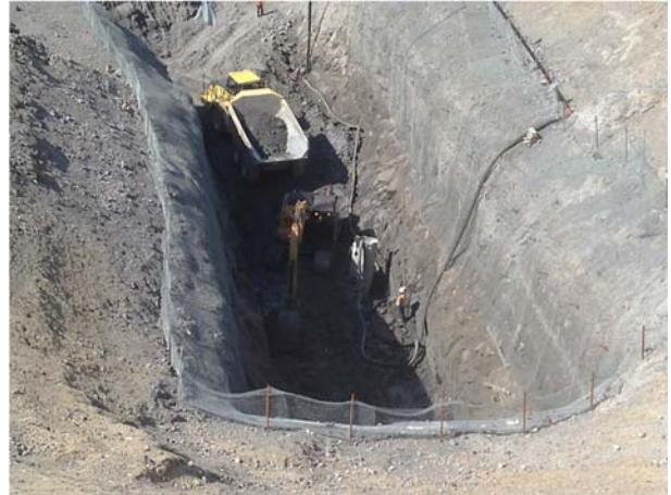
Photo 4 – ULRHEF upstream portal excavation (May 18, 2015).
