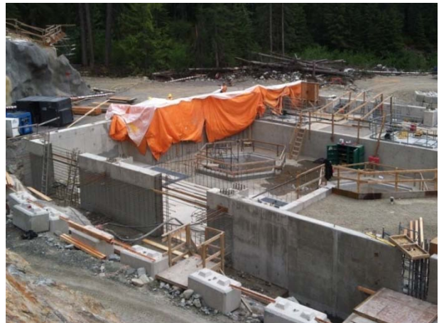
Photo 26 – Tarp over uncured concrete at BDRHEF powerhouse (May 23, 2015).
