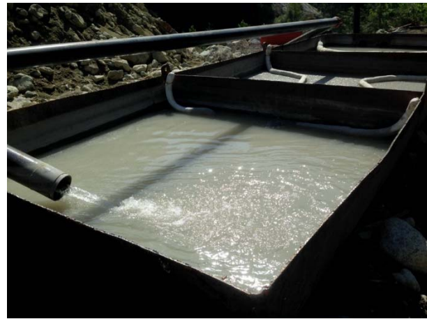
Photo 10 – Dewatering ULRHEF downstream tunnel portal to oil water separator (May 18, 2015).
