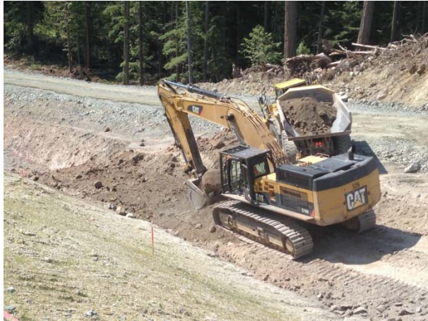
Photo 12 – Penstock bulk excavation at 3+325 (May 18, 2015).
