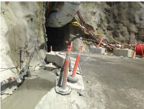
Photo 27 – Current conditions at the BDRHEF tunnel portal (May 19, 2015).
