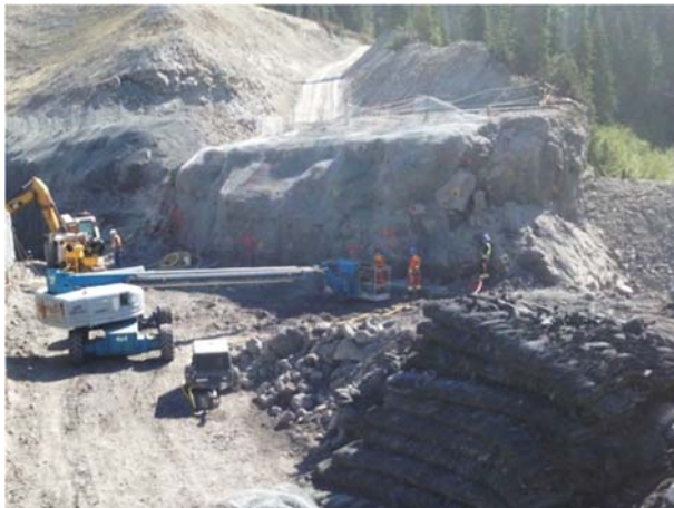
Photo 5 – Blast preparation between upstream portal excavation and downstream cofferdam (May 18, 2015).
