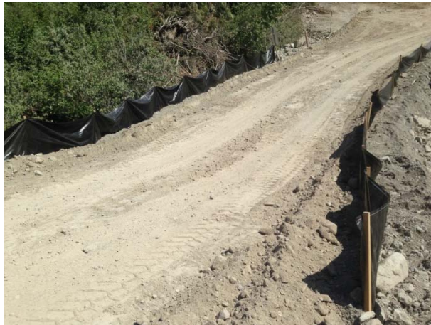
Photo 14 – Silt fencing repairs at ASTR03 crossing (May 19, 2015).
