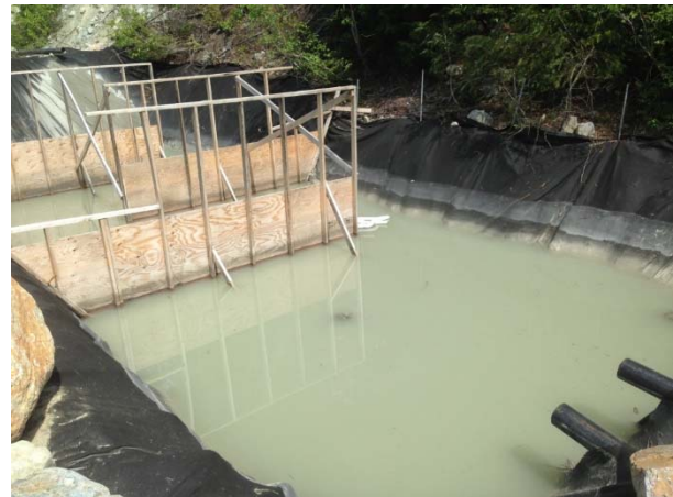
Photo 10 – ULRHEF downstream tunnel portal settling ponds (May 12, 2015).
