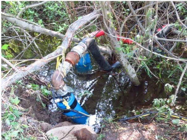
Photo 15 – Pumps installed above Lillooet River FSR at 42.25km (May 15, 2015).
