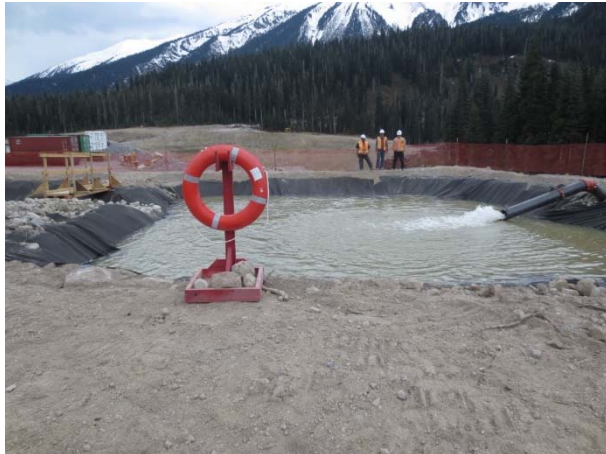
Photo 7 – Dewatering upstream portal excavation to sediment basins (May 13, 2015).
