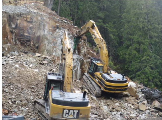
Photo 21 – Rock hammering and excavation continued at BDRHEF intake (May 11, 2015).
