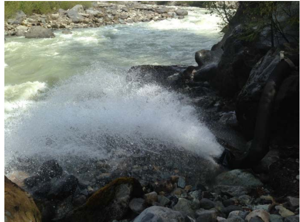
Photo 18 – Outlet of 10” powerhouse sump dewatering hose (May 10, 2015).
