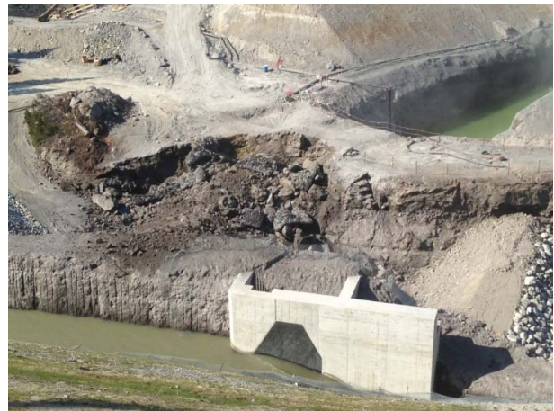
Photo 4 – Conditions after blast between downstream cofferdam and portal excavation (May 11, 2015).
