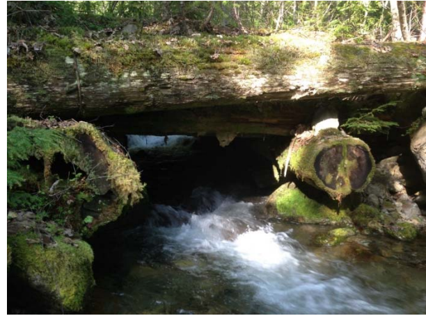
Photo 25 – Old log box culvert over Vans Creek (May 11, 2015).
