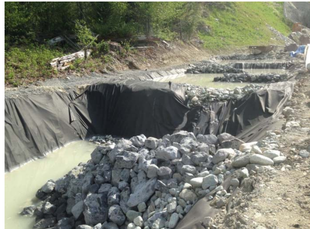
Photo 23 – Dewatering the BDRHEF tunnel to settling ponds (May 7, 2015).
