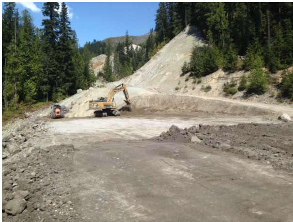
Photo 11 – Fill and compaction works at 2+800 (May 10, 2015).
