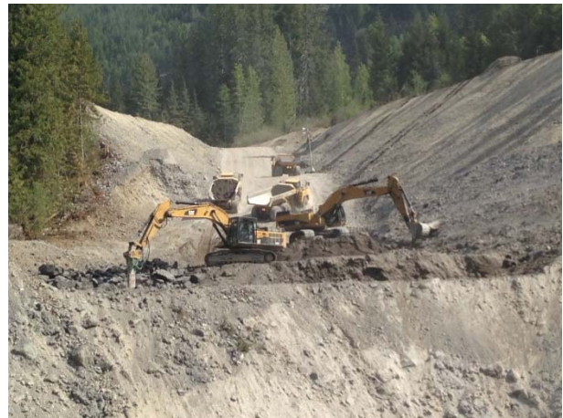
Photo 12 – Penstock excavation at 4+060 (May 10, 2015).
