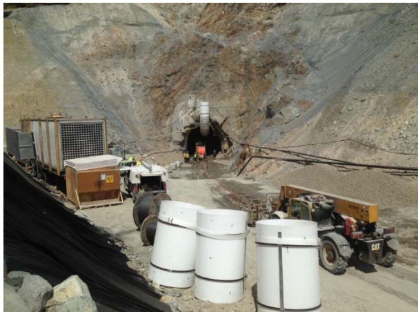
Photo 9 – Current conditions at the ULRHEF downstream tunnel portal (May 12, 2015).
