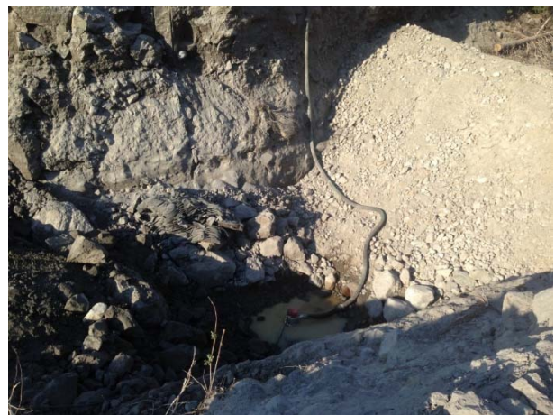
Photo 6 – Pumping sediment-laden water from downstream cofferdam to portal excavation (May 11, 2015).
