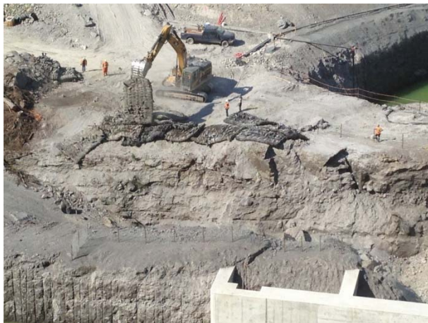
Photo 3 – Blast preparation between downstream cofferdam and portal excavation (May 11, 2015).
