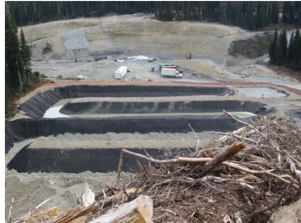
Photo 8 – Intake sediment basins (May 13, 2015).
