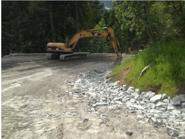
Photo 1 – Ditch maintenance near 43km on the Lillooet River FSR (May 12, 2015).
