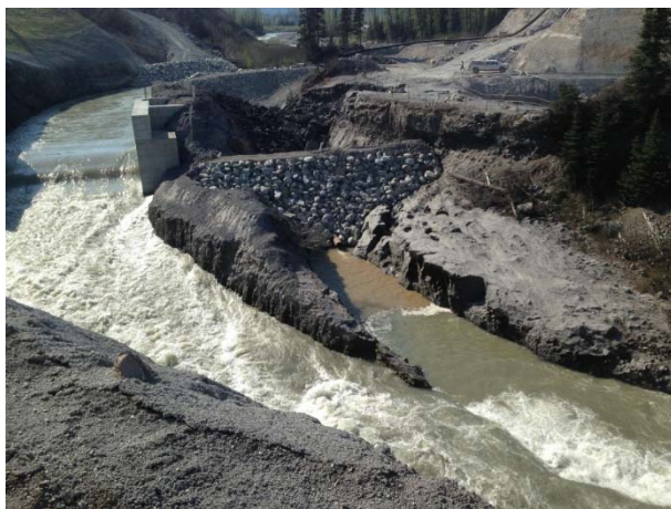
Photo 5 – Sediment-laden water discharging from downstream cofferdam culvert following blast (May 11, 2015).
