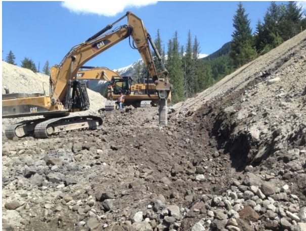
Photo 13 – Penstock excavation at 4+060 (May 12, 2015).
