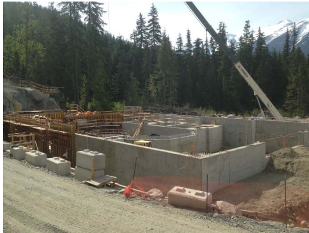
Photo 22 – Current conditions at the BDRHEF powerhouse (May 7, 2015).
