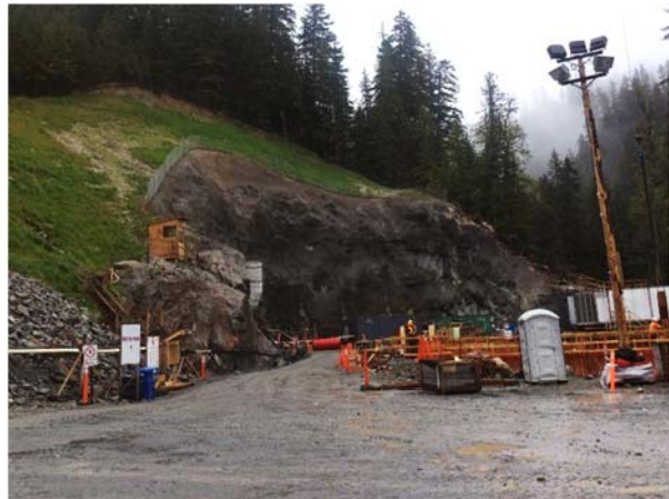
Photo 22 – Current conditions at BDRHEF tunnel portal (May 2, 2015).
