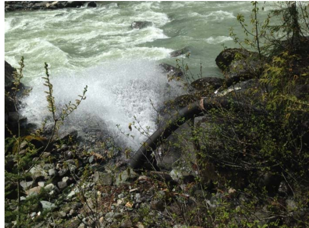
Photo 13 – Dewatering of ULRHEF powerhouse sump to Lillooet River (May 1, 2015).
