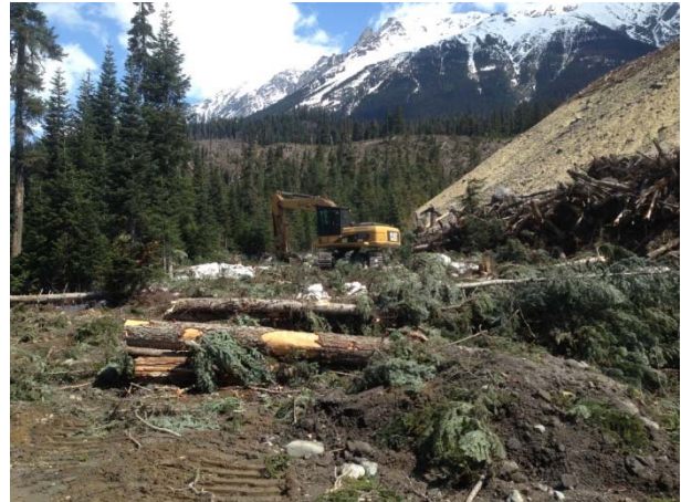
Photo 4 – Machine clearing for spoil pile enlargement (May 2, 2015).
