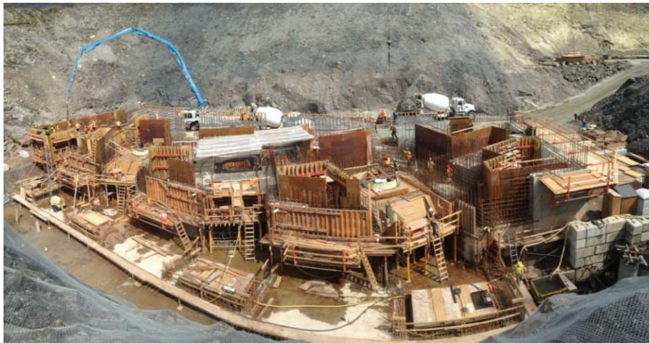
Photo 11 – Current conditions at ULRHEF powerhouse with concrete pour in progress (May 1, 2015).
