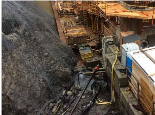
Photo 12 – ULRHEF powerhouse sump (May 1, 2015).
