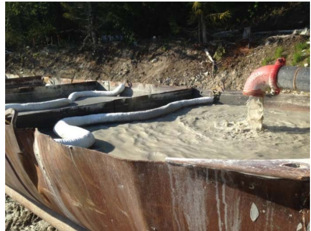
Photo 23 – Dewatering tunnel and powerhouse to oil water separator (May 2, 2015).
