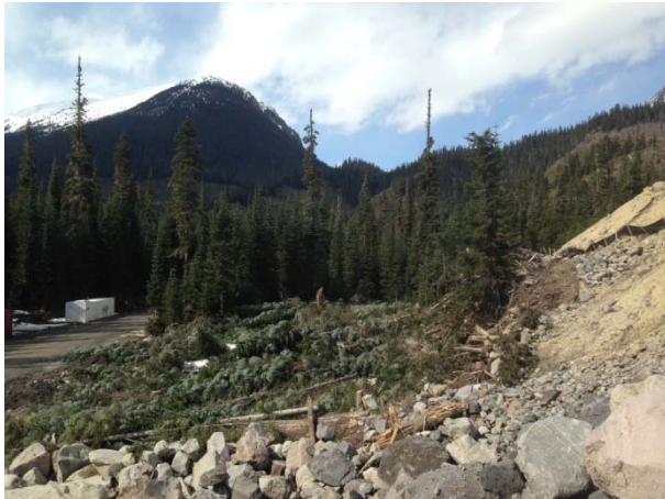
Photo 3 – Hand falling for spoil pile enlargement (May 2, 2015).
