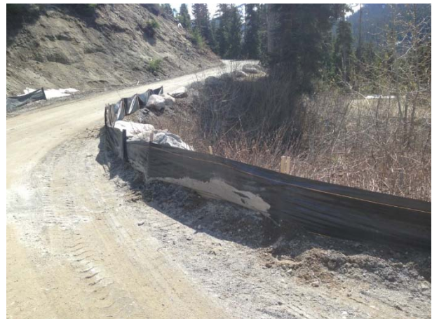
Photo 6 – Silt fencing repaired at 47.5km tributary (May 2, 2015).
