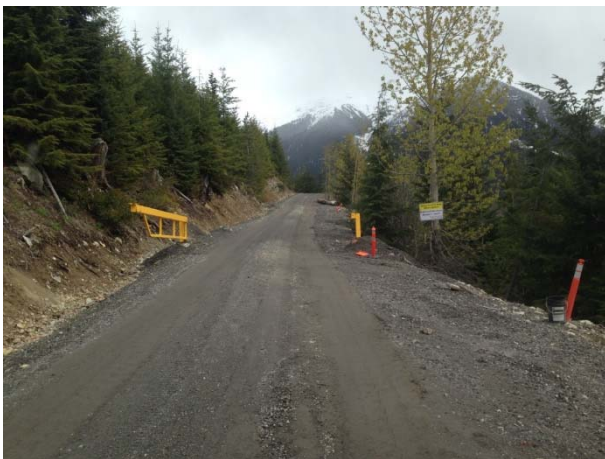
Photo 18 – Gate at 3.5km on the BDRHEF intake access road (May 1, 2015).
