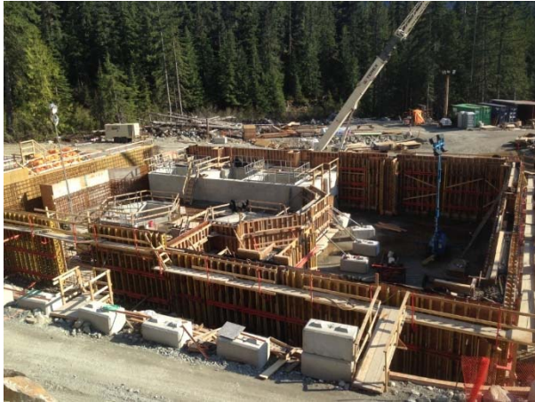
Photo 20 – Current conditions at the BDRHEF powerhouse (May 2, 2015).
