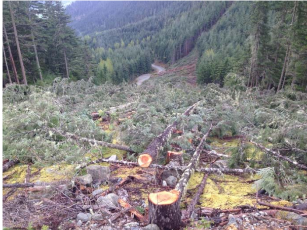
Photo 25 – Hand falling completed for spur road 306.1 in Segment 13 (April 30, 2015).
