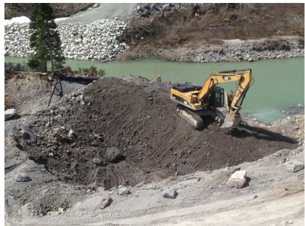
Photo 2 – Sump excavation for wastewater treatment system (May 2, 2015).
