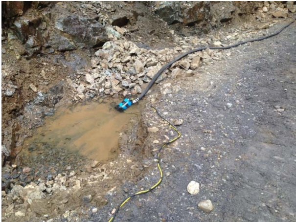
Photo 16 – 2" pump used to convey water around road clearing works at 3.75km on BDRHEF intake access road (May 1, 2015).
