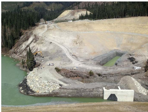
Photo 1 – Current conditions at ULRHEF intake (May 2, 2015).
