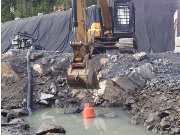
Photo 9 – Pump suspended from excavator at ULRHEF downstream tunnel portal (May 1, 2015).
