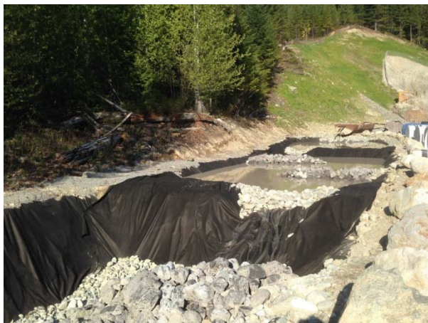
Photo 24 – BDRHEF portal/powerhouse settling ponds (May 2, 2015).
