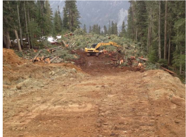
Photo 26 – Building spur road 327.1 in Segment 14 (April 30, 2015).
