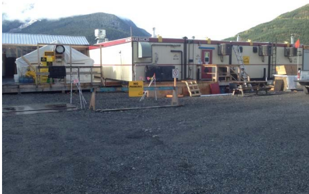
Photo 3 – The area outside of the kitchen trailers was observed to be clean, organized and free of bear attractants (April 24, 2015).
