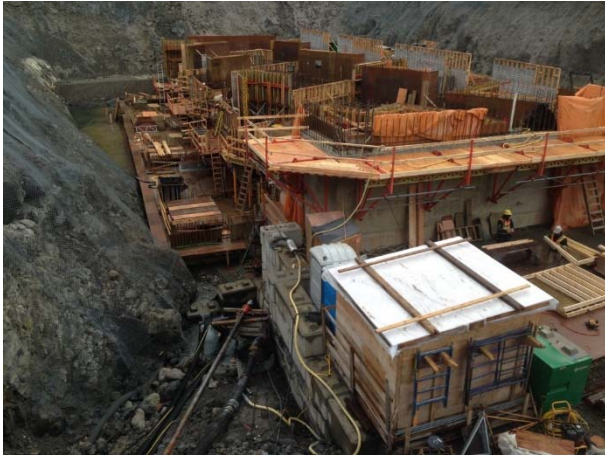
Photo 4 – Current conditions at ULRHEF powerhouse (April 24, 2015).
