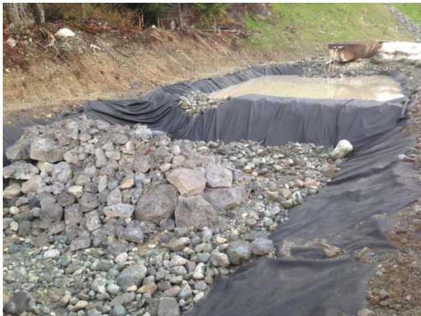
Photo 9 – BDRHEF settling ponds (April 24, 2015).
