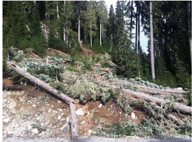
Photo 15 – Falling completed near structure 318 (April 23, 2015).
