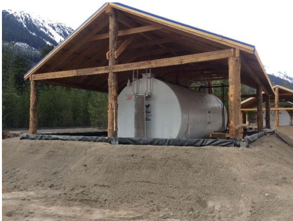
Photo 10 – Construction of temporary generator site in Segment 2 (April 21, 2015).
