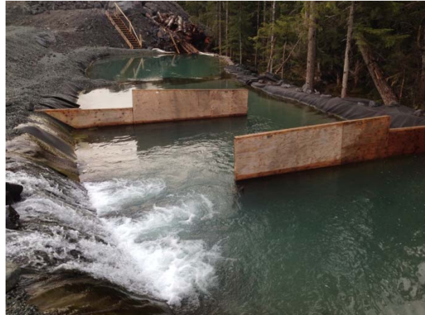
Photo 5 – ULRHEF powerhouse settling ponds (April 24, 2015).
