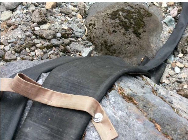
Photo 6 – 10" hose anchored to boulder to restrict movement of hose (April 21, 2015).
