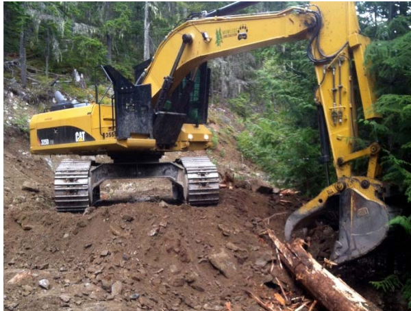
Photo 14 – Culvert installation works at MB50 (April 22, 2015).
