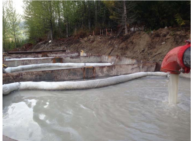
Photo 8 – BDRHEF tunnel dewatering to oil water separator and settling ponds (April 24, 2015).
