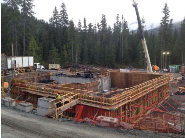
Photo 7 – Current conditions at BDRHEF powerhouse (April 24, 2015).
