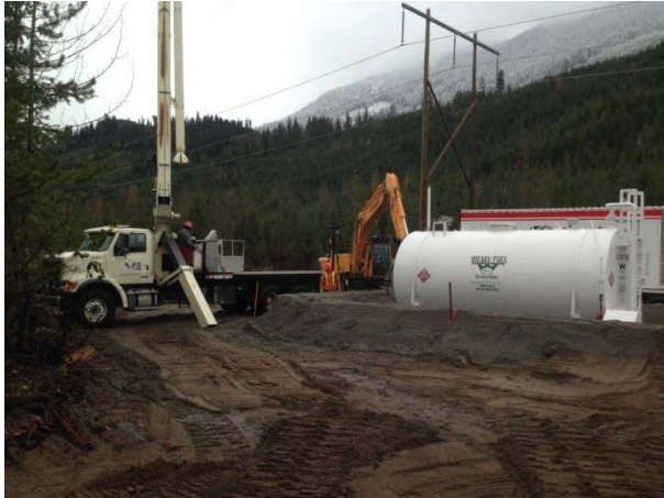
Photo 8 – Construction of temporary generator site in Segment 2 (April 13, 2015).
