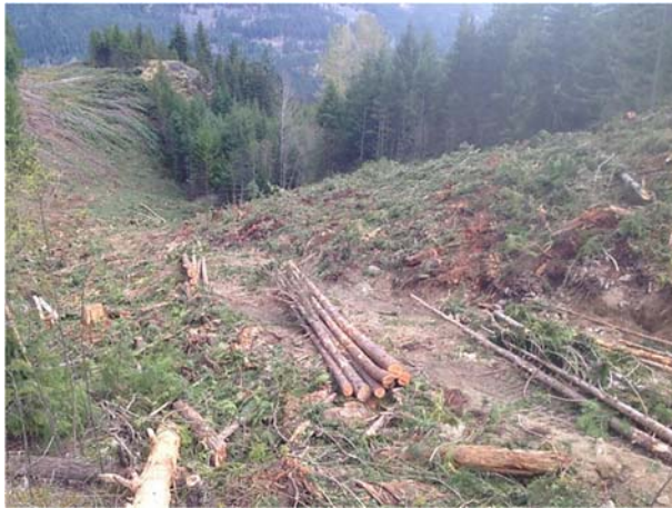
Photo 14 – Hoe chucking and log decking completed in Segment 16 (April 15, 2015).
