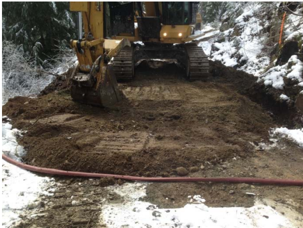
Photo 10 - Culvert installation with diversion in place at MB24 in Segment 12 (April 14, 2015).
