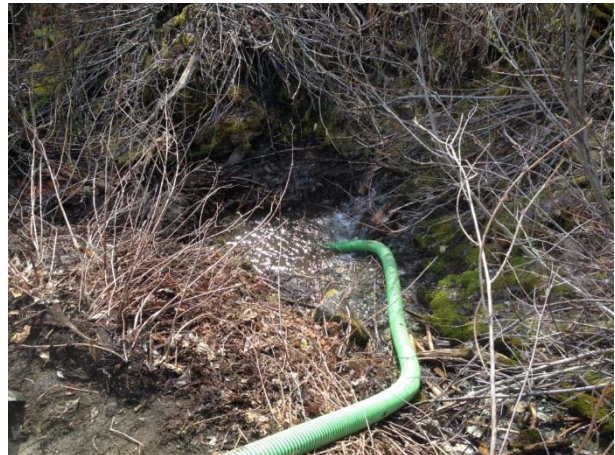
Photo 11 – Sump and 3" pump used to divert water at MB34 (April 15, 2015).
