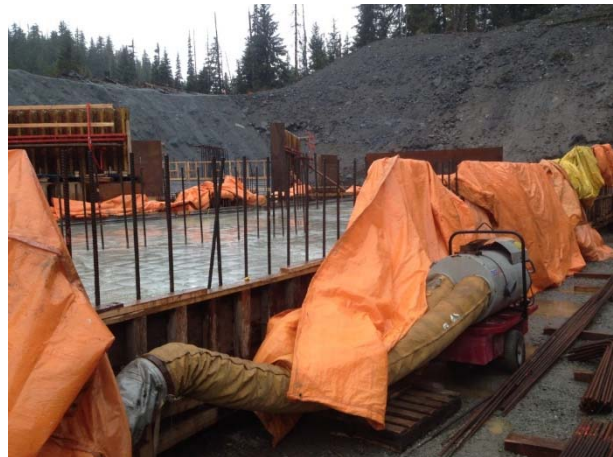
Photo 2 – Concrete poured at ULRHEF powerhouse (April 13, 2015).
