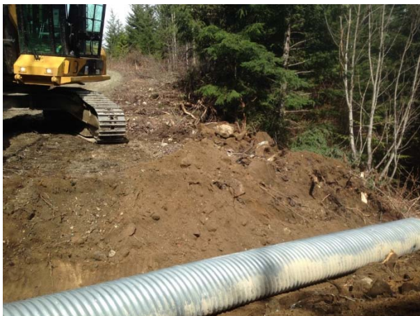
Photo 12 – Culvert installation in progress at MB32 (April 15, 2015).
