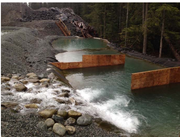
Photo 3 – ULRHEF powerhouse settling ponds (April 13, 2015).
