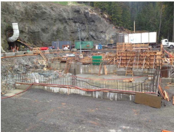
Photo 4 – Current conditions at BDRHEF powerhouse (April 13, 2015).
