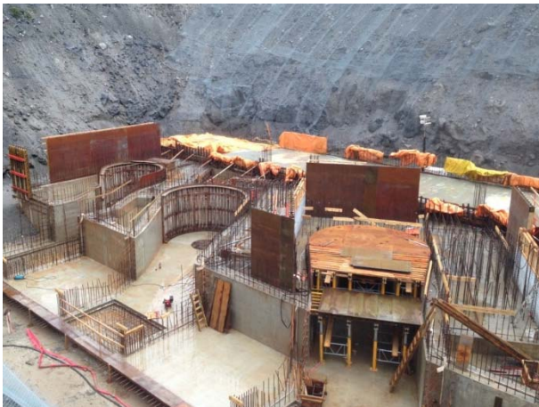
Photo 1 – ULRHEF powerhouse with recently poured concrete in background (April 13, 2015).
