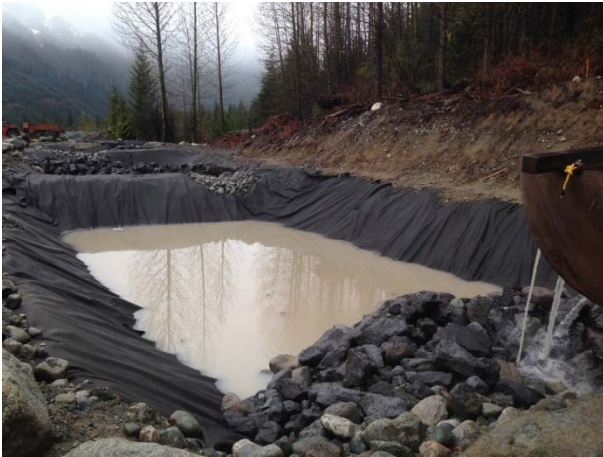
Photo 6 – BDRHEF powerhouse settling ponds (April 13, 2015).
