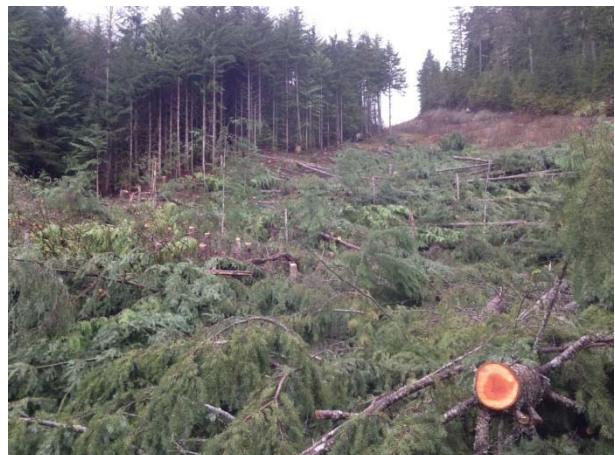
Photo 13 – Falling completed near structure 120 (April 15, 2015).
