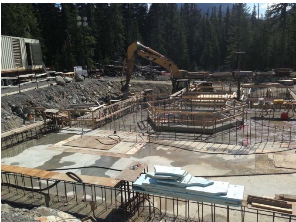
Photo 3 – Current conditions at BDRHEF powerhouse (April 8, 2015).
