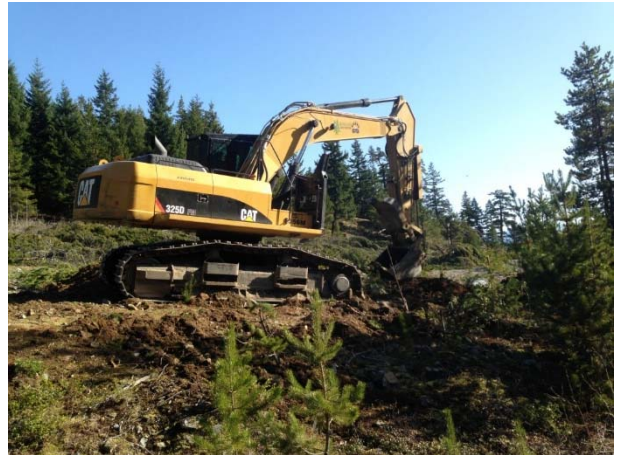
Photo 10 – Spur road construction in segment 16 (April 9, 2015).
