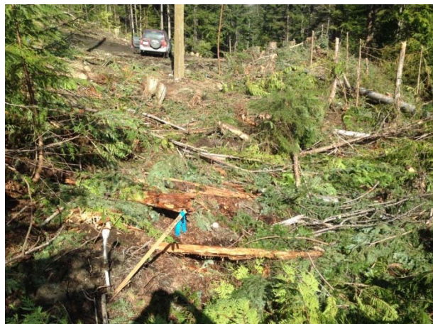
Photo 13 – RVMA near structure 193 following completion of works, anchor in foreground (April 9, 2015).
