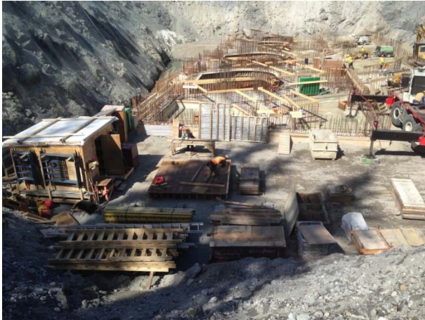
Photo 1 – Formwork installation at ULRHEF powerhouse (April 8, 2015).
