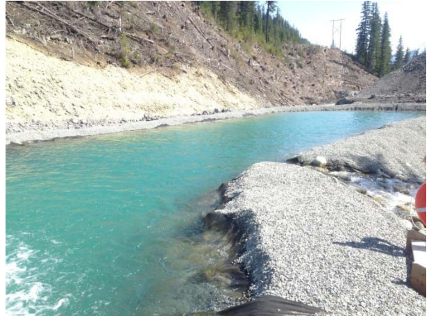
Photo 2 – Current condition of ULRHEF settling ponds (April 8, 2015).
