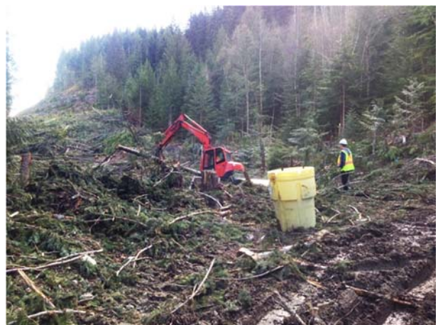
Photo 12 – Machine works in RVMA near pole 193, spill kit onsite (April 7, 2015).
