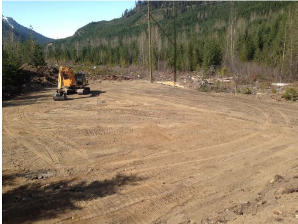
Photo 7 – Levelling of temporary generator site in Segment 1 (April 8, 2015).
