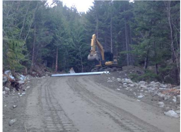
Photo 8 - Dry culvert installation on road 197.2 (April 8, 2015).
