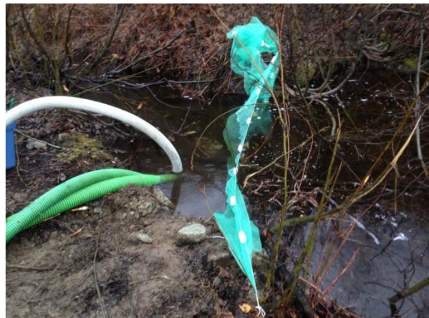
Photo 12 – Three pumps used to dewater worksite for MB27 culvert installation (March 30, 2015).
