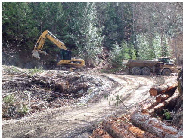
Photo 15 – Road works on road 197.2 above Black's Bridge (April 1, 2015).
