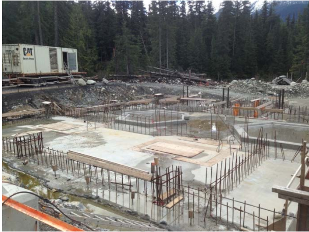
Photo 7 – Current conditions at BDRHEF powerhouse (April 1, 2015).
