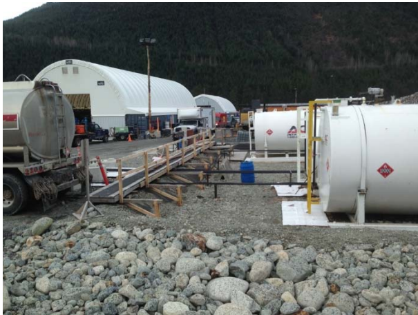
Photo 1 – Fuel storage area at 38KM laydown (April 1, 2015).
