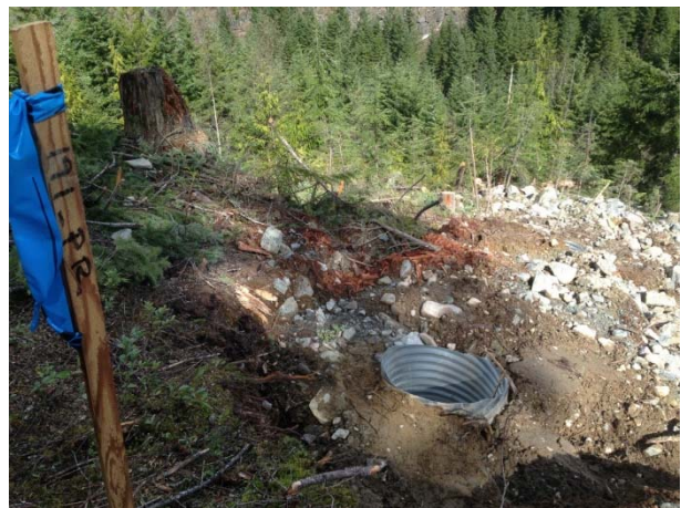
Photo 16 – Groundworks completed for pole installation at structure 191 in Segment 8 (April 1, 2015).
