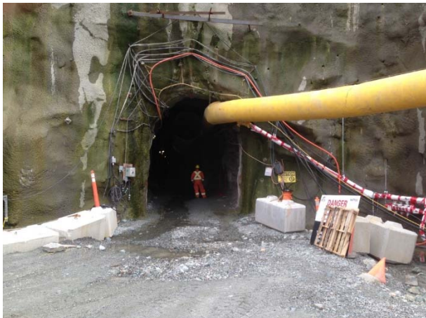
Photo 9 – Preparation for hydraulic jacking at the BDRHEF downstream tunnel portal (April 1, 2015).
