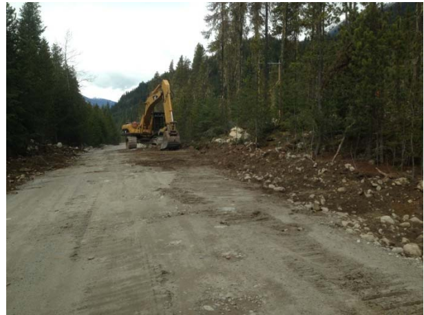
Photo 2 – Road maintenance on Lillooet River FSR near 19km (April 1, 2015).
