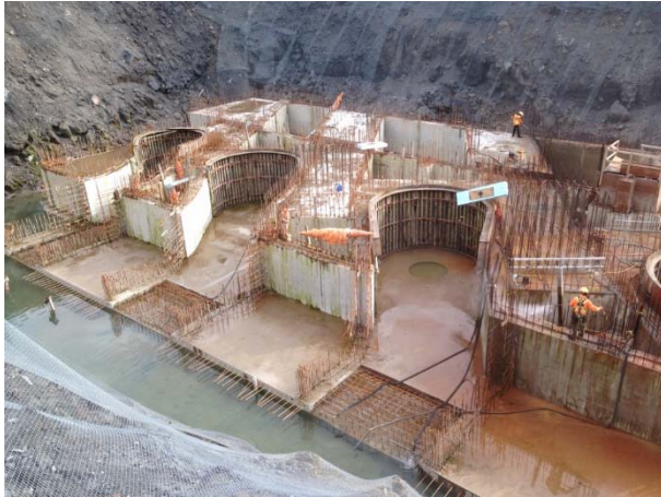
Photo 3 – Looking northeast at ULRHEF powerhouse (April 1, 2015).
