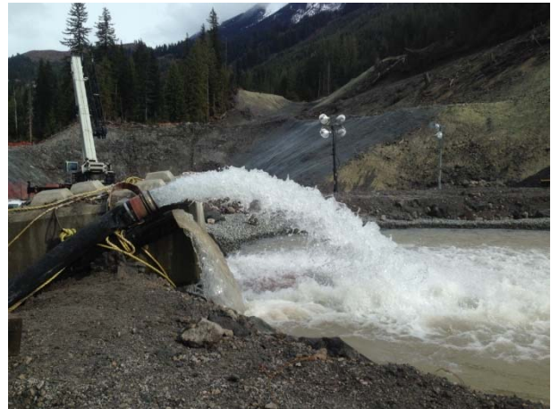
Photo 6 – ULRHEF powerhouse discharge to settling ponds following French drain excavation (April 1, 2015).
