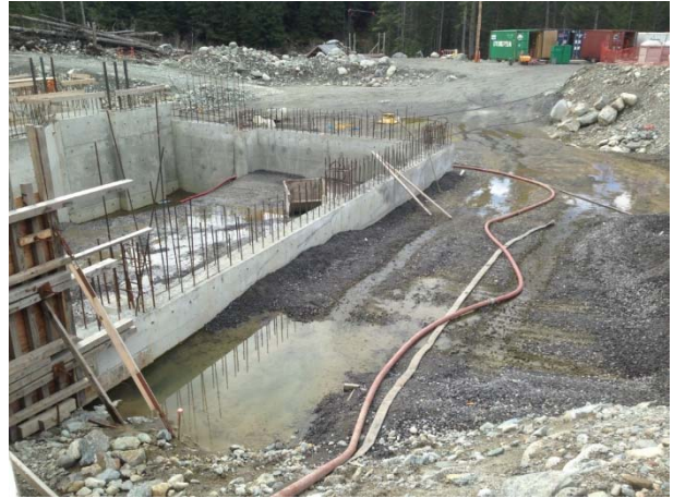
Photo 8 – BDRHEF powerhouse dewatering directed to settling ponds (April 1, 2015).
