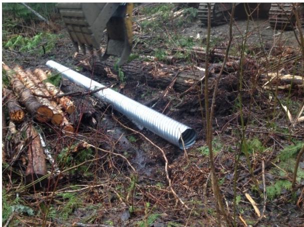
Photo 12 – Culvert installed at spur 184.1 off of road 197.2 (March 26, 2015).
