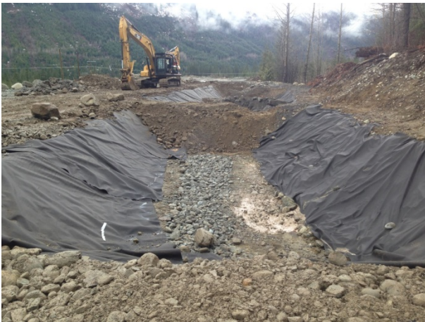
Photo 5 – Reconstruction of BDRHEF powerhouse settling ponds (March 26, 2015).
