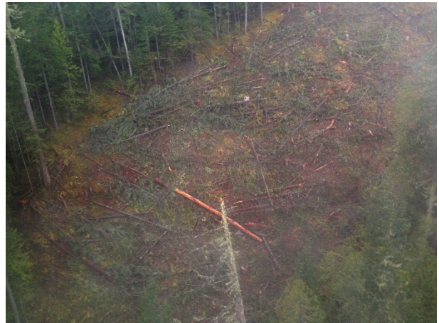
Photo 11 – ROW clearing completed in Segment 9 (March 25, 2015).
