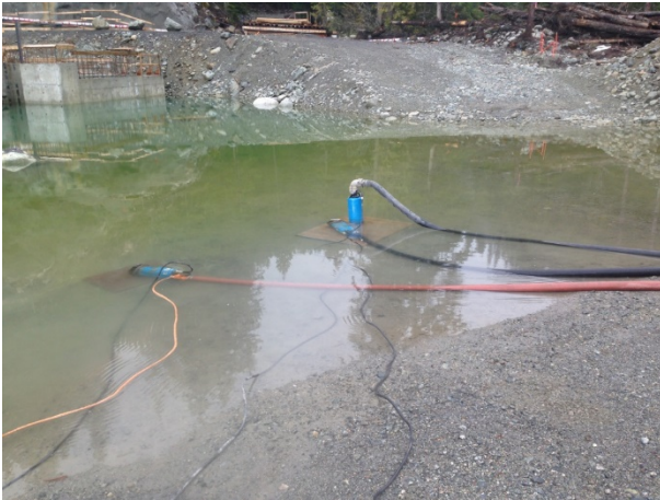
Photo 3 – Three pumps used to dewater BDRHEF powerhouse (March 26, 2015).
