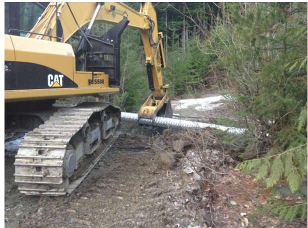
Photo 7 – Culvert installation works at MB47 on the Miller Bench FSR (March 17, 2015).
