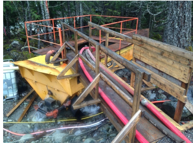
Photo 4 – BDRHEF powerhouse water conveyed to container for sediment detention (March 26, 2015).
