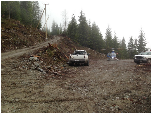
Photo 10 – Segment 9 staging area at end of Salmon Main (March 25, 2015).
