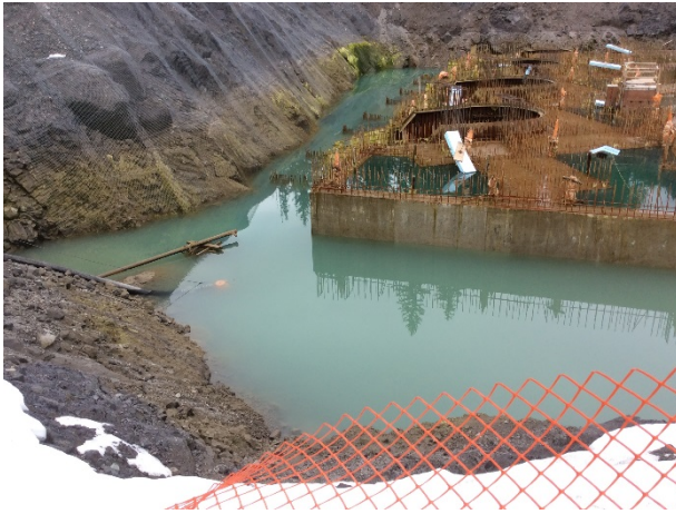
Photo 1 – 10” hose leading out of ULRHEF powerhouse for dewatering (March 27, 2015).
