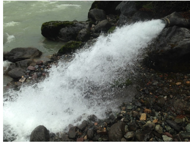
Photo 2 – Outlet of 10” hose used for dewatering ULRHEF powerhouse (March 26, 2015).
