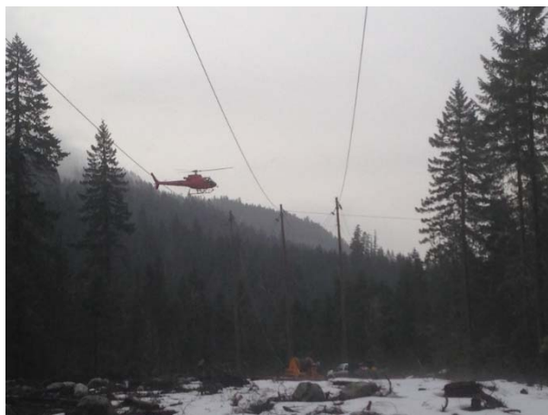
Photo 10 – A-Star B3 helicopter flying pilot line at pole 136 (March 11, 2015).
