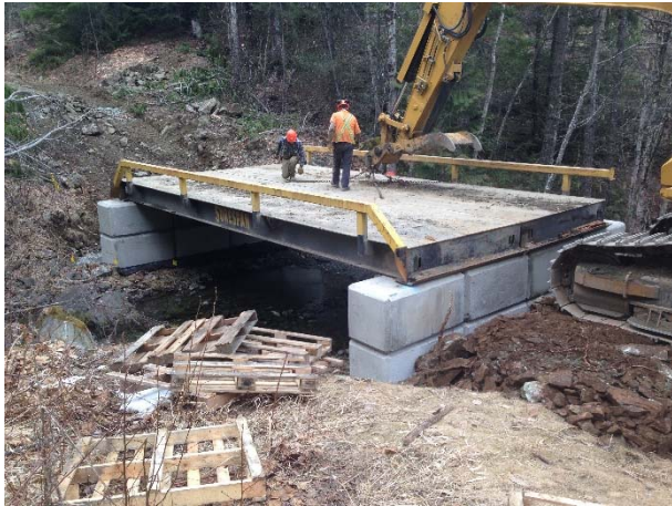
Photo 7 – Bridge installation works at MB53 on the Miller Bench FSR (March 6, 2015).
