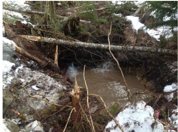
Photo 4 – Sump excavated to allow water to be pumped for worksite isolation during culvert installation at 1+335 on road 197.2 (March 4, 2015).
