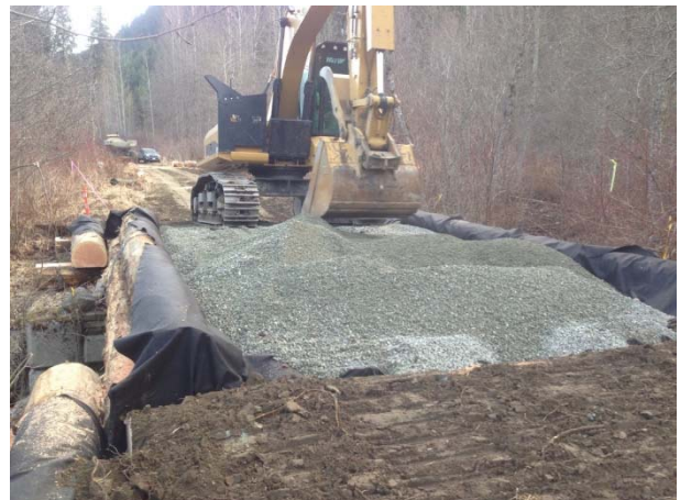
Photo 6 – Bridge installation works at MB59 on the Miller Bench FSR (March 3, 2015).
