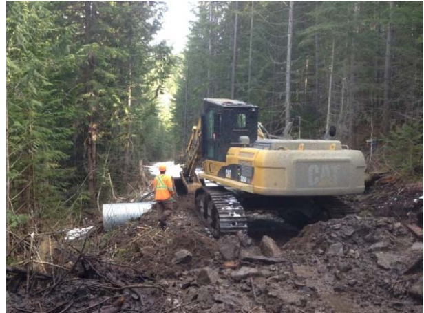
Photo 2 – Culvert installation works at 1+911 on road 197.2 (March 3, 2015).
