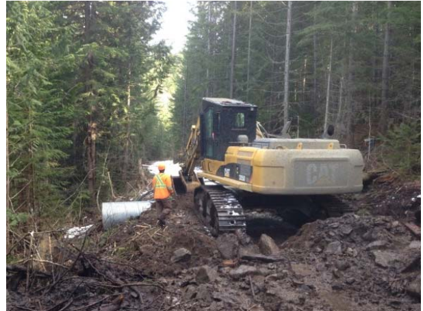
Photo 2 – Culvert installation works at 1+911 on road 197.2 (March 3, 2015).
