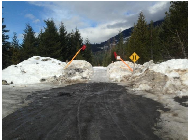
Photo 2 – Transition into winter work area at 38.5km (February 26, 2015).
