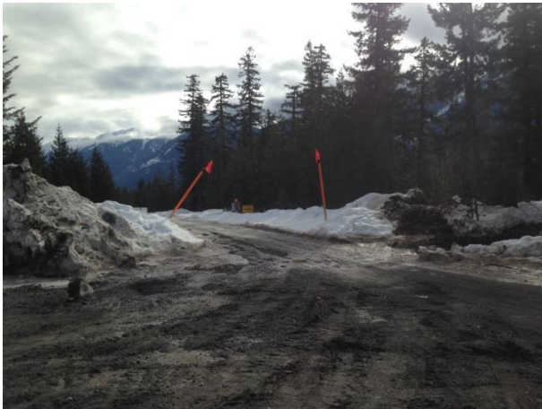
Photo 1 – Transition into winter work area at 37.5km (February 26, 2015).
