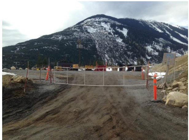
Photo 4 – The electric fence was operational and snow free during the February 26, 2015 inspection.
