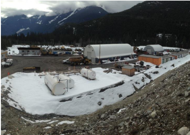
Photo 5 – Conditions at fuel storage area within Pad 2 of the 38km laydown (February 26, 2015).
