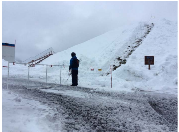
Photo 4 – The electric fence was operational and snow free during the January 23, 2015 inspection.
