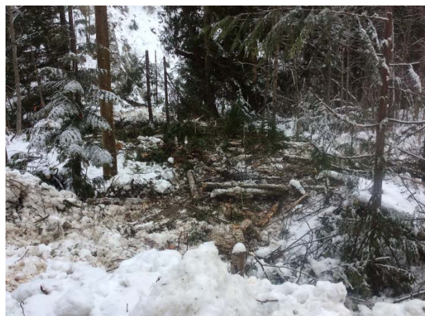
Photo 10 – Conditions following the operation of an excavator with 30m of the Salmon Slough (January 22, 2015).
