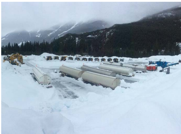
Photo 5 – Conditions at fuel storage area within Pad 1 of the 38km laydown (January 23, 2015).
