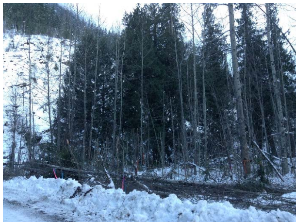
Photo 7 – Hand falling near pole 5 of the Stringer Line alignment (January 13, 2015).
