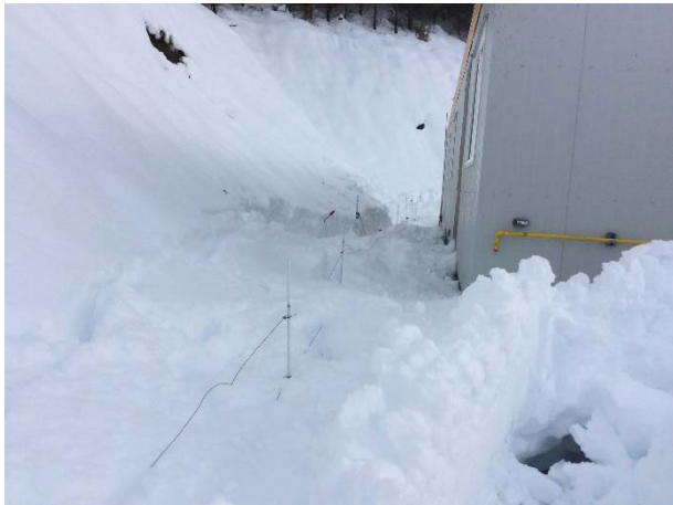
Photo 3 – The electric fence was being repaired and cleared of snow during the January 9, 2015 inspection.
