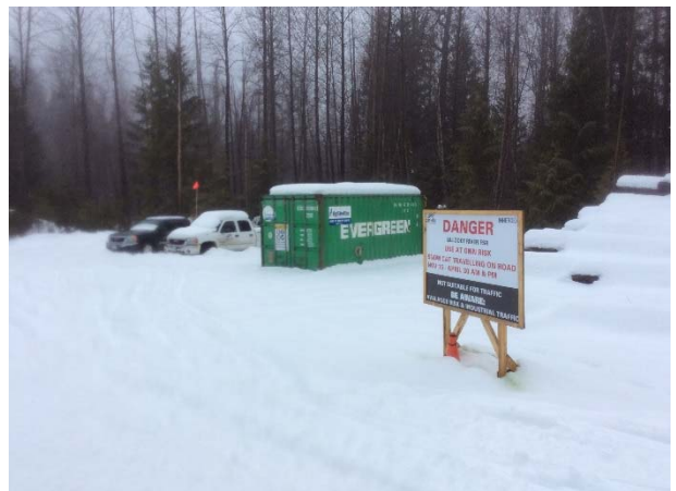
Photo 6 – Example of sign boards posted to warn public of the dangers of entering closed construction areas (January 23, 2015).
