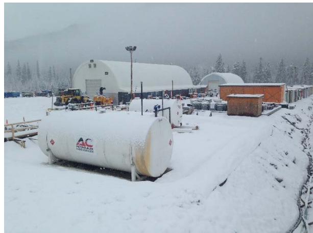
Photo 2 – Conditions at fuel storage area at the 39 km laydown (December 18, 2014).
