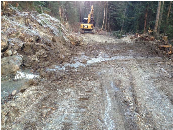
Photo 4 – Segment 8 crossing ditching above Hillaby Creek (December 15, 2014).
