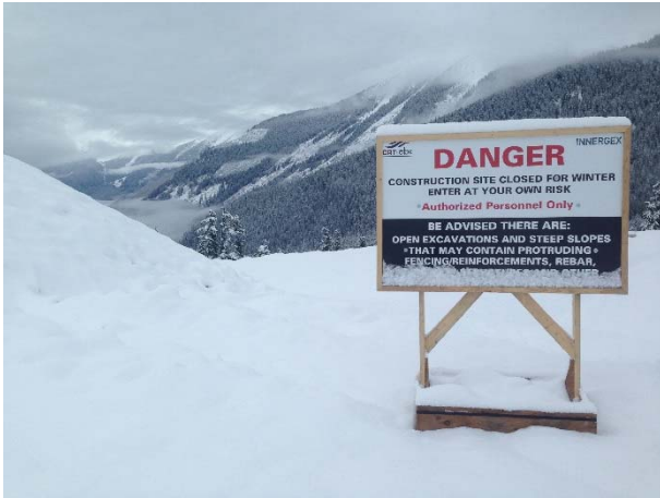
Photo 3 – Example of sign boards posted at all closed construction areas (December 18, 2014).
