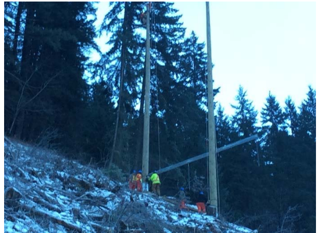
Photo 5 – Segment 5 pole dressing works (December 2, 2014).
