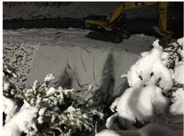
Photo 4 – Installing geotextile on the downstream face of the cofferdam (November 24, 2014).
