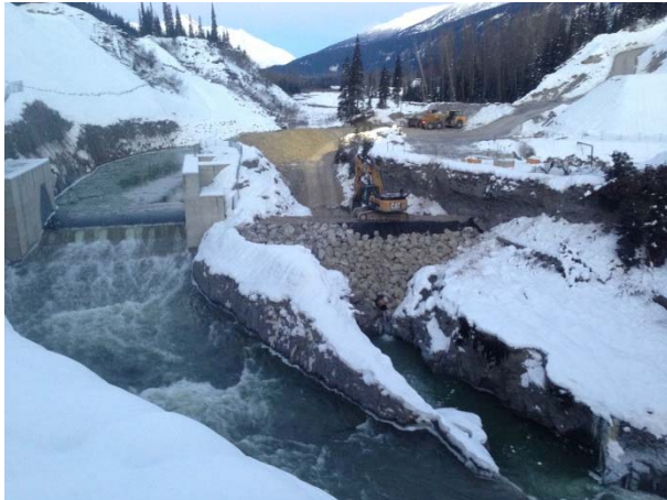
Photo 11 – Final riprap armoring of the downstream cofferdam (November 29, 2014)
