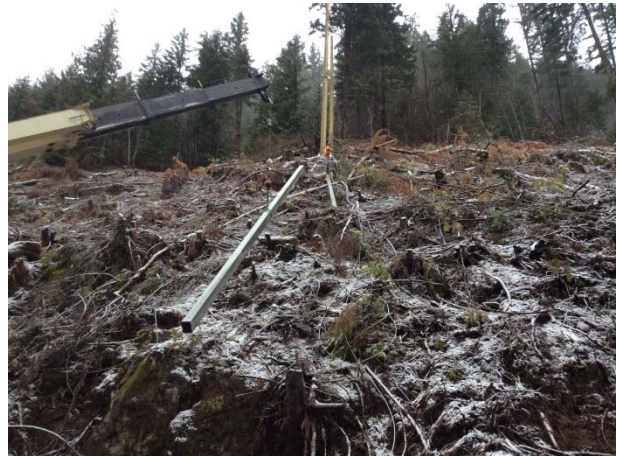
Photo 19 – Segment 5 pole dressing works (November 25, 2014).
