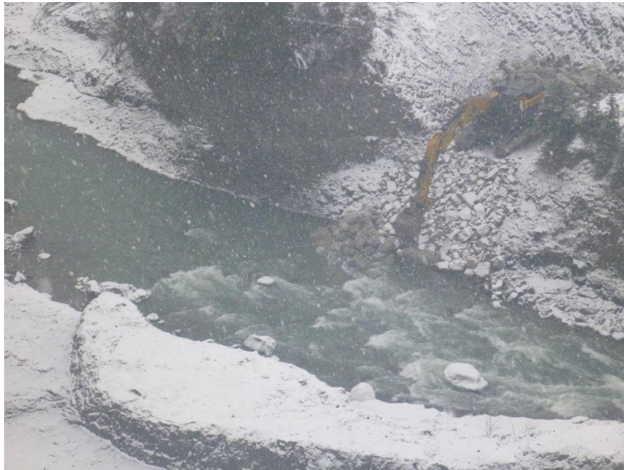
Figure 3. Placement of first rock layer of cofferdam instream.
