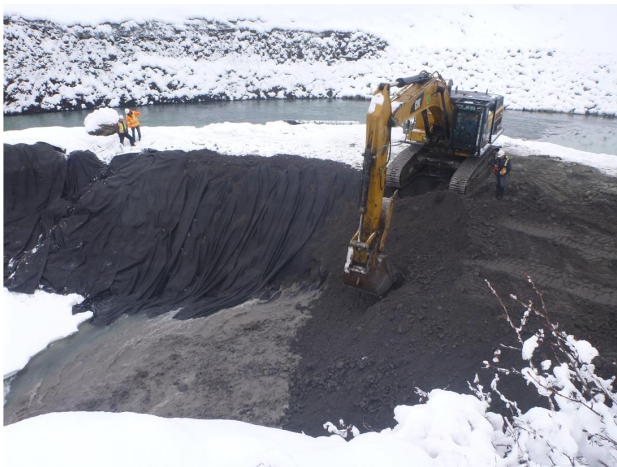
Figure 16. Installation of the fine material backfill began at river left and a full cofferdam width was packed in before proceeding section by section across the channel. The flows through the rock fill resulted in material washing out, elevating turbidity downstream.
