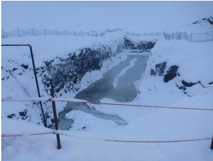
Figure 16. Installation of the fine material backfill began at river left and a full cofferdam width was packed in before proceeding section by section across the channel. The flows through the rock fill resulted in material washing out, elevating turbidity downstream.
