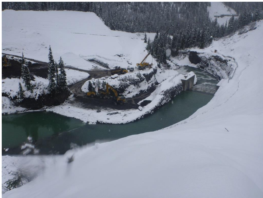
Figure 24. View of the temporary diversion channel from river right. Machinery on river left is working on the newly constructed cofferdam. Flows are entirely diverted and running clear. The clean flow through the temporary diversion had a significant diluting effect on turbid flows where it met with the discharge from the cofferdam works at the downstream end.
