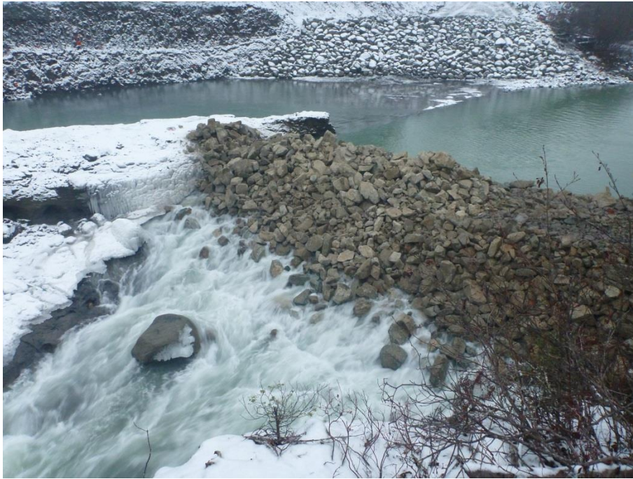
Figure 7. Once the initial flow diversion had taken place, turbidity in the river rapidly reverted to background values below the cofferdam.
