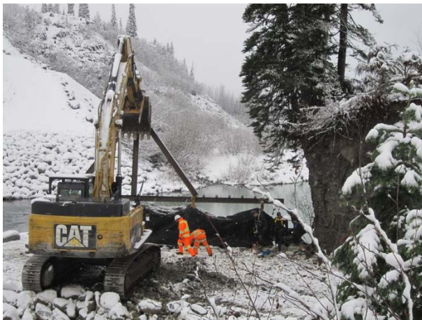
Photo 1 – Continued installation of cofferdam liner to the upstream cofferdam (November 23, 2014)
