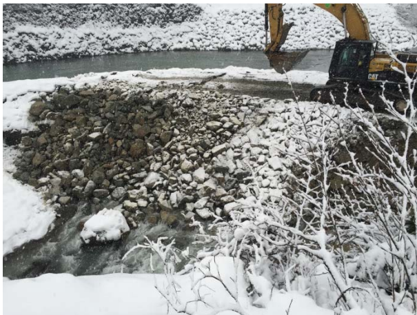
Photo 3 – Reshaping the downstream side of the cofferdam (November 24, 2014).
