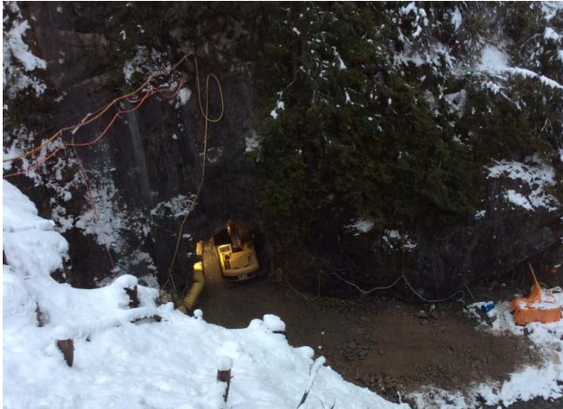
Photo 14 – Excavator completing mucking activities inside the BDRHEF diversion tunnel excavation (November 25, 2014).
