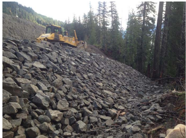
Photo 15 – Stabilization works at 2+800 fill slope (November 9, 2014).
