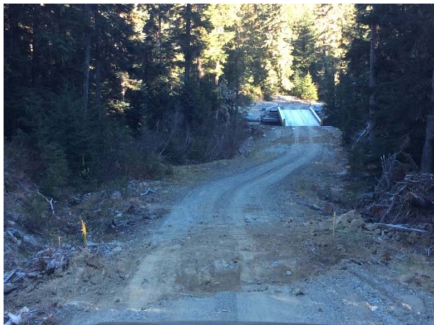
Photo 31 – Road upgrade and winterization works on road 371.1 (November 13, 2014).
