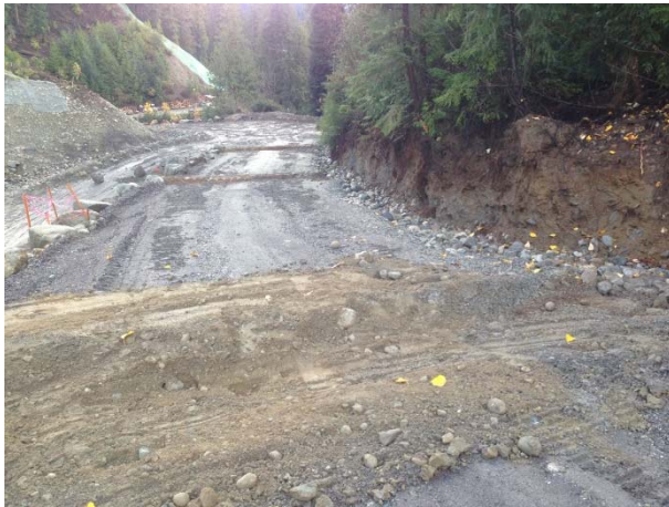
Photo 11 – Cross ditching on ULRHEF access road (November 9, 2014).
