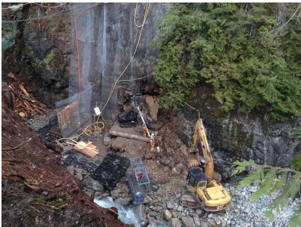
Photo 25– BDRHEF intake diversion tunnelling works (November 9, 2014).
