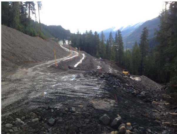
Photo 14 – Re-grading and rock armouring works at 2+800 fill slope (November 9, 2014).
