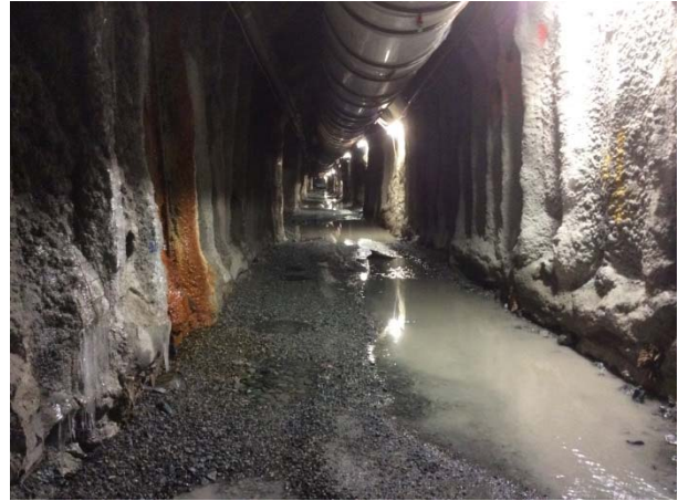
Photo 29– Current conditions in BDRHEF downstream portal tunnel (November 15, 2014).
