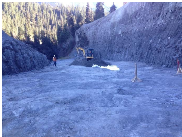
Photo 5 – Cleaning of downstream end of ULRHEF intake diversion channel (November 10, 2014).
