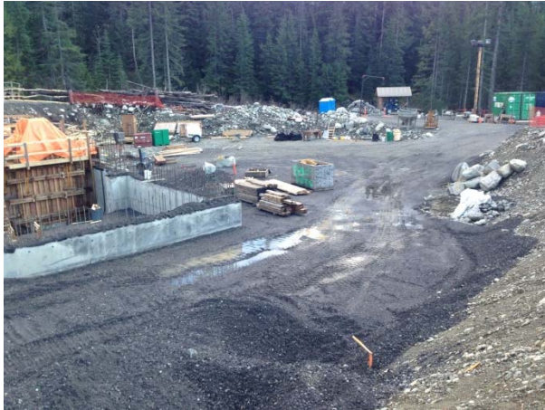
Photo 28 – BDRHEF powerhouse following backfill works (November 9, 2014).
