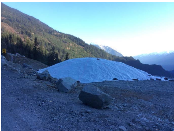
Photo 13– PAG stockpile covered with tarp at KM 44.5 on Lillooet River FSR (November 14, 2014).
