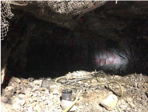
Photo 27 – Conditions inside BDRHEF intake diversion tunnel (November 11, 2014).
