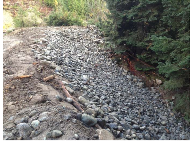
Photo 10 – Re-grading and armoring of slope at bottom of access road (November 9, 2014)
