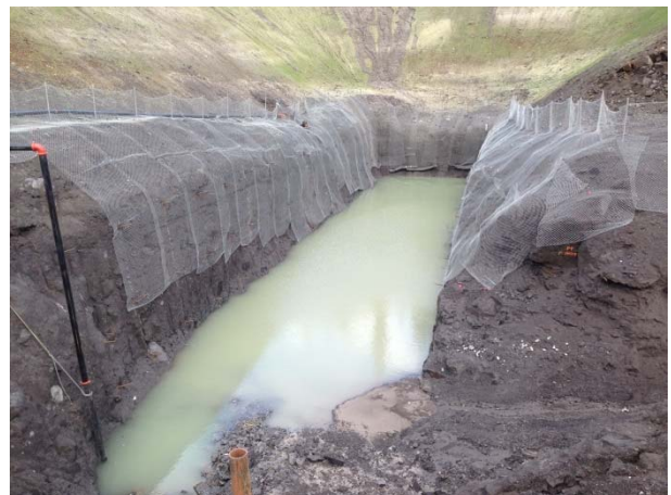
Photo 6 – Current conditions at ULRHEF upstream tunnel portal excavation (November 9, 2014).
