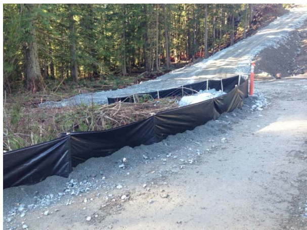
Photo 20 – Silt fencing installed around ASTR04 (November 10, 2014).
