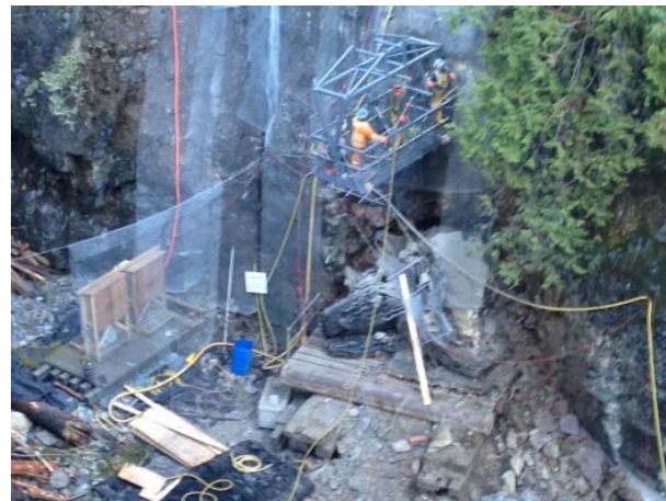
Photo 26– Stabilization works above BDRHEF intake diversion tunnel (November 10, 2014).
