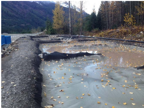
Photo 30– Current conditions at BDRHEF portal settling ponds (November 9, 2014).
