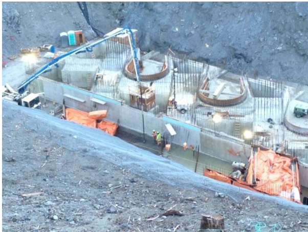
Photo 21 – Continued concrete works at ULRHEF powerhouse (November 12, 2014).
