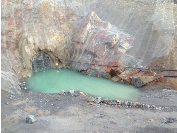
Photo 9 – Conditions at ULRHEF downstream tunnel portal (November 9, 2014)
