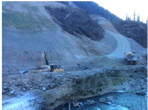
Photo 4 – Excavation for upstream end of ULRHEF intake diversion channel (November 15, 2014).
