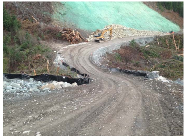
Photo 19 – Silt fencing installed around ASTR03 (November 10, 2014).
