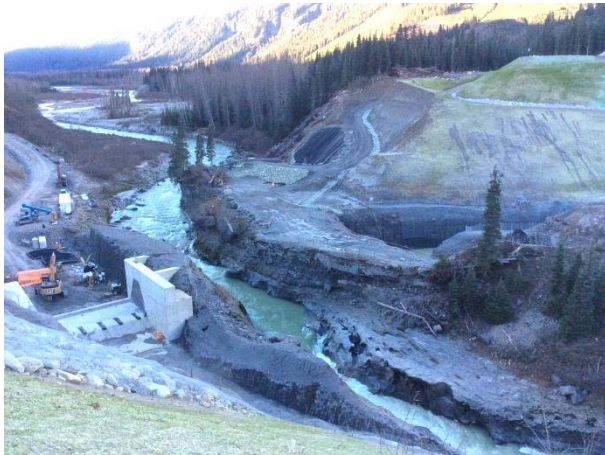
Photo 1 – Current conditions at ULRHEF intake (November 10, 2014).
