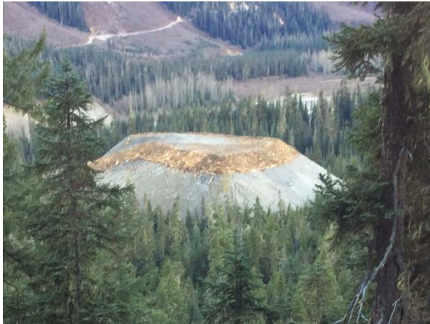
Photo 7 – Woody debris and organic material placed on top of north side spoil pile slopes (November 10, 2014).
