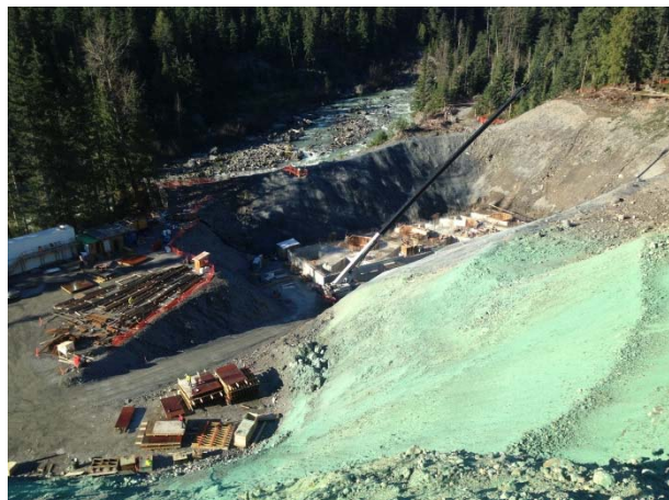
Photo 23 – Hydroseeding completed on slope above ULRHEF powerhouse (November 11, 2014).
