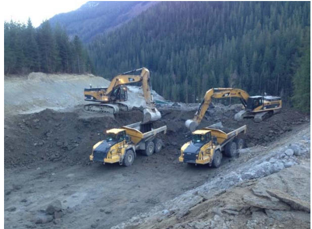
Photo 17 – Bulk excavation at 4+000 (November 12, 2014).
