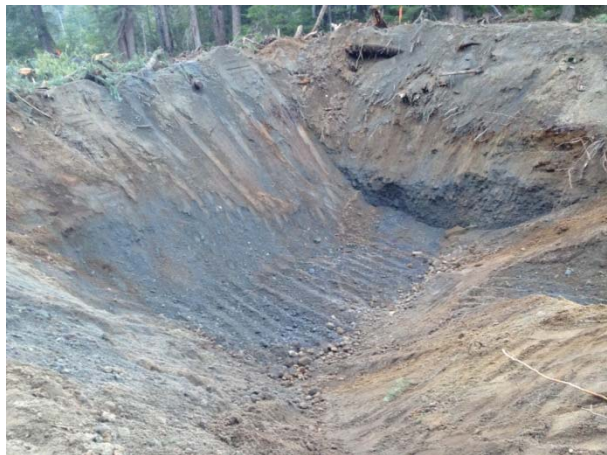
Photo 18 – Sediment basin at drain #6 near station 3+875 (November 12, 2014).
