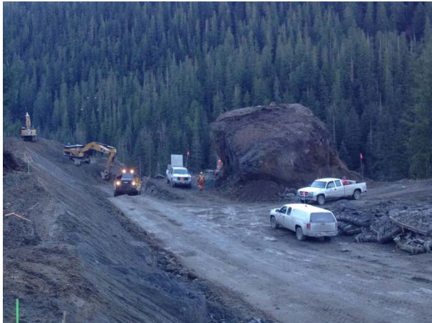
Photo 16 – Bulk excavation and preparation for blasting works at 4+000 (November 11, 2014).
