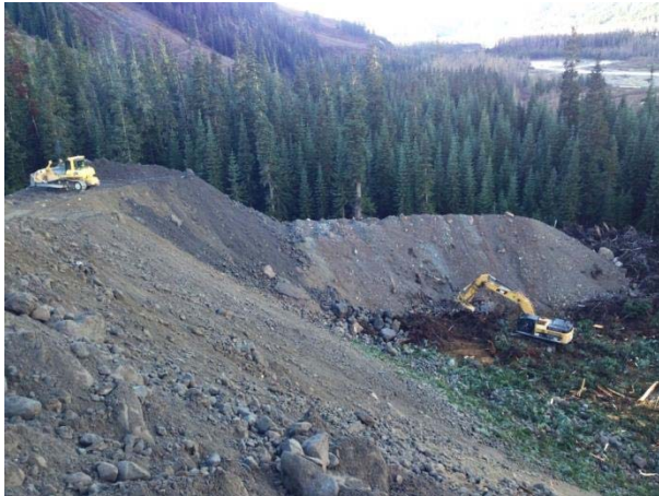
Photo 5 – Re-contouring of south side spoil piles (November 7, 2014).
