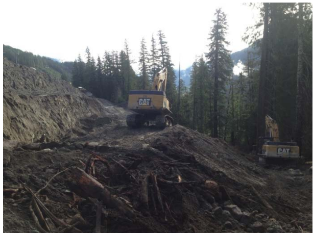
Photo 20 – Stabilization works at 2+800 fill slope (November 7, 2014).
