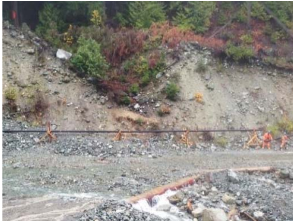
Photo 13 – Dismantling of downstream portal dewatering system (November 3, 2014).
