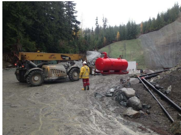
Photo 12 – Crews demobilizing tunnelling equipment (November 3, 2014)
