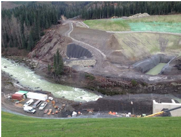
Photo 1 – Current conditions at ULRHEF intake (November 8, 2014).
