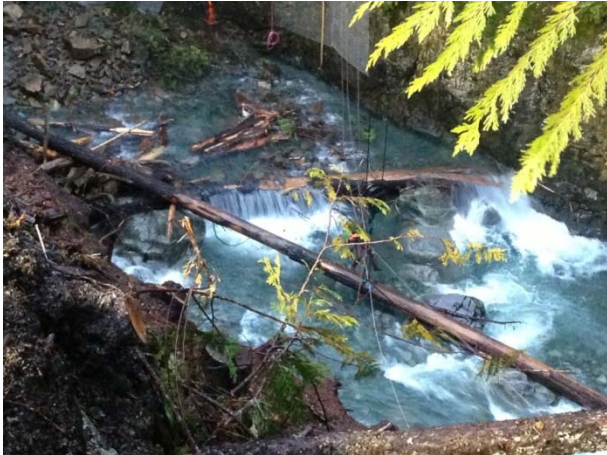
Photo 27 – Rope access crews choke log for crane removal (November 3, 2014).
