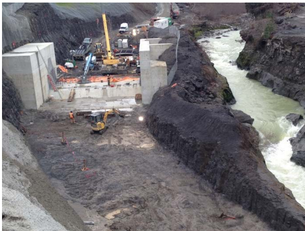
Photo 3 – ULRHEF intake diversion channel cleaning (November 6, 2014).
