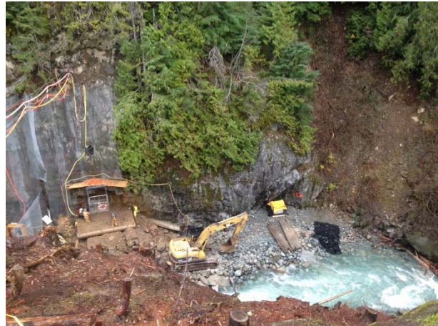
Photo 34 – Conditions at BDRHEF intake diversion tunnel following first blast (November 8, 2014).
