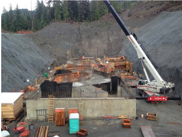
Photo 23 – Current conditions at ULRHEF powerhouse (November 7, 2014).
