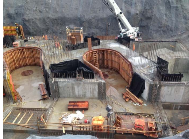
Photo 24 – Current conditions at ULRHEF powerhouse (November 7, 2014).
