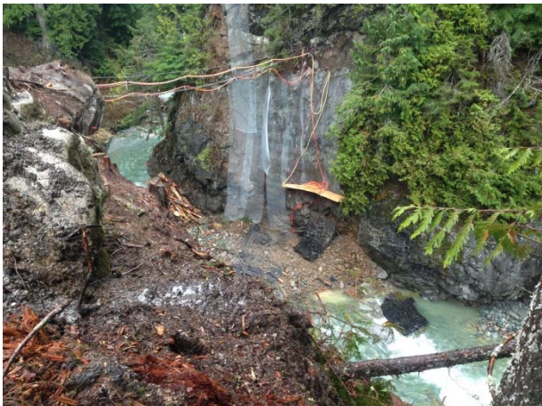
Photo 31 – Blast mat hung during diversion tunnel platform preparation blast (November 5, 2014).
