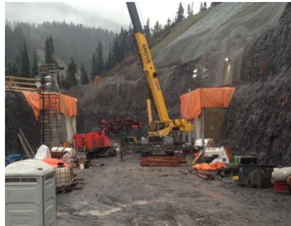
Photo 2 – Current conditions in the ULRHEF intake diversion channel (November 8, 2014).
