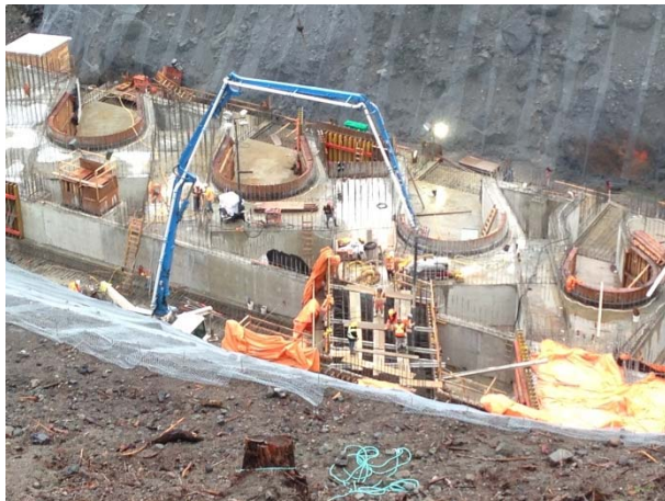
Photo 25 – Continued concrete works at ULRHEF powerhouse (November 8, 2014).
