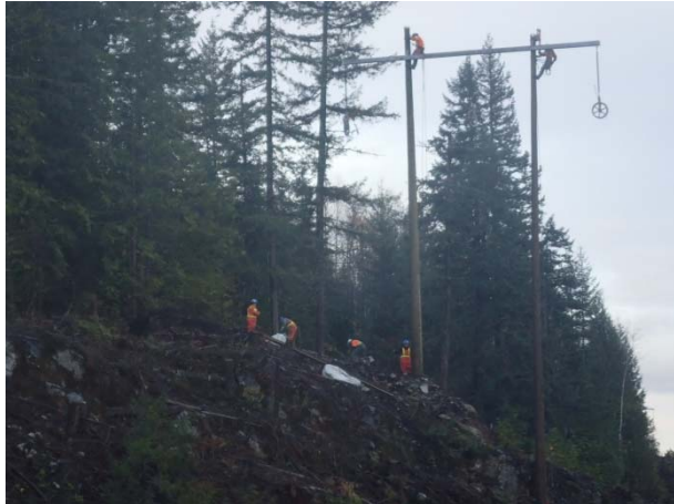
Photo 42 – Segment 5 pole stringing (November 7, 2014)
