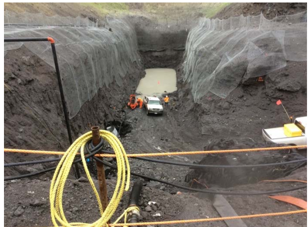
Photo 4 – Demobilization works at the ULRHEF upstream portal excavation (November 4, 2014).
