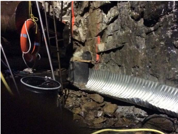
Photo 35 – Half-culvert utilized to convey tunnelling wastewater for containment and disposal (November 6, 2014).
