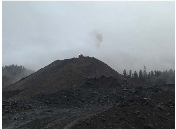
Photo 6 – Bulldozer re-contouring north side spoil pile (November 7, 2014).
