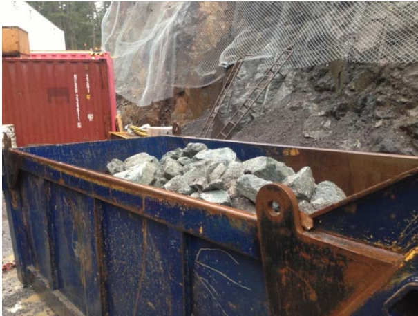
Photo 33 – Clean rock for pad construction at diversion tunnel (November 6, 2014).
