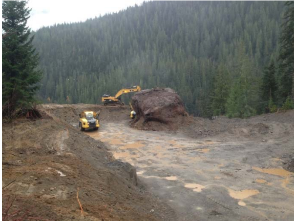
Photo 17 – ULRHEF penstock bulk excavation from station 3+090m – 4+095 (November 3, 2014).
