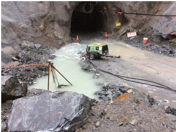
Photo 11 – Conditions at ULRHEF downstream tunnel portal (November 3, 2014)
