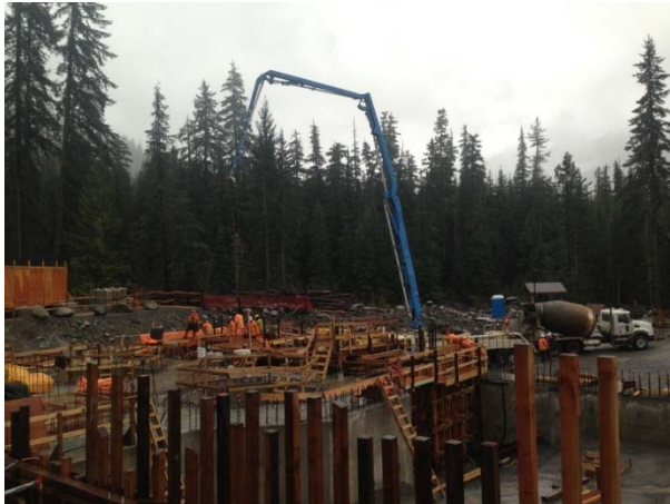
Photo 38 – Concrete works at BDRHEF powerhouse (November 6, 2014).
