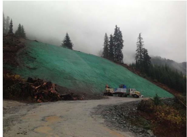
Photo 22 – Hydroseeding slopes near station 3+100 (November 3, 2014).
