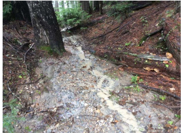
Photo 14 – Mobilizing and deposited sediment observed below downstream portal access road (November 3, 2014).
