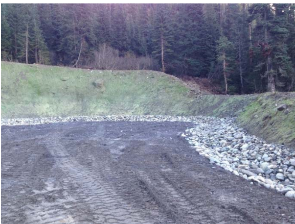
Photo 9 – Re-grading and ditching completed on north side of Keyhole Falls bridge (November 7, 2014).
