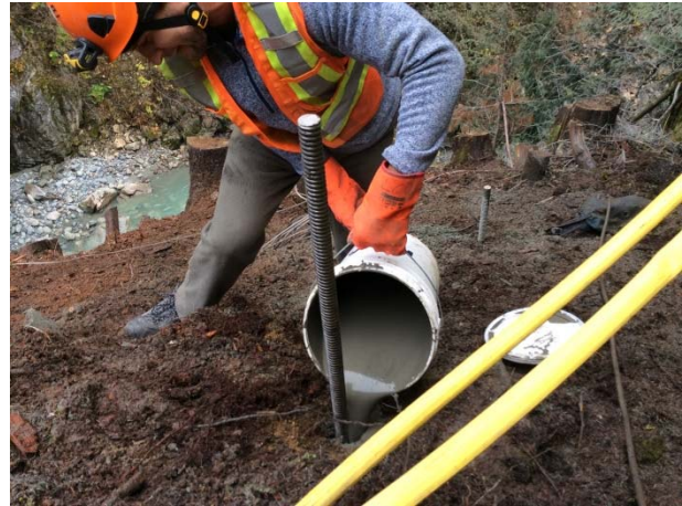
Photo 23 – Grouting anchor bolts for stabilization works (October 27, 2014).
