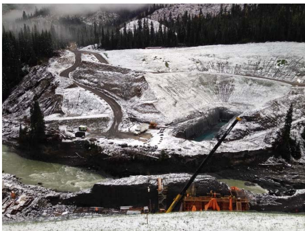
Photo 1 – Current conditions at ULRHEF intake (October 26, 2014).
