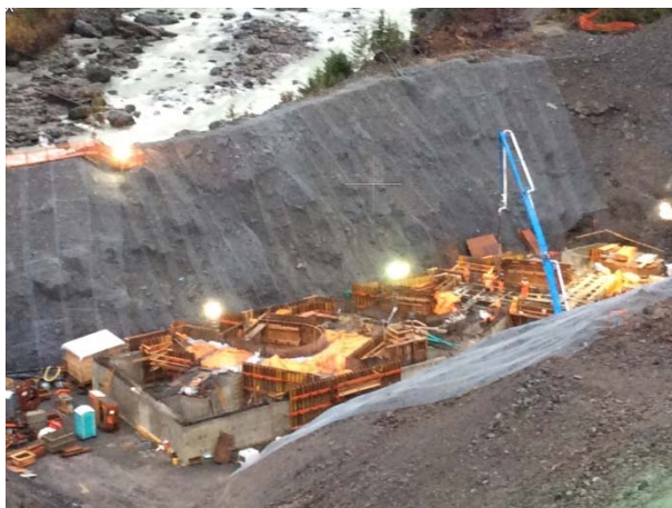
Photo 20 – Current conditions at ULRHEF powerhouse (October 30, 2014).
