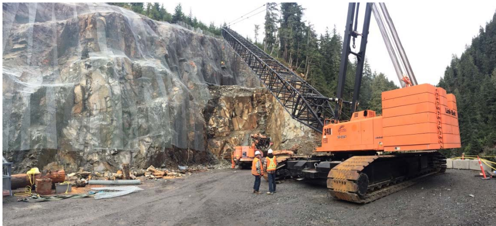
Photo 21 – Slope protection measures at BDRHEF crane pad (October 27, 2014).
