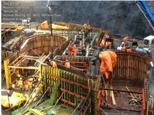
Photo 18 – Continued concrete works at ULRHEF powerhouse (October 30, 2014).
