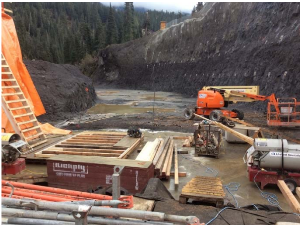
Photo 3 – Current conditions in ULRHEF intake diversion channel (October 27, 2014).
