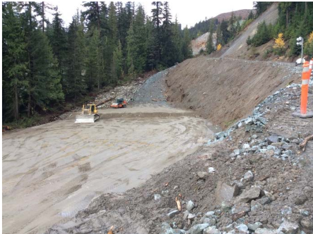
Photo 12 – ULRHEF penstock fill works at station 2+800 (October 26, 2014).
