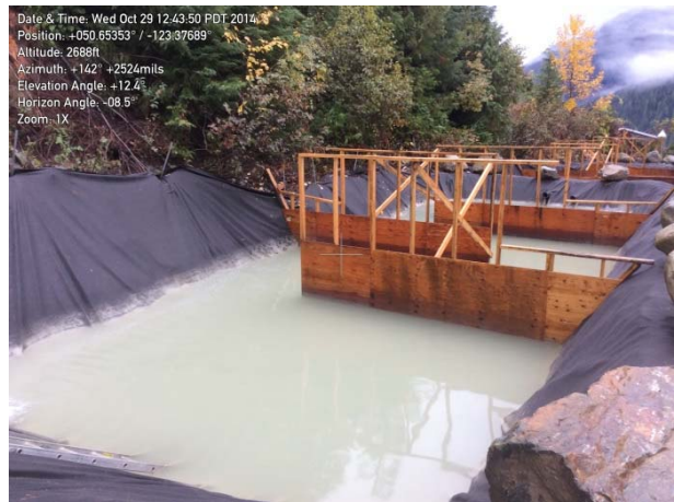
Photo 9 – ULRHEF downstream portal settling ponds (October 29, 2014).
