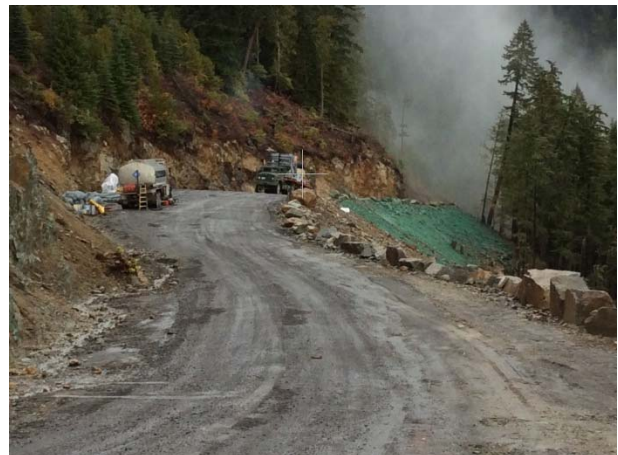
Photo 25 – Hydroseeding on BDRHEF intake access road (October 29, 2014).
