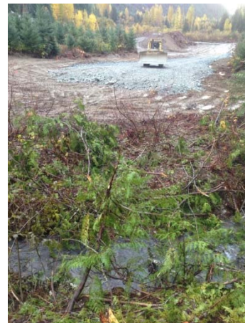
Photo 17–ASTR04 culvert installation site (October 28, 2014).
