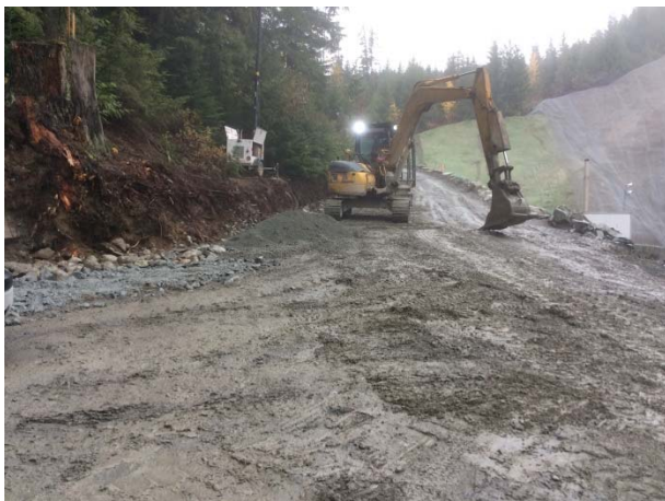
Photo 10 – Ditching works at bottom of ULRHEF downstream portal access road (October 31, 2014).
