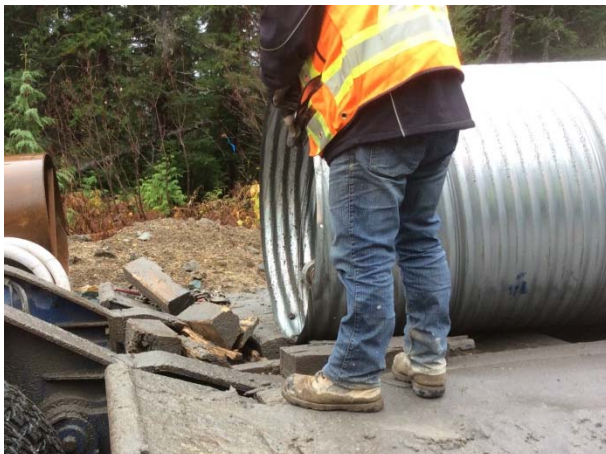
Photo 16– Culvert staged prior to installation at ASTR04 (October 28, 2014).
