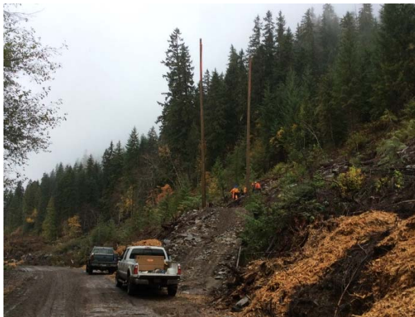
Photo 29 – Setting poles in Segment 4 (October 28, 2014).
