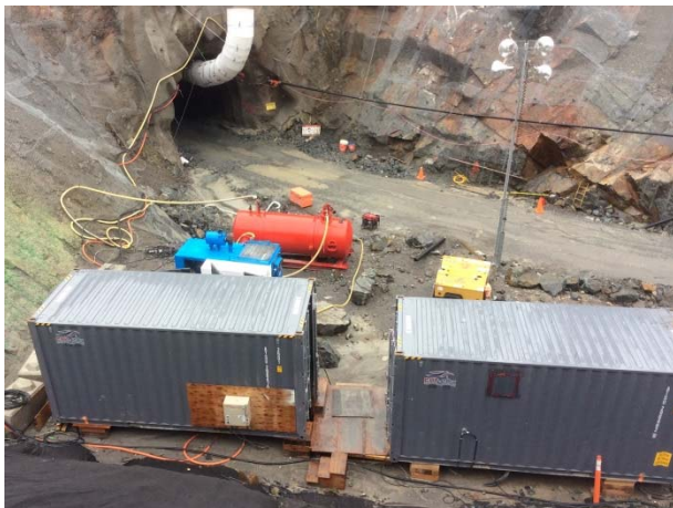
Photo 8 – Current conditions at the ULRHEF downstream tunnel portal (October 31, 2014).
