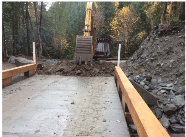
Photo 30 – Segment 8 Black Creek Bridge final approach grading works (October 29, 2014)
