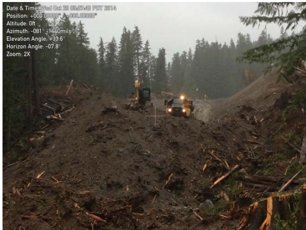
Photo 14 – ULRHEF penstock grubbing and bulk excavation from 2+725 to 3+090m (October 29, 2014).
