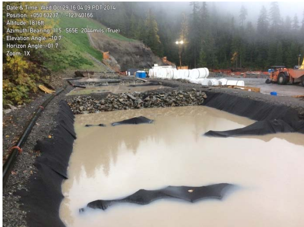
Photo 26 – BDRHEF downstream tunnel portal settling pond (October 29, 2014).
