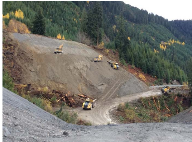
Photo 13 – ULRHEF penstock bulk excavation from station 2+725 to 3+090m (October 26, 2014).
