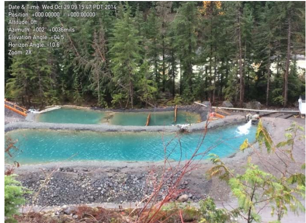
Photo 19 – Current conditions at ULRHEF powerhouse settling ponds (October 29, 2014).
