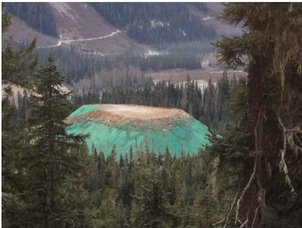
Photo 1 – Re-shaping and hydro-seeding of the north side spoil area at the ULRHEF intake (November 17, 2014).
