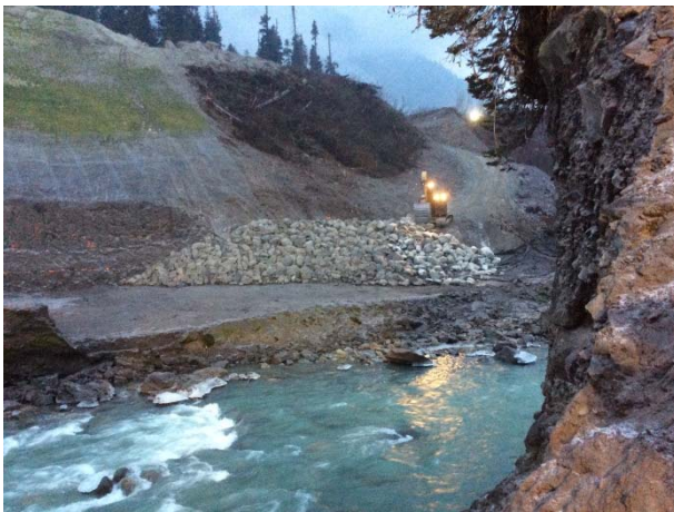
Photo 5 – Armoring of the ULRHEF diversion channel upstream slope (November 20, 2014).
