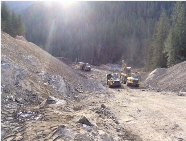
Photo 12 – ULRHEF penstock excavation near station 4+095m (November 17, 2014).
