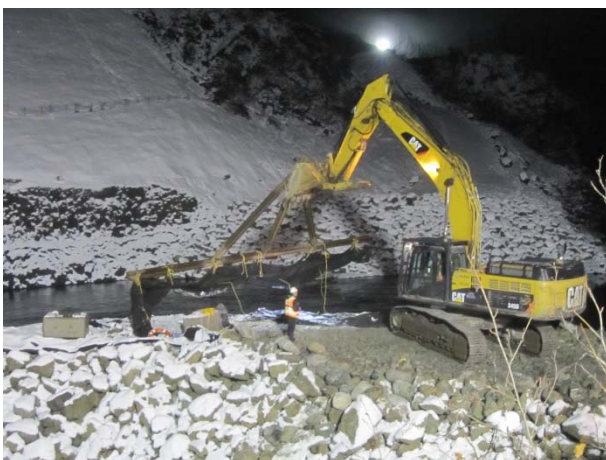
Photo 11 – Excavator modification for placement of the geo-membrane (November 22, 2014).
