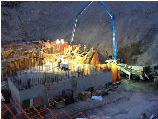
Photo 13 – Structural concrete pour at ULRHEF powerhouse (November 16, 2014).
