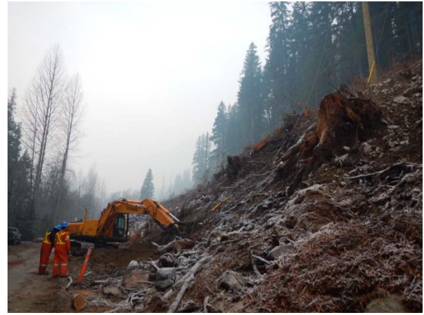
Photo 20 – Segment 5 pole anchor installation (November 18, 2014).
