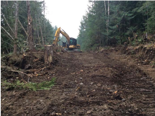
Photo 19 – Segment 8 road construction works November 19, 2014).
