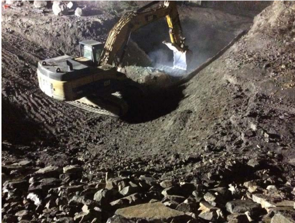
Photo 7 – ULRHEF intake north side cofferdam access ramp excavation (November 18, 2104).
