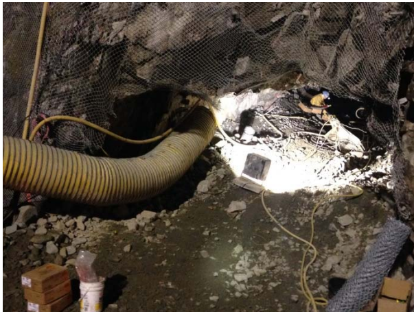
Photo 15 – Conditions inside the BDRHEF diversion tunnel excavation (November 19, 2014).
