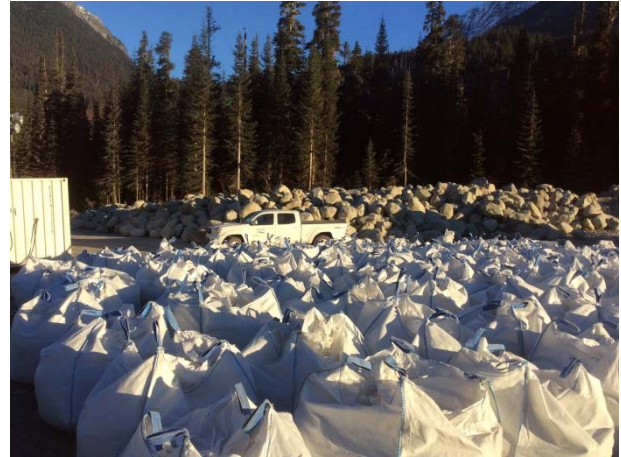
Photo 8 – Stockpiled material near the ULRHEF intake (November 16, 2014).
