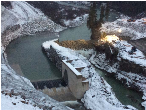
Photo 9 – Washed rock cofferdam and flooding of the diversion channel (November 20, 2014).
