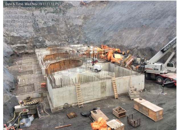
Photo 14 – Continued rebar and formworks at ULRHEF powerhouse (November 19, 2014).
