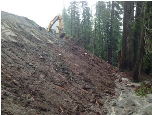
Photo 13 – Fill slope at 2+800 capped with organic material for slope stabilization (October 19, 2014).
