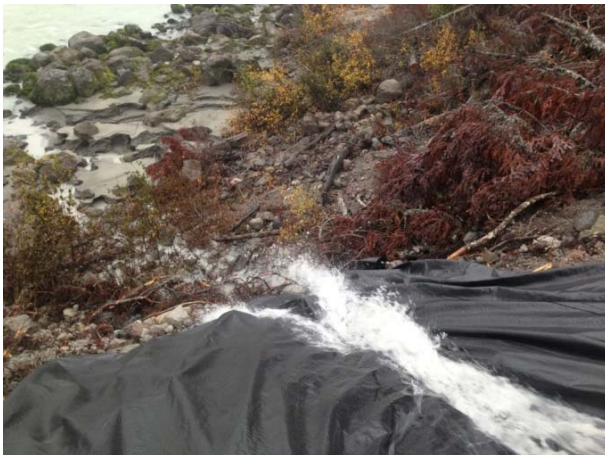
Photo 3 – Turbid water discharging to Upper Lillooet River from north side settling pond spillway (October 19, 2014).
