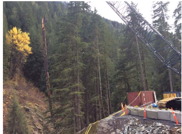
Photo 21 – Log removal at BDRHEF intake using 300 tonne crane (October 24, 2014).
