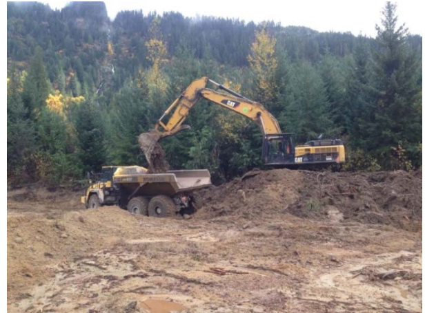
Photo 14 – ULRHEF penstock bulk excavation at 4+075 (October 22, 2014).
