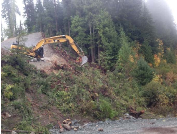
Photo 11 – ULRHEF penstock grubbing and bulk excavation from 2+725 to 3+090m (October 19, 2014).
