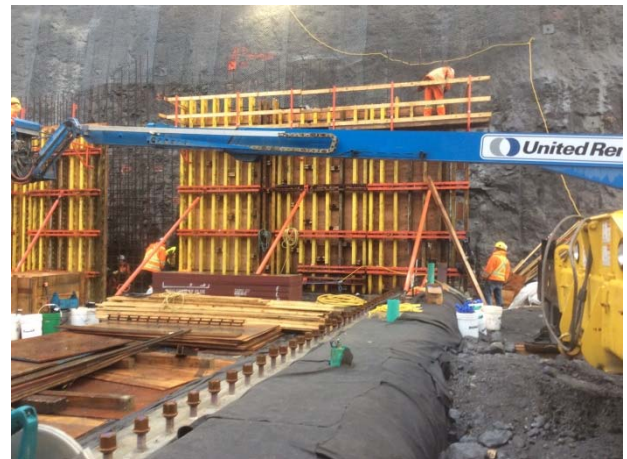
Photo 2 – ULRHEF intake diversion channel Obermeyer weir formworks (October 21, 2014).
