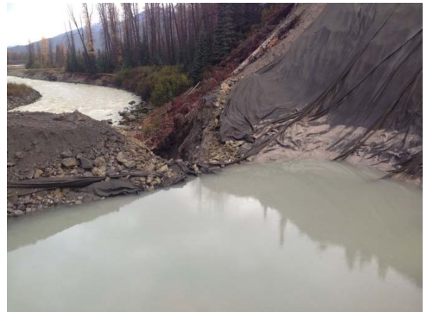
Photo 8 – Second failure at north side settling pond (October 21, 2014).
