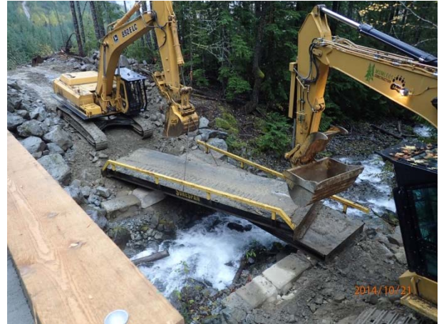
Photo 26 – Removal of temporary bridge over Black's Creek (October 21, 2014).
