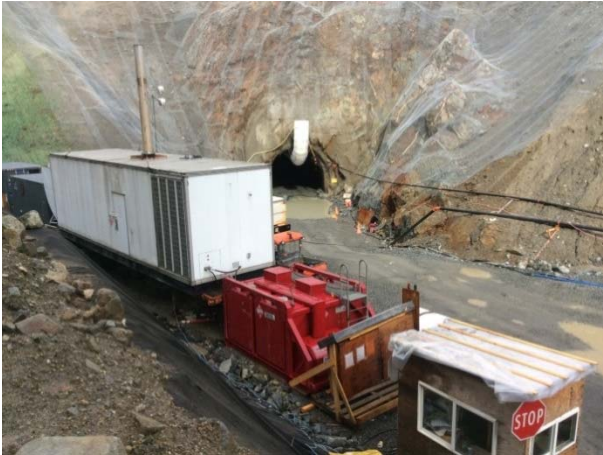
Photo 9 – ULRHEF downstream tunnel portal (October 22, 2014).
