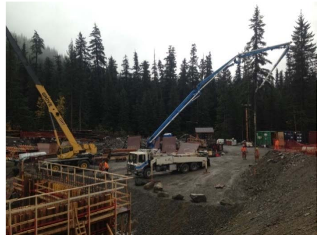
Photo 24 – Concrete works at BDRHEF powerhouse (October 19, 2014).
