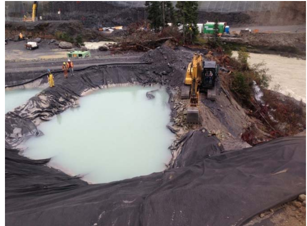
Photo 6 – ULRHEF intake north side settling pond repair works in progress (October 20, 2014).
