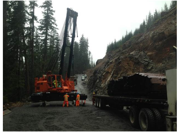
Photo 18 – 300 tonne crane mobilization at BDRHEF intake (October 17, 2014).
