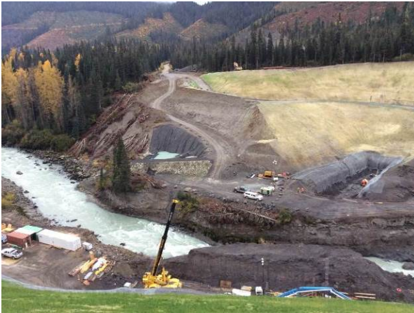
Photo 1 – Overview of the north side of the ULRHEF intake (October 12, 2014).
