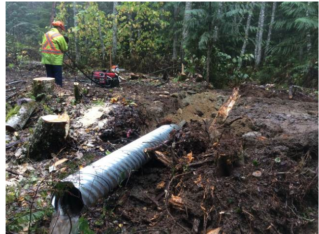
Photo 22 – Segment 8 cross drain culvert installation (October 15, 2014)
