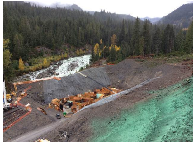
Photo 16 – Current conditions at ULRHEF powerhouse, hydroseeding commenced on upper slopes (October 12, 2014).
