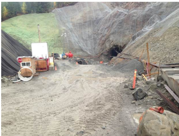
Photo 8 – ULRHEF downstream tunnel portal (October 16, 2014)
