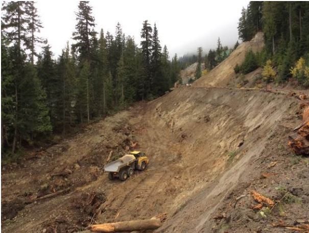
Photo 13 – ULRHEF penstock grubbing and bulk excavation from 2+725 to 3+090m (October 12, 2014).
