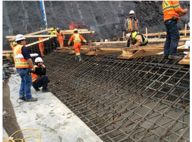
Photo 2 – ULRHEF intake diversion channel, Obermeyer weir formworks (October 12, 2014).
