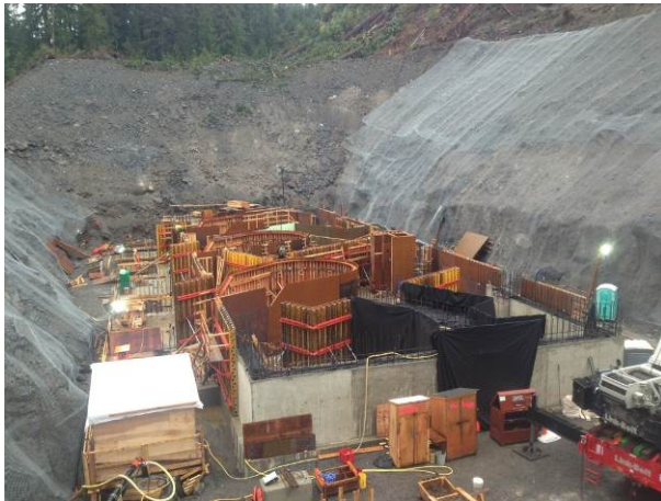
Photo 15 – Continued rebar and formworks at ULRHEF powerhouse (October 3, 2104).
