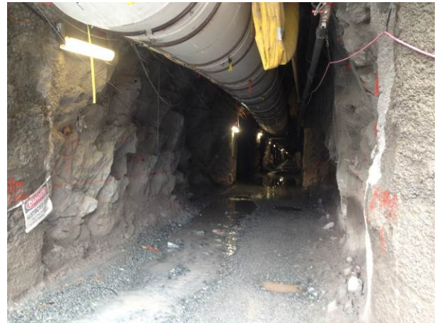
Photo 20 – BDRHEF downstream tunnel portal (October 16, 2014).
