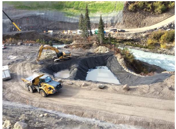
Photo 2 – ULRHEF north side sediment pond (October 10, 2014).
