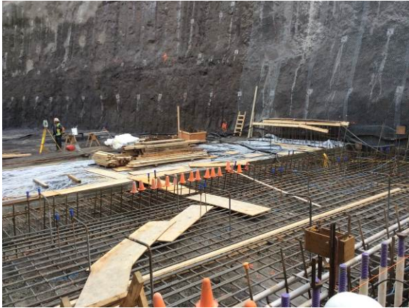
Photo 5 – ULRHEF intake diversion channel, rebar and formworks at Obermeyer weir (October 7, 2014).
