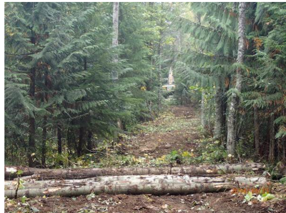
Photo 22 – Segment 8 road upgrading (October 11, 2014)
