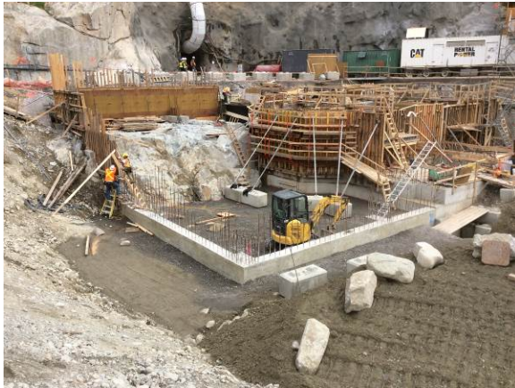
Photo 19 – Current conditions at BDRHEF powerhouse, continued rebar/formworks (October 9, 2014).
