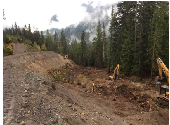
Photo 13 – Stripping and grubbing activities between stations 2+725 to 3+025 (October 11, 2014).
