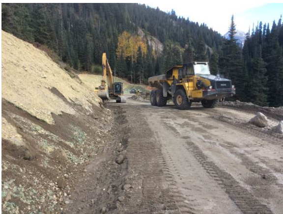
Photo 7 – Ditch improvements along the north side intake access road (October 8, 2014).
