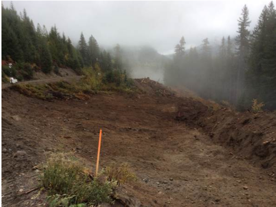
Photo 14 – Stripping and grubbing activities between stations 3+090 to 4+095 (October 11, 2014).
