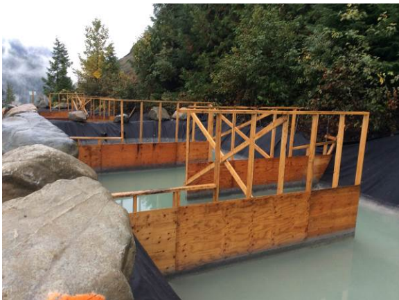
Photo 11 – ULRHEF downstream portal sediment ponds. No discharge was observed (October 11, 2014).
