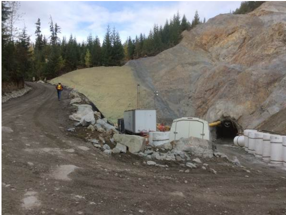
Photo 9 – ULRHEF downstream portal work area (October 9, 2014)
