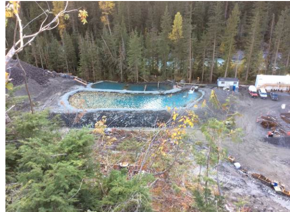
Photo 16 – Condition of the sediment ponds used for ULRHEF powerhouse dewatering (October 8, 2014).
