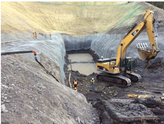
Photo 3 – ULRHEF intake tunnel portal excavation, once seepage was encountered (October 10, 2014).
