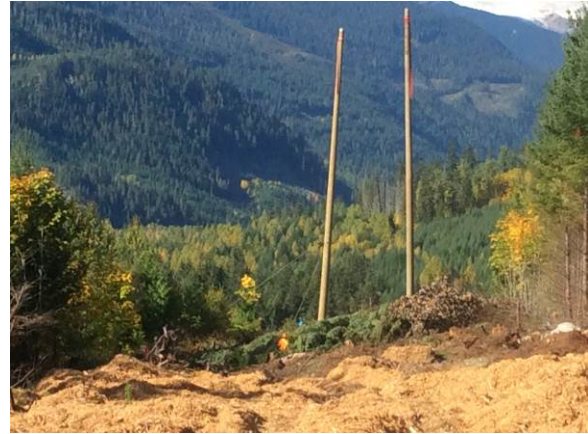
Photo 24 – Segment 4, structure framing works (October 8, 2014).
