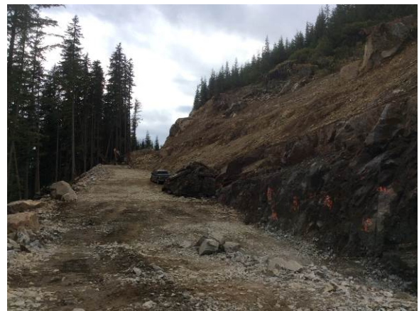
Photo 18 – BDRHEF Intake access road construction (October 9, 2014).
