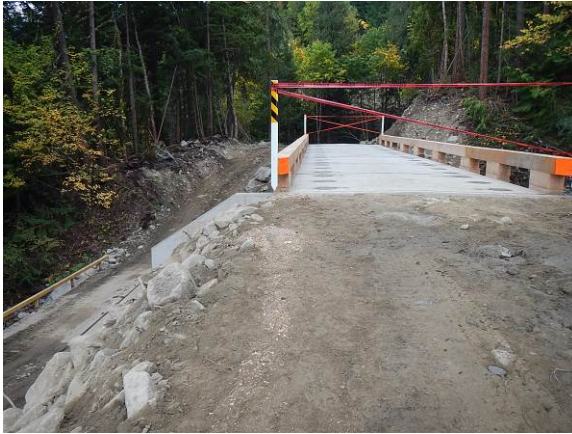
Photo 23 – Segment 8, Black Creek permanent bridge approach final backfill and grading (October 9, 2014).
