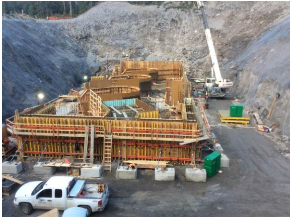
Photo 15 – Current conditions at ULRHEF powerhouse (October 8, 2014).
