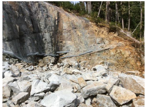
Photo 19 – BDRHEF crane pad wire mesh installation for slope stabilization (October 2, 2014).
