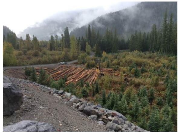
Photo 14 – Yarding and roadside decking at KM 42.5 (October 4, 2014).
