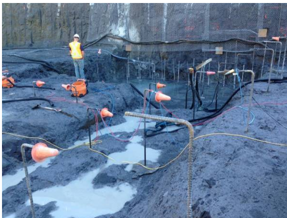
Photo 3 – ULRHEF intake diversion channel, Obermeyer weir anchors (September 28, 2014).
