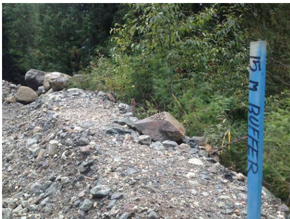
Photo 15 – Surveyed 15m buffer on Truckwash Creek in preparation for ULRHEF penstock clearing (September 28, 2014).
