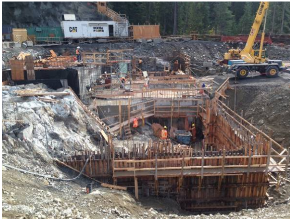
Photo 21 – Current conditions at BDRHEF powerhouse, continued rebar/formworks (September 30, 2014).
