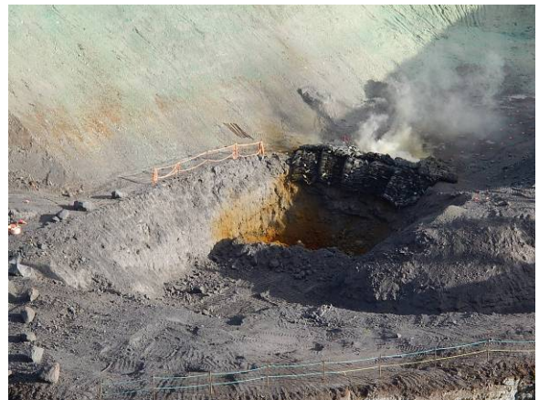
Photo 2 – ULRHEF north side tunnel portal drilling/blasting for tunnel portal (September 30, 2014).
