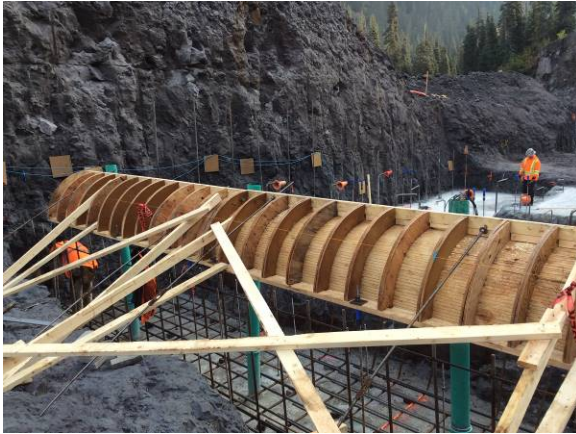
Photo 5 – ULRHEF intake diversion channel, rebar and formworks at Obermeyer weir (October 2, 2104).
