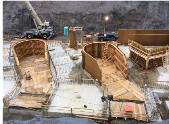
Photo 17 – Continued rebar and formworks at ULRHEF powerhouse (October 3, 2014).
