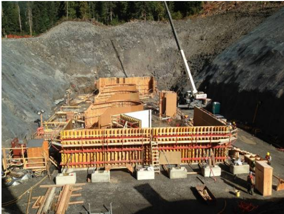
Photo 16 – Current conditions at ULRHEF powerhouse (September 30, 2014).
