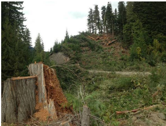
Photo 13 – ULRHEF penstock clearing (October 1, 2014).
