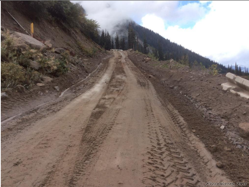
Photo 1. South side access road surface runoff causing erosion must be mitigated. Ditching and check dam installation is recommended.
