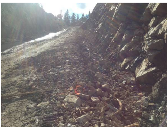
Photo 20 – BDRHEF Intake access road construction including ditching (September 30, 2014).
