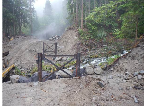
Photo 26 – Segment 8, construction of Black Creek permanent bridge (October 4, 2014).
