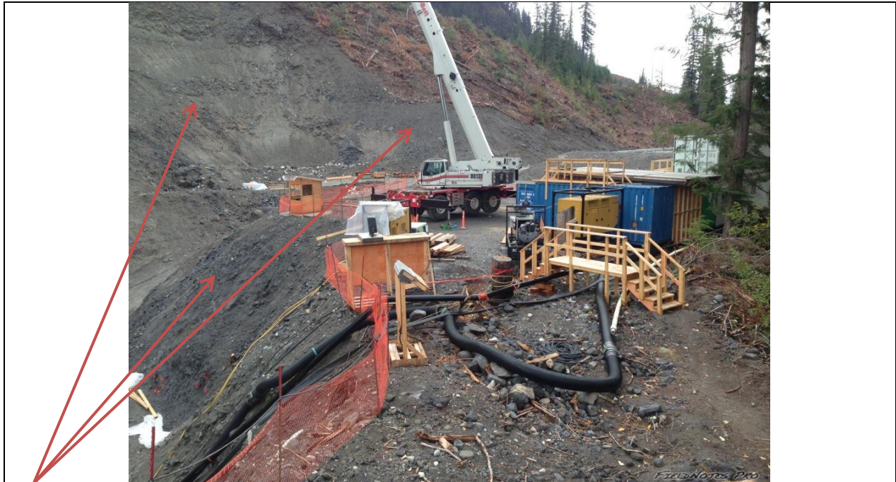
Photo 17. Slope stabilization measures required at the ULRHEF powerhouse cut slopes to protect against erosion. Recommendations include the application of hydro-seed with appropriate mulch product (BFM or FGM) for the upper (final slopes) and covering temporary slopes (below powerhouse backfill elevation) with poly-sheeting.
