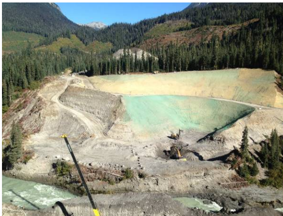
Photo 1 – Overview of the north side of the ULRHEF intake (September 28, 2014).
