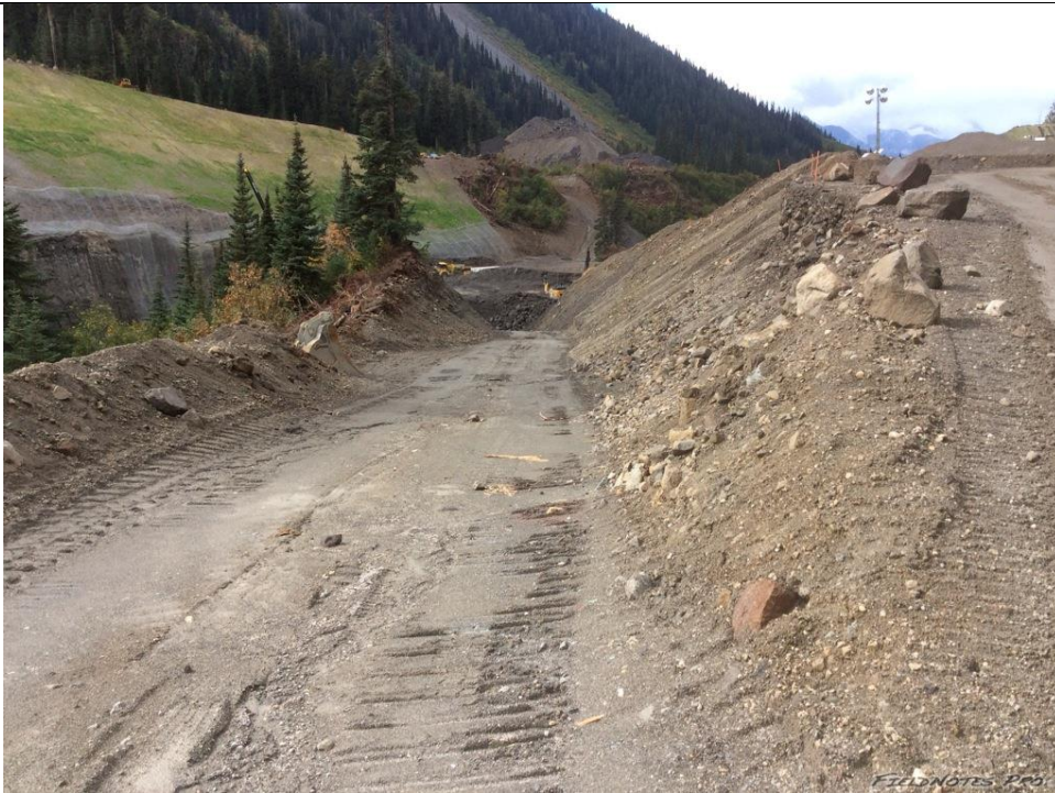
Photo 1. South side access road surface runoff causing erosion must be mitigated. Ditching and check dam installation is recommended.
