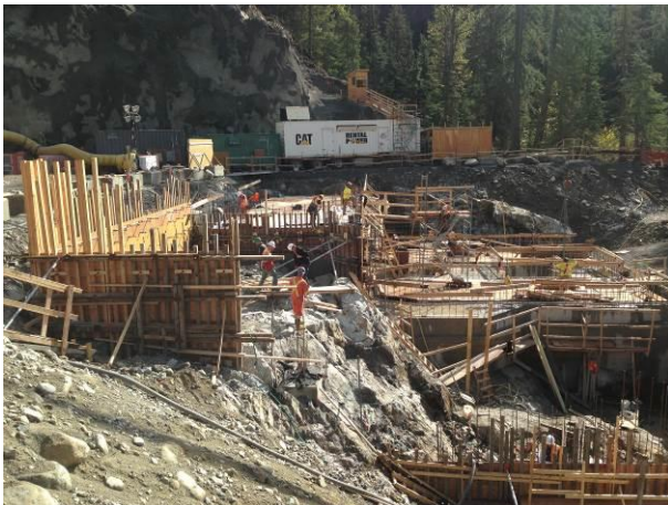
Photo 13 – BDRHEF downstream tunnel portal and powerhouse rebar/formworks (September 27, 2014).
