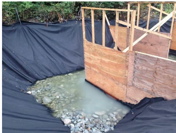
Photo 8 – The second ULRHEF settling pond, no discharge observed (September 26, 2014).
