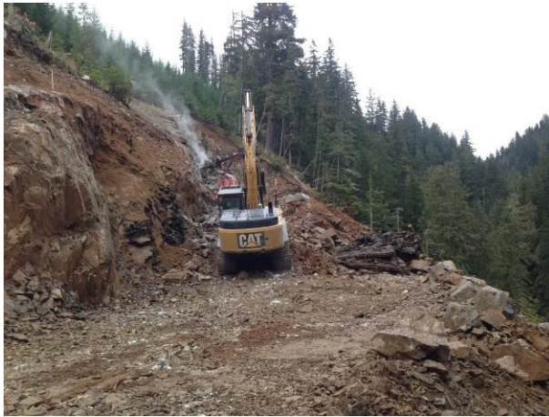
Photo 11 – BDRHEF crane pad excavation at upper pad (September 26, 2014).
