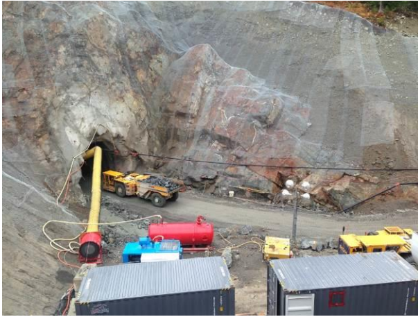
Photo 6 – ULRHEF downstream tunnel portal (September 16, 2014).
