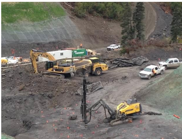
Photo 2 – ULRHEF north side tunnel portal excavation below elevation 666m (September 26, 2014).
