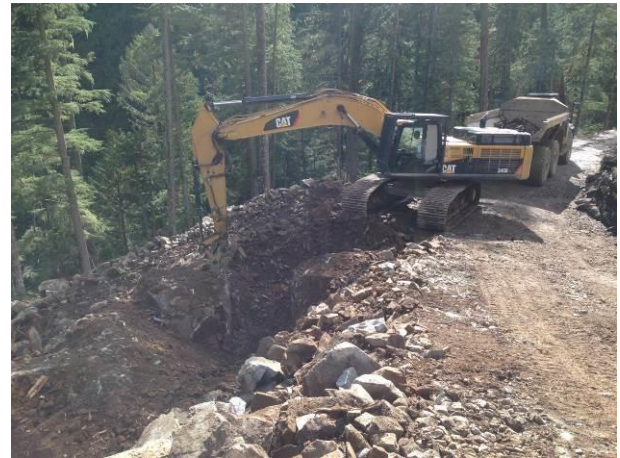
Photo 12 – BDRHEF Intake access road construction at ~4.2km (September 27, 2014).
