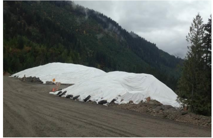
Photo 7 – Temporary PAG stockpiles located near the ULRHEF downstream tunnel portal remained covered with impermeable plastic tarps (September 26, 2014).
