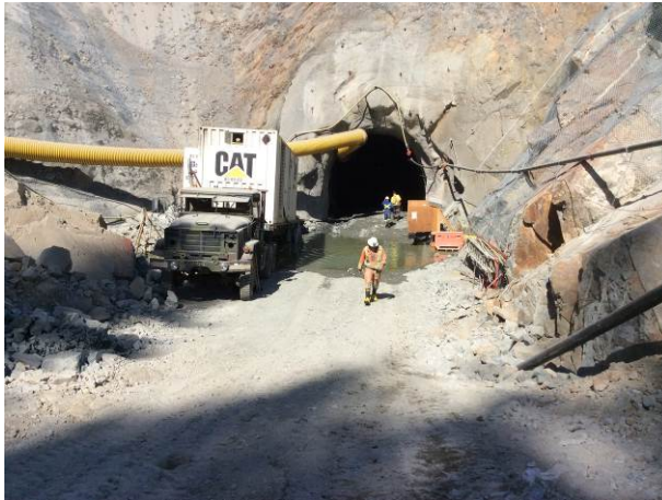
Photo 5 – ULRHEF downstream tunnel portal (September 16, 2014).
