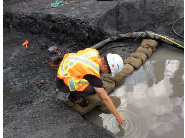
Photo 4 – Measuring pH in isolated section of Obermeyer weir excavation. This water was treated with a CO 2 and confirmed to be below pH 9 prior to reaching the pump (September 19, 2104).
