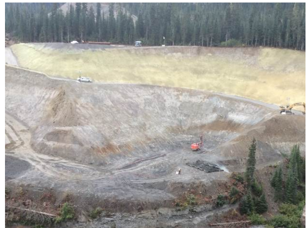
Photo 2 – ULRHEF north side tunnel portal excavation below elevation 666m (September 18, 2014).
