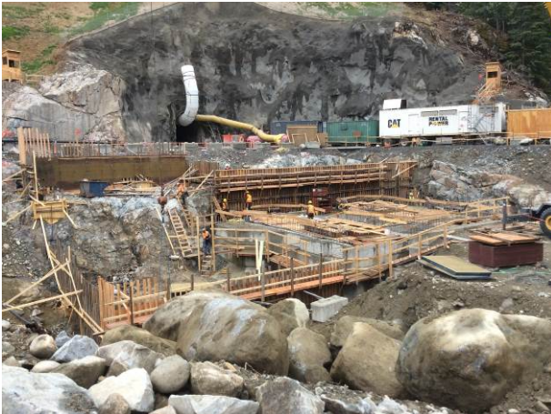
Photo 13 – BDRHEF downstream tunnel portal and powerhouse rebar/formworks (September 18, 2014).
