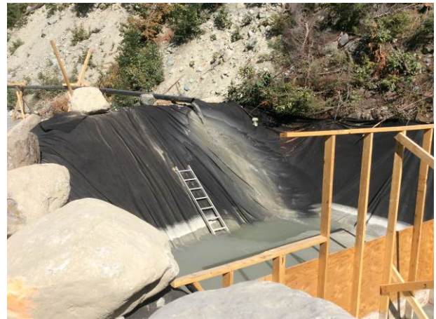
Photo 8 – Inlet of the ULRHEF settling ponds, no discharge observed (September 16, 2014).
