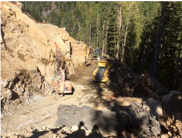
Photo 11 – BDRHEF Intake access road construction (September 16, 2014).
