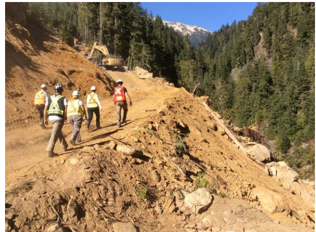
Photo 12 – BDRHEF crane pad excavation at upper pad (September 16, 2014).
