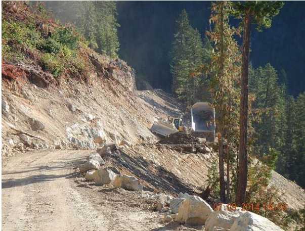
Photo 22 – BDRHEF Intake access road construction (September 7, 2014)
