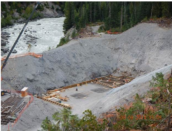
Photo 11 – ULRHEF powerhouse rebar and formworks (September 8, 2014).
