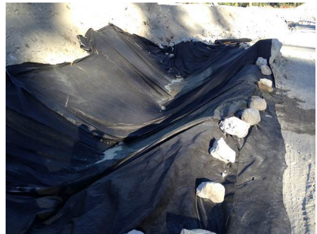
Photo 14 – Concrete washout pit along access road to ULRHEF powerhouse (September 10, 2014)
