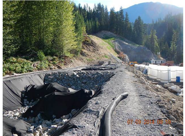
Photo 25 – BDRHEF powerhouse settling pond, no discharge observed (September 7, 2014)
