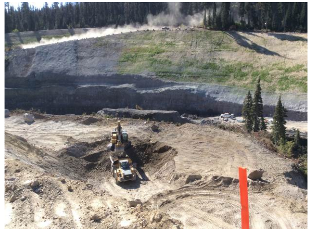
Photo 4 – Continued bulk excavation at ULRHEF north side open cut (September 12, 2014).
