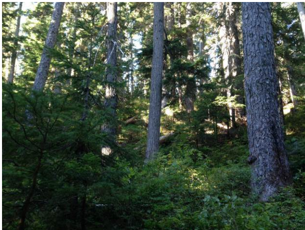
Photo 26 – Segment 14, hand falling within 100m CTF buffer near structure 340 (September 1, 2014).
