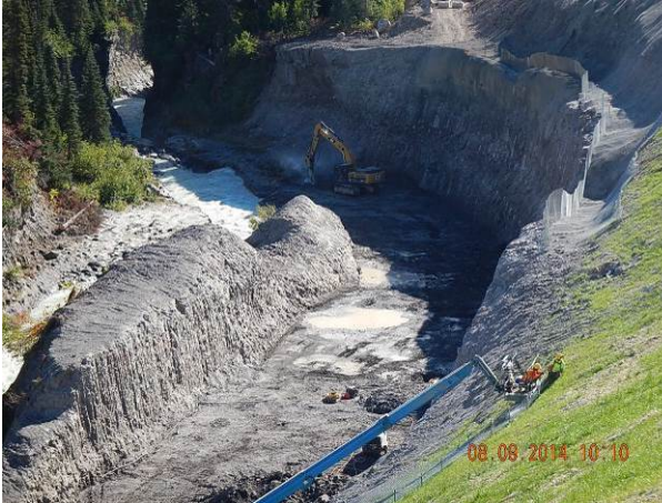
Photo 1 – Continued excavation of ULRHEF intake diversion channel, river levels dropped (September 9, 2014).
