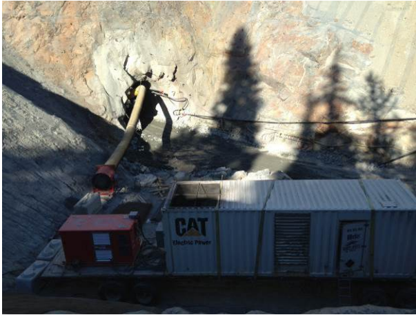
Photo 7 – ULRHEF downstream tunnel portal (September 9, 2014).
