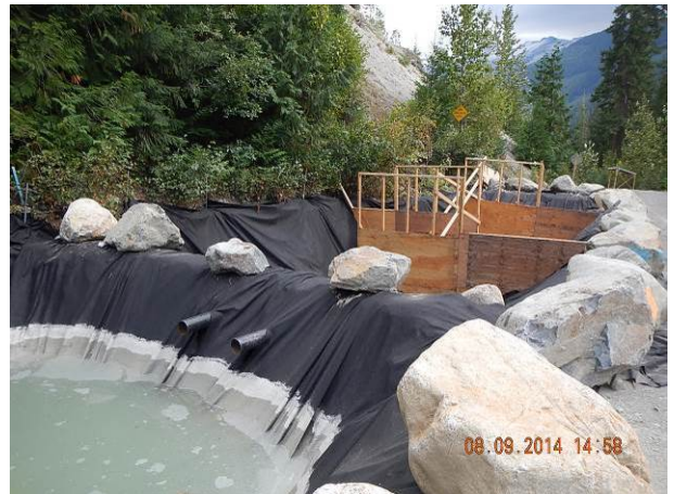
Photo 10 – ULRHEF settling ponds, no discharge observed (September 8, 2014).
