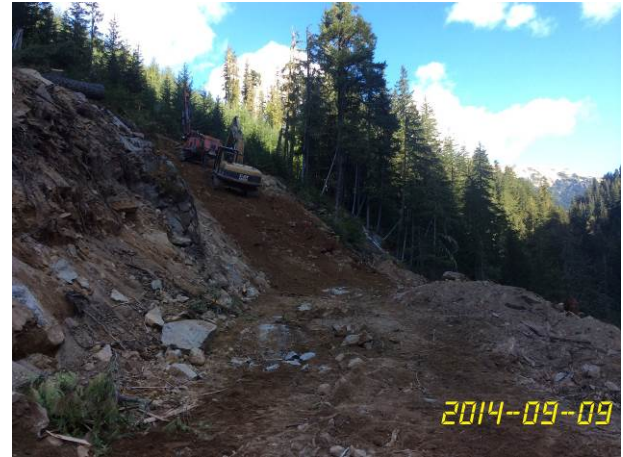
Photo 23 – BDRHEF crane pad drilling and excavation at upper bench (September 9, 2014)
