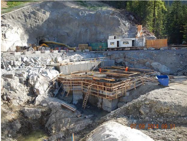
Photo 24 – BDRHEF downstream tunnel portal and powerhouse rebar/formworks (September 7, 2014)
