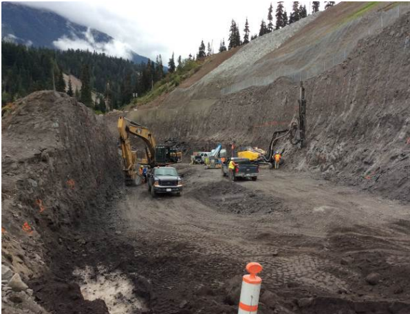
Photo 1 – Drilling and blasting at ULRHEF intake diversion channel (September 1, 2014).
