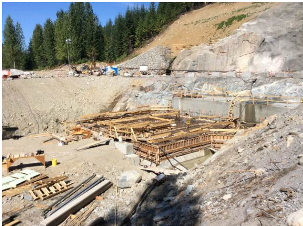
Photo 10 – Continued formworks at BDRHEF powerhouse (September 4, 2014)
