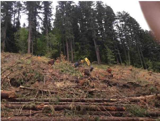
Photo 12 – Segment 5 machine works (spider hoe) at structure locations (August 31, 2014).
