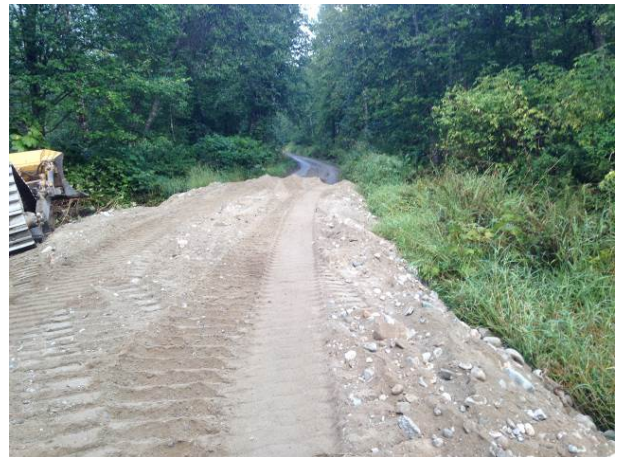
Photo 13 – Lillooet South FSR road ballasting near KM 7 (September 3, 2014).
