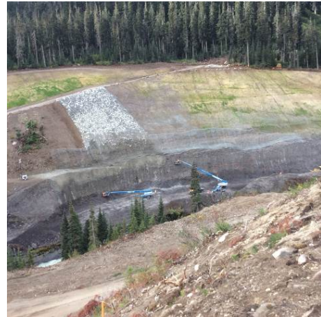
Photo 2 – ULRHEF intake diversion channel, vertical slope anchoring (August 31, 2014)
