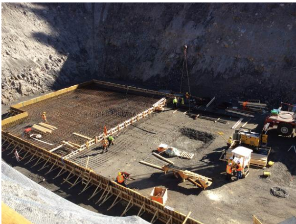
Photo 6 – ULRHEF powerhouse rebar installation and formworks (September 4, 2014)
