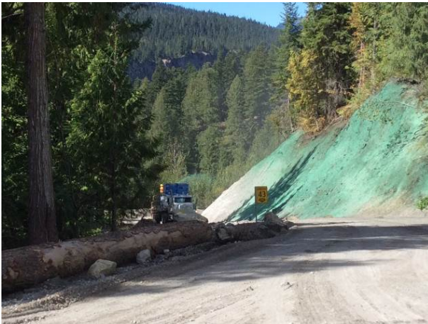
Photo 7 – Hydroseeding near KM 43 on Lillooet River FSR (September 3, 2014)
