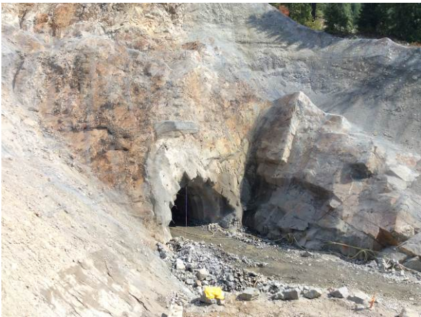
Photo 7 – ULRHEF downstream tunnel portal (August 24 th , 2014)
