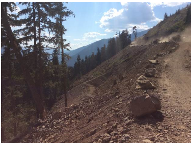
Photo 3 – BDRHEF Intake access road construction with OLTC protection berm (August 24 th , 2014)
