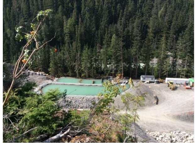
Photo 6 – Settling ponds at ULRHEF powerhouse (August 24 th , 2014)
