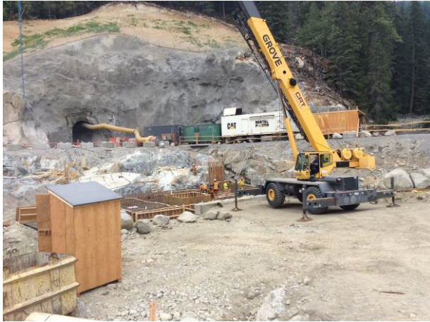
Photo 1 – Formworks at powerhouse and tunnel portal (August 25 th , 2014)
