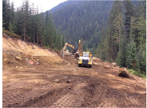
Photo 2 – Intake access road construction and ditching (August 25 th , 2014)
