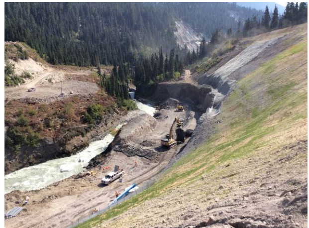
Photo 8 – ULRHEF intake diversion channel, north side (August 24 th , 2014)
