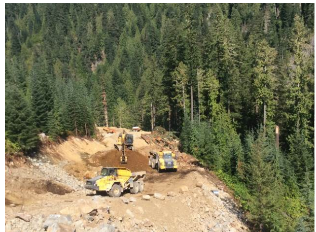
Photo 4 – BDRHEF crane pad construction (August 24 th , 2014)
