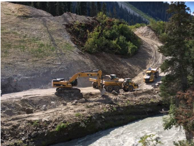
Photo 3. ULRHEF intake diversion channel excavation adjacent to the Lillooet River. (August 21, 2014).
