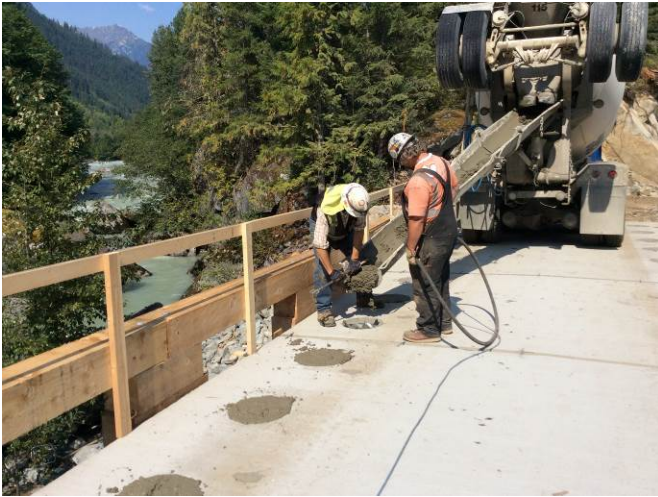
Photo 5. Grouting of Ryan River bridge deck panels (August 22, 2014).
