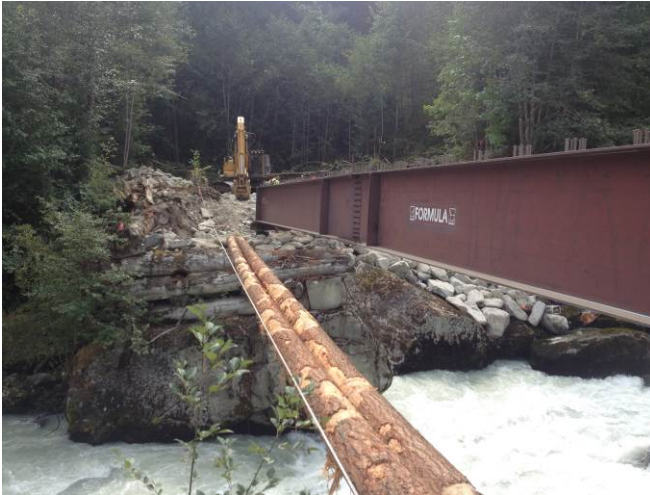
Photo 8. Ryan River Bridge girders (August 16, 2014).
