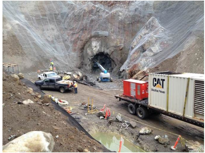
Photo 4. Tunnel stabilization activities at the ULR downstream portal. (August 15, 2014).
