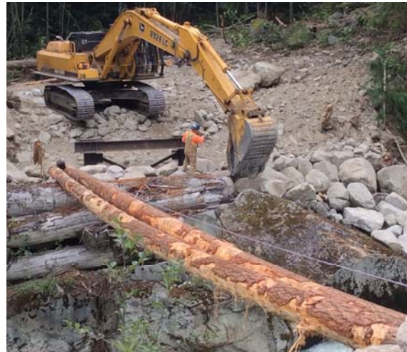
Photo 6. Riprap placement adjacent to the Ryan River (August 14, 2014).
