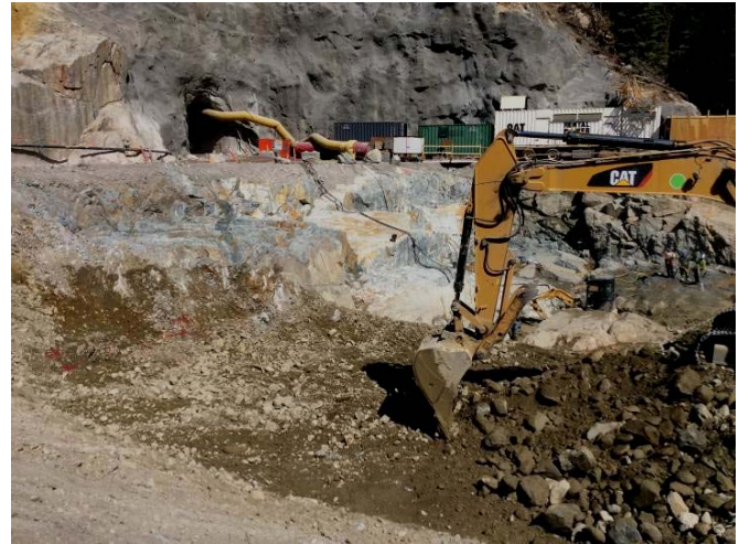
Photo 2. Dewatering of seepage from within the powerhouse excavation was pumped to the sediment ponds. Water has not yet reached the second treatment pond (August 9, 2014).
