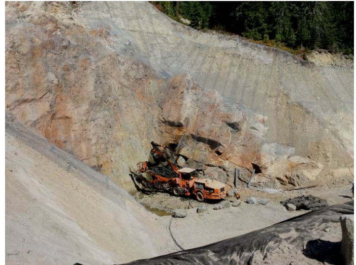
Photo 4. Drilling activities at the ULR downstream portal. (August 6, 2014).
