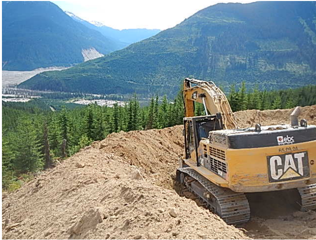
Photo 1. Stripping and grubbing of the BDR-3 spoil area (August 1, 2014).
