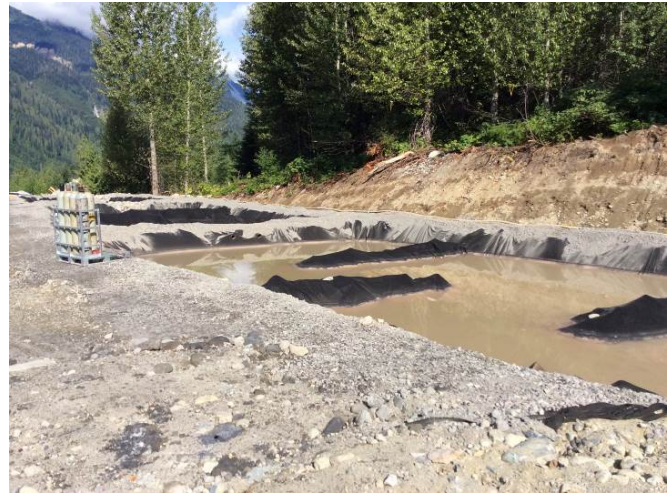
Photo 2. Dewatering of seepage from the tunneling activities was performed this week but the water has not yet reached the second treatment pond (July 19, 2014).
