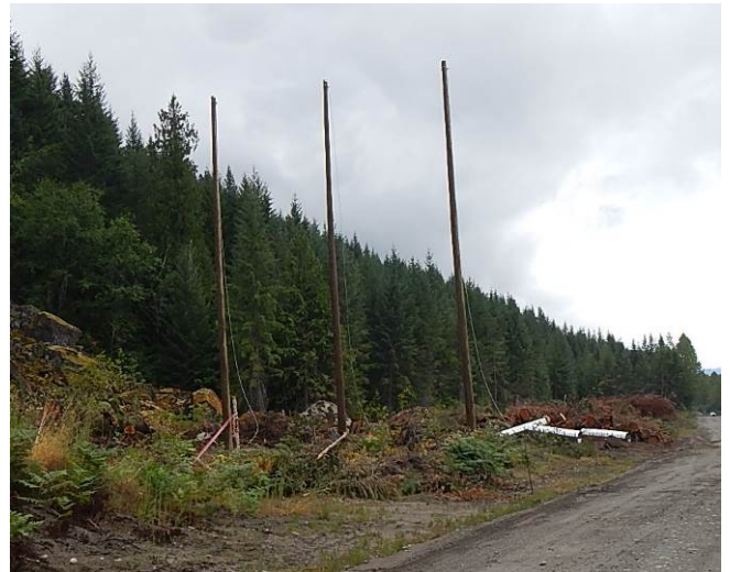
Photo 6. Poles installation underway in Segment 4 (July 19, 2014).
