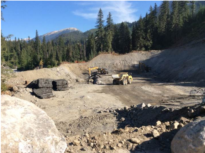
Photo 3. Excavation of the ULRHEF powerhouse footprint (July 15, 2014).
