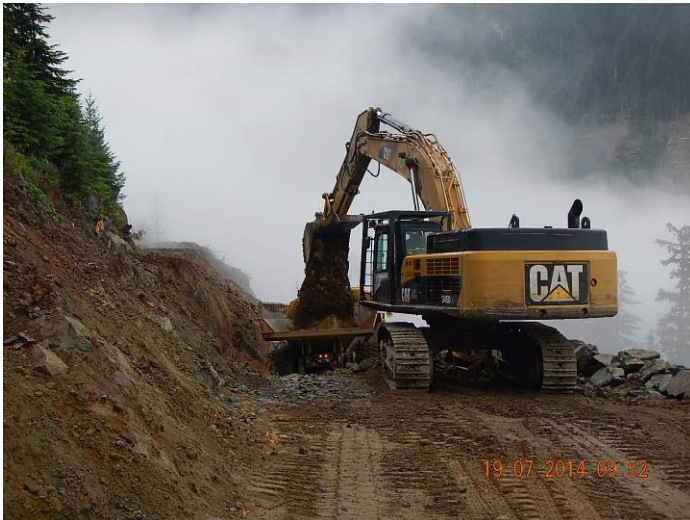
Photo 1. Construction of the BDR intake access road. (July 19, 2014).
