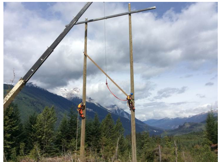
Photo 6. Pole dressing work in Segment 2 (July 4, 2014).
