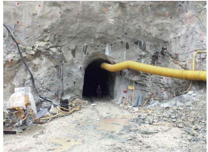
Photo 2. Tunneling works at the tunnel portal entrance. (July 4, 2014).
