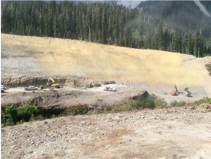
Photo 3. Excavation activities and hydro-seeding that has not successfully germinated at the ULRHEF intake diversion (July 4, 2014).
