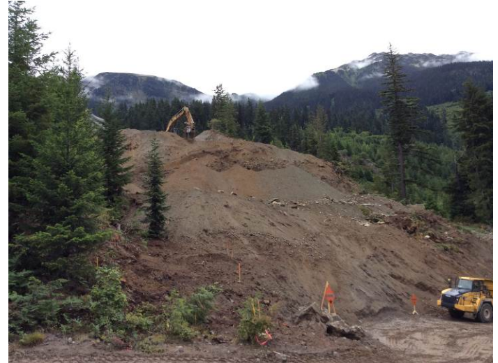
Photo 4. Excavation of the ULRHEF downstream portal (July 5, 2014).
