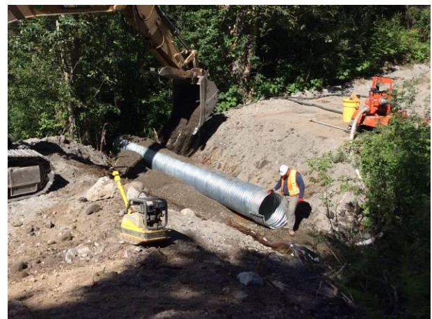
Photo 4. Culvert installation works at the Truckwash Creek east heading (June 25, 2014).
