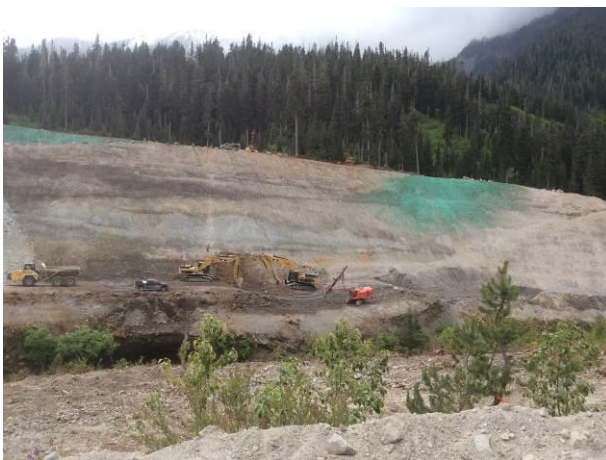
Photo 3. Excavation activities and hydro-seeding works at the ULRHEF intake diversion (June 27, 2014).
