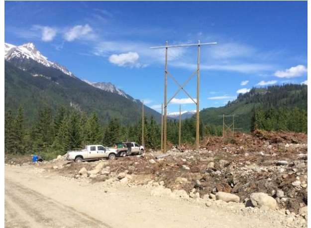
Photo 6. Pole installation work in Segment 1 (June 26, 2014).
