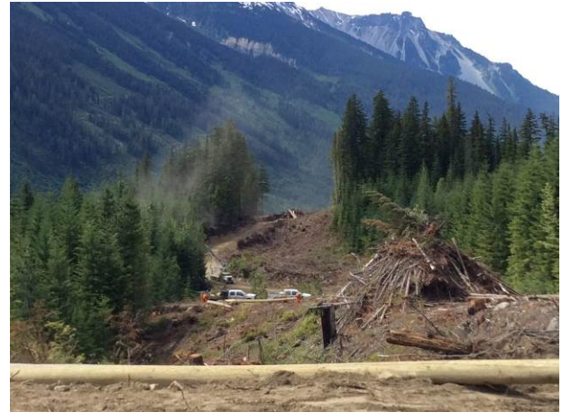
Photo 8. Pole installation work in Segment 2 (June 21, 2014).
