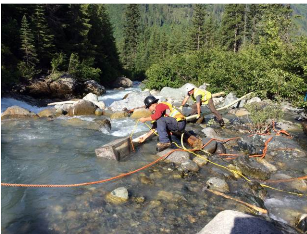
Photo 3. Installing the gravity-fed water diversion in Boulder Creek (June 21, 2014).
