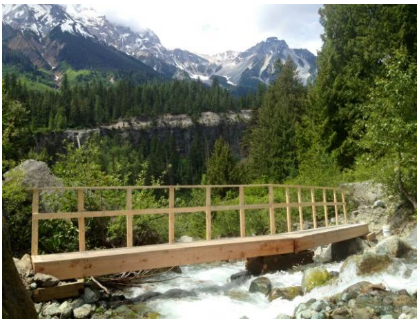
Photo 1. Temporary Truckwash Creek crossing (June 19, 2014).
