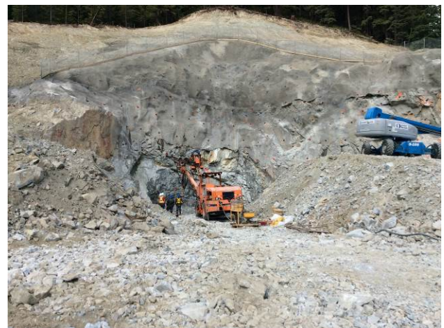
Photo 4. Stabilization works at the tunnel portal. (June 21, 2014).
