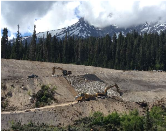
Photo 5. Slope protection installed at the right bank diversion excavation (June 18, 2014).
