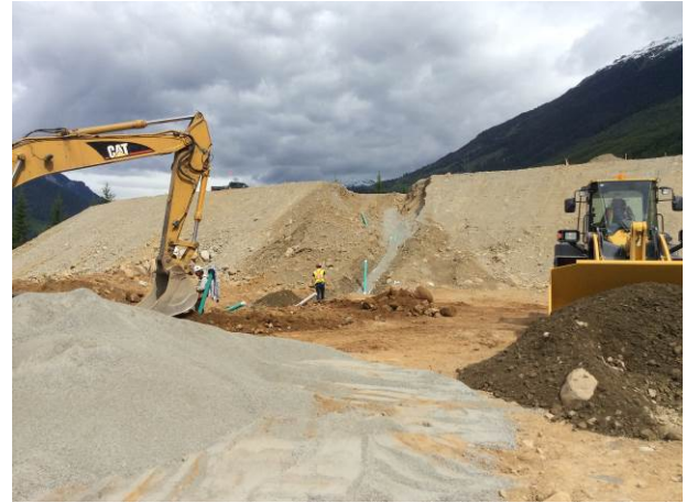
Photo 2. Utility installation at the construction camp. (June 8, 2014).
