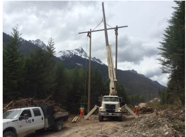
Photo 7. Pole installation work in Segment 1 (June 11, 2014).
