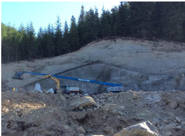
Photo 1. Shotcrete and rock bolt installation at the
