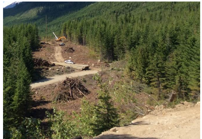
Photo 7. Pole installation work in Segment 2 (June 4, 2014).
