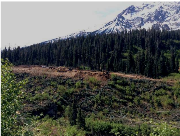
Photo 4. Conditions at the right bank diversion channel excavation on June 7, 2014.
