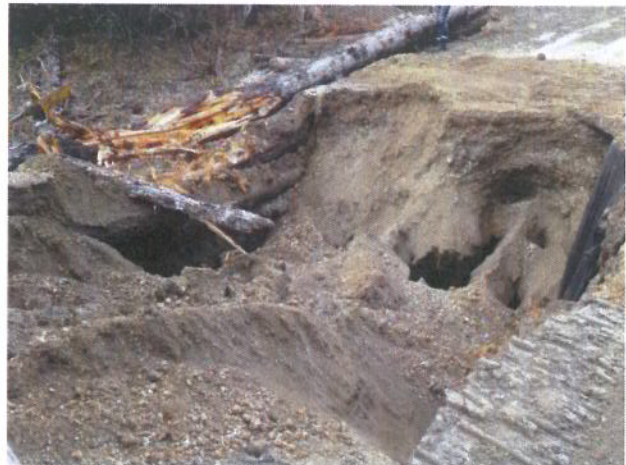
Photo 2: Box culvert post-excavator removal.
