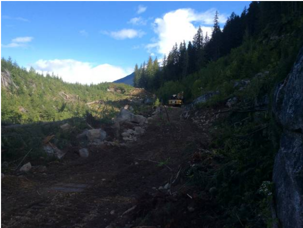
Photo 6. Access road construction; Pebble D.1 Branch road (May 28, 2014).
