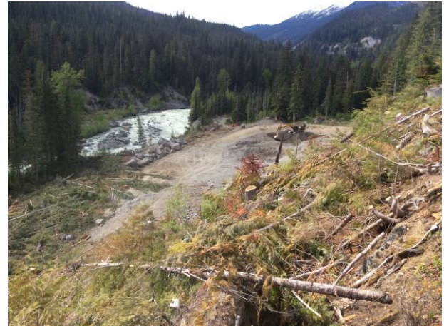
Photo 5. Bench excavation at the ULRHEF powerhouse. (May 27, 2014).
