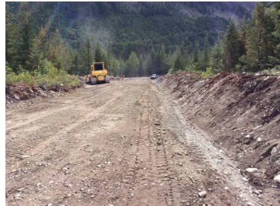
Photo 2. Grade changes along Boulder Creek powerhouse access road. (May 27, 2014).
