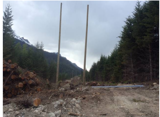
Photo 7. Pole installation work in Segment 1 (May 28, 2014).
