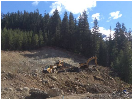
Photo 1. Excavation of the BDRHEF downstream portal location (May 28, 2014).
